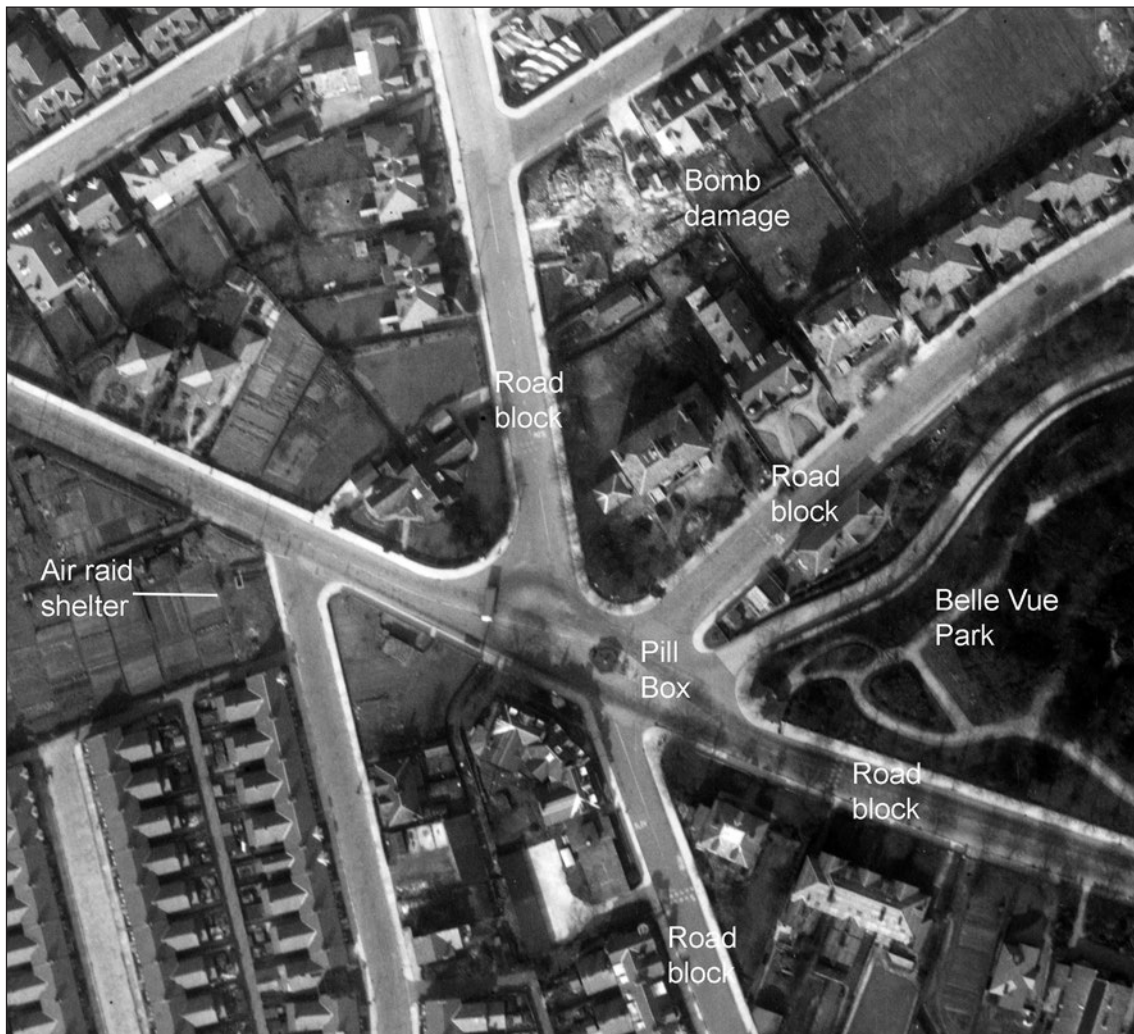
Figure 54 – The north-west of Bellevue Park showing a pill box controlling the junction and road blocks (seen as parallel rows of white dots), an air raid shelter in allotments (left), and some bomb damage on the corner of Lyndhurst and Corton roads; note the camouflaged buildings across the road (mid-top frame) (RAFHLA/698 3020 08-APR-1944 Historic England (RAF Photography))
