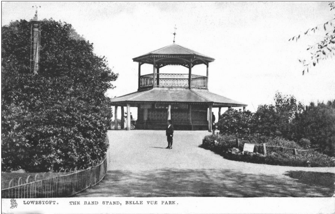
Figure 11 – A postcard, posted in 1904, showing the pagoda with deep ground floor veranda and open viewing platform above. Note the anemometer of the weather station which can be seen projecting above the shrubs to the left. (© Historic England)
