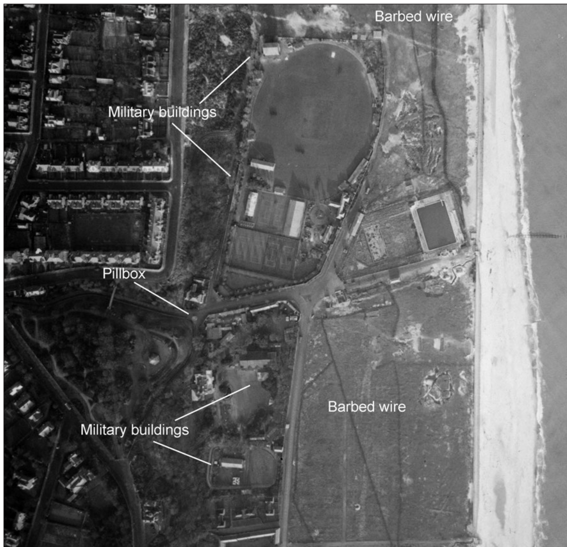
Figure 45 – An aerial view of military buildings associated with Sparrow’s Nest and the developing beach defences in December 1941; barbed wire entanglements on the Denes show up as broad dark lines (Detail from RAF-2H-BR165 V 15 24-DEC-1941, Historic England (RAF Photography))
