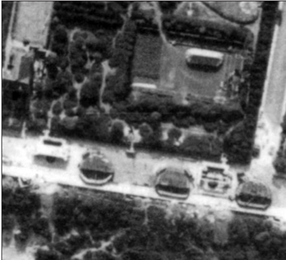
Figure 48 – Detail of Figure 47 showing the three temporary gun emplacements and other structures on Gunton Esplanade with the new emplacements under construction between them, north is to the right (RAF/2/BR11/16 VA A12 19-JUL-1940 Historic England (RAF Photography))
