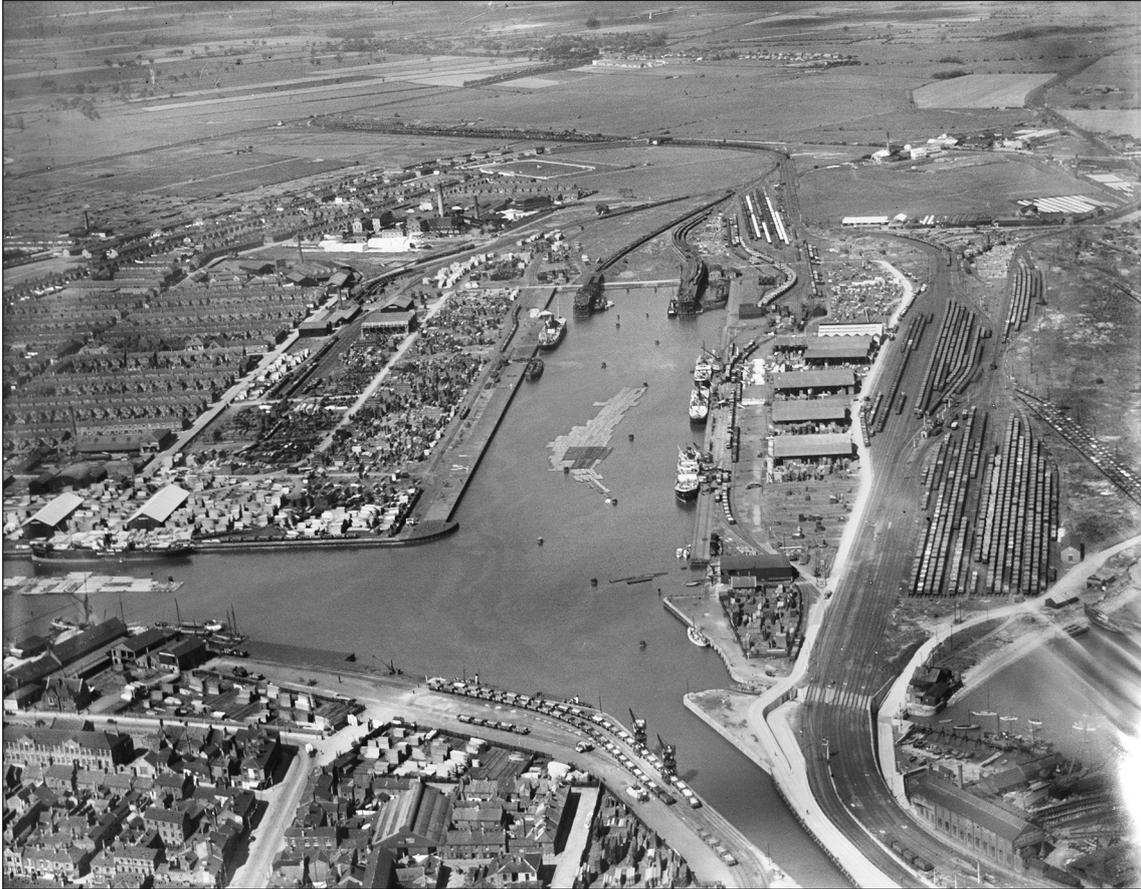
Fig 9: A view of Alexandra Dock looking westwards. The two coal drops can be seen at the western end of the dock along with extensive railway sidings to the north. © Historic England Archive. Aerofilms Collection EPW053388 31-MAY-1937.
