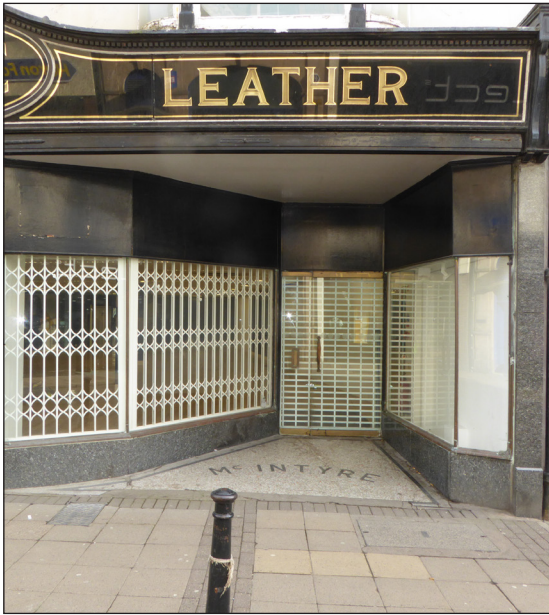
Figure 19: Detail of south shopfront and recessed doorway (© Historic England, photograph: Alastair Coey Architects 2019)
