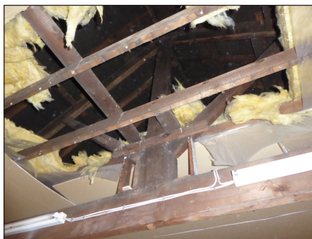
Figure 27: (b) Detail of roof structure (© Historic England, photograph: Alastair Coey Architects 2019)
