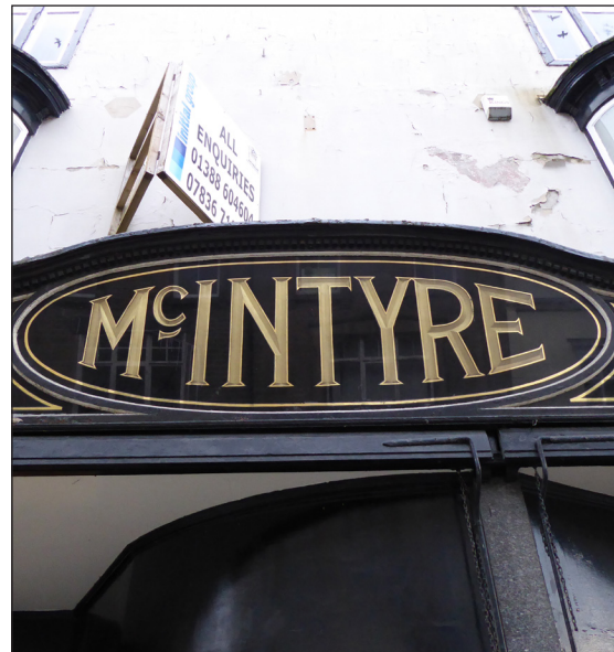
Figure 18: Detail of central fascia signage (© Historic England, photograph: Alastair Coey Architects 2019)
