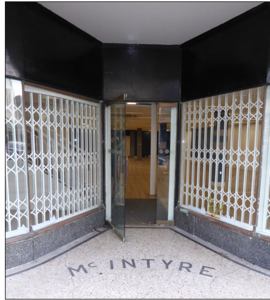
Figure 20: Detail of recessed doorway to north showing mosaic flooring (© Historic England, photograph: Alastair Coey Architects 2019)
