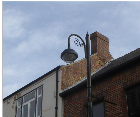
Figure 14: The south gable of the premises showing the English Garden Wall brick bond (© Historic England, photograph: Alastair Coey Architects 2019)
