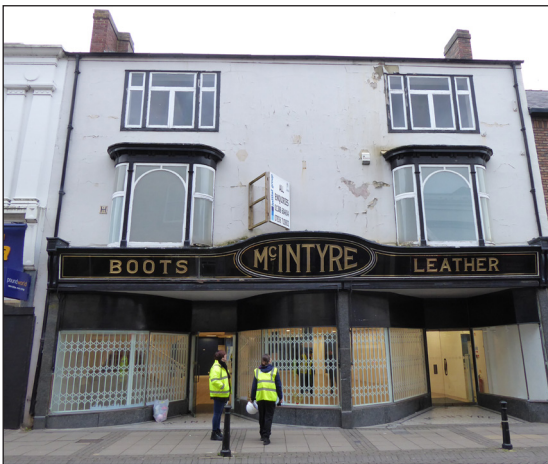
Figure 10: 25 Newgate Street in 2019 (© Historic England, photograph: Alastair Coey Architects 2019)
