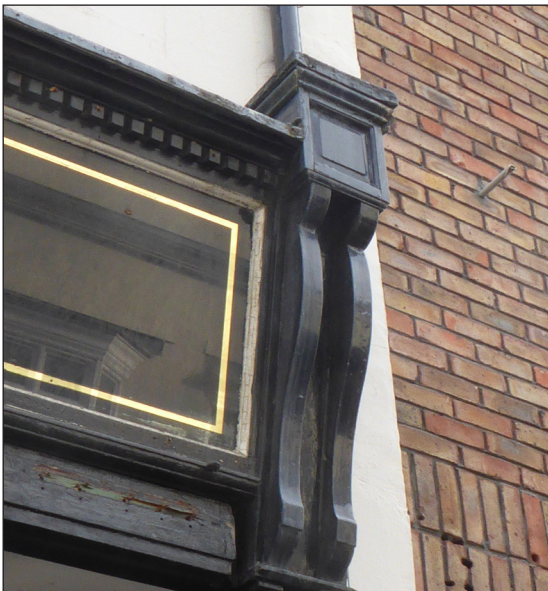
Figure 17: (b) Detail of console bracket (© Historic England, photograph: Alastair Coey Architects 2019)
