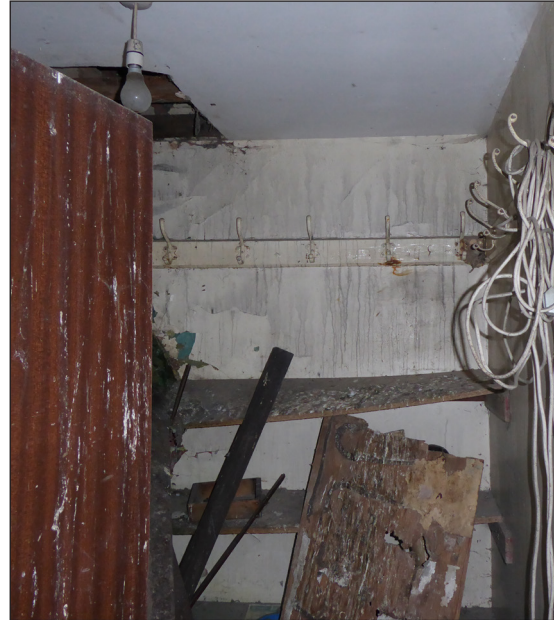
Figure 59: Detail of coat racks and hangers in second-floor cloak room (© Historic England, photograph: Alastair Coey Architects 2019)
