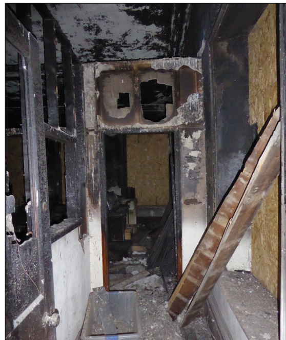
Figure 40: View of the first-floor glazed and timber lobby (© Historic England, photograph: Alastair Coey Architects 2019)
