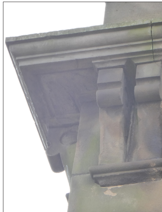
Figure 23: Detail of cornicing and eaves brackets of the Mechanics' Institute (© Historic England, photograph: Alastair Coey Architects 2019)
