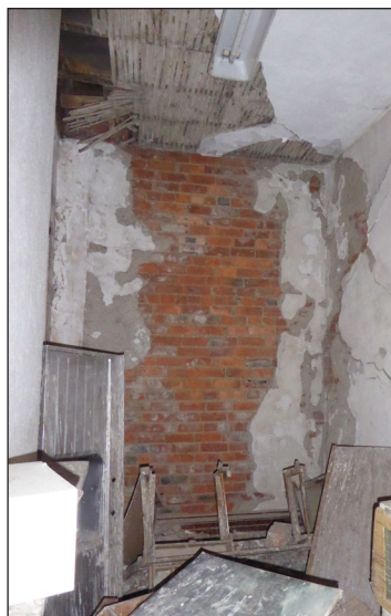
Figure 45: View of first-floor south-west room (© Historic England, photograph: Alastair Coey Architects 2019)
