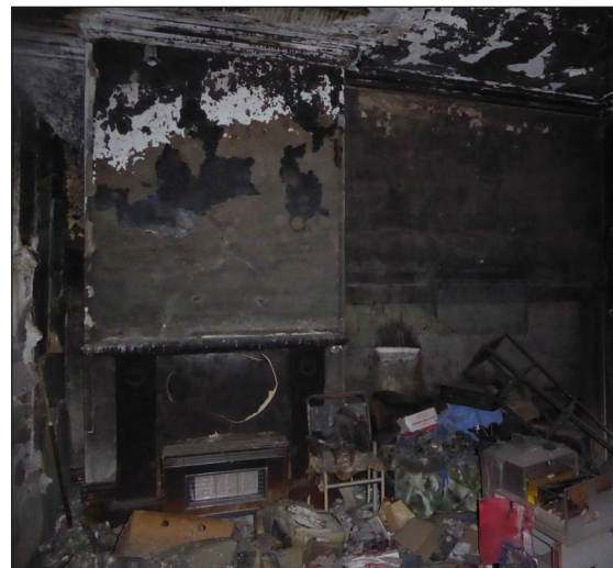
Figure 42: View of first-floor front room (© Historic England, photograph: Alastair Coey Architects 2019)
