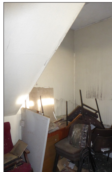
Figure 46: View of first-floor south-east room (© Historic England, photograph: Alastair Coey Architects 2019)
