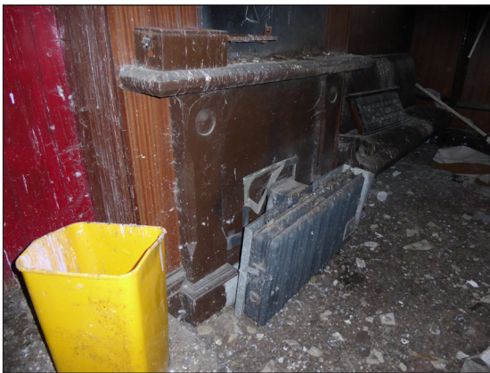
Figure 55: Detail of billiard room fireplace (© Historic England, photograph: Alastair Coey Architects 2019)
