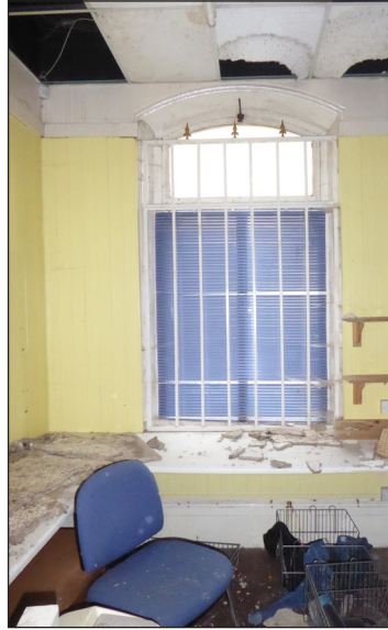
Figure 35: Internal detail of ground-floor window (© Historic England, photograph: Alastair Coey Architects 2019)
