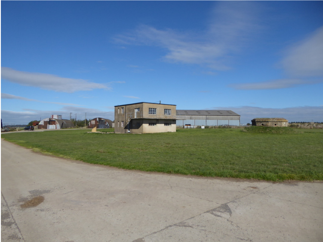
Figure 15: The control tower, pillbox and (to left) Romney huts form the core of a well-retained group of Second World War airfield buildings at former RAF Windrush. The control tower is open to visitors on an occasional basis. Pillboxes such as this are well-known as bat habitats. Note the hard-standing in the foreground. © Jeremy Lake.
