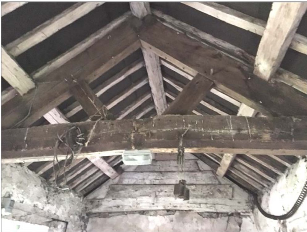
Figure 15: The Gatehouse, truss 2 in foreground, photograph taken from (Alison Arnold)
