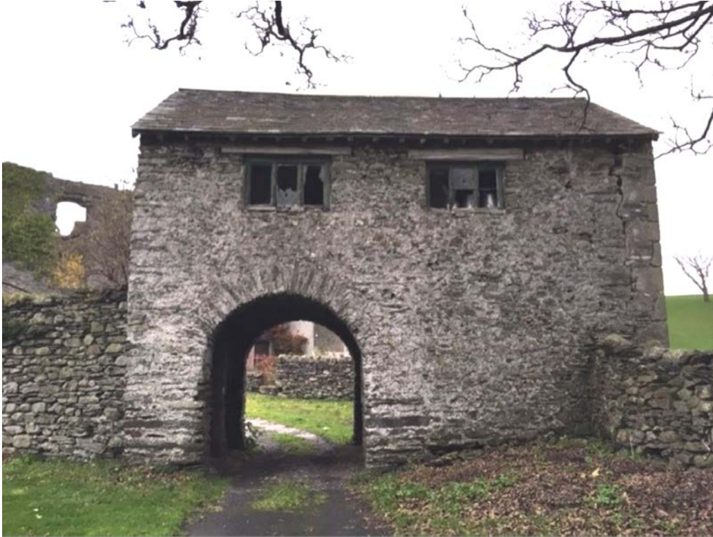
Figure 14: The Gatehouse, photograph taken from the north-east (Alison Arnold)
