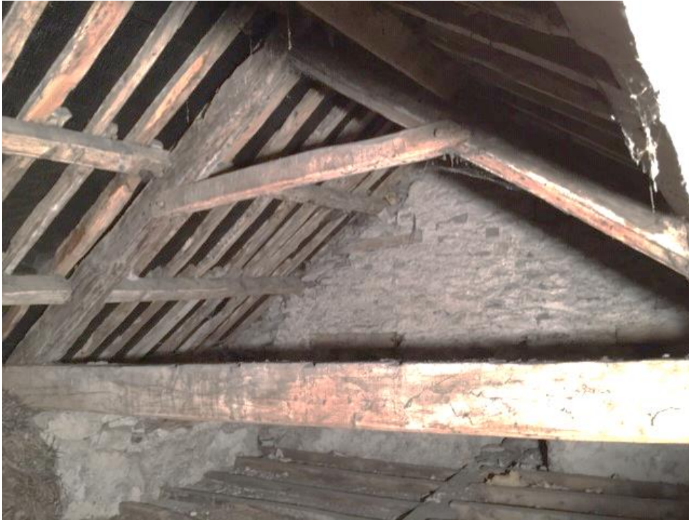
Figure 10: Cross-wing truss 5, photograph taken from the west (Alison Arnold)
