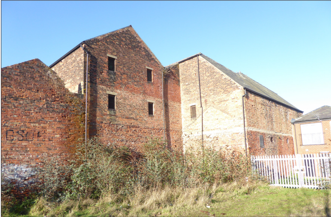
Figure 24: East elevation and north-east projection with variations in brickwork colour and evidence of the cast concrete first-floor slab (© Historic England, photograph: Alastair Coey Architects 2019)
