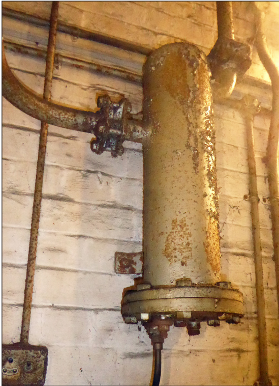
Figure 31: Oil separator (© Historic England, photograph: Alastair Coey Architects 2019)
