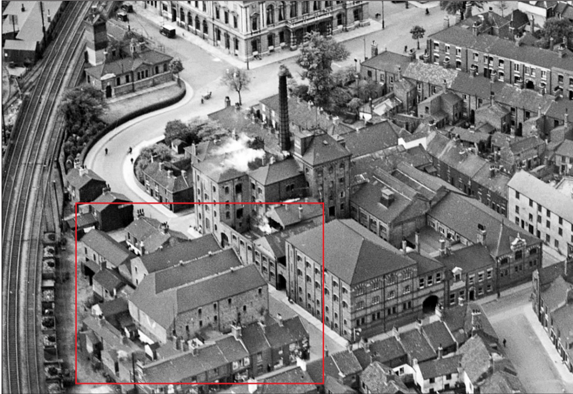
Figure 17: An aerial image of Hewitts Brewery in 1933 with the warehouse shown within the red square (© Historic England, Aerofilms Collection) Ref. EPW042807
