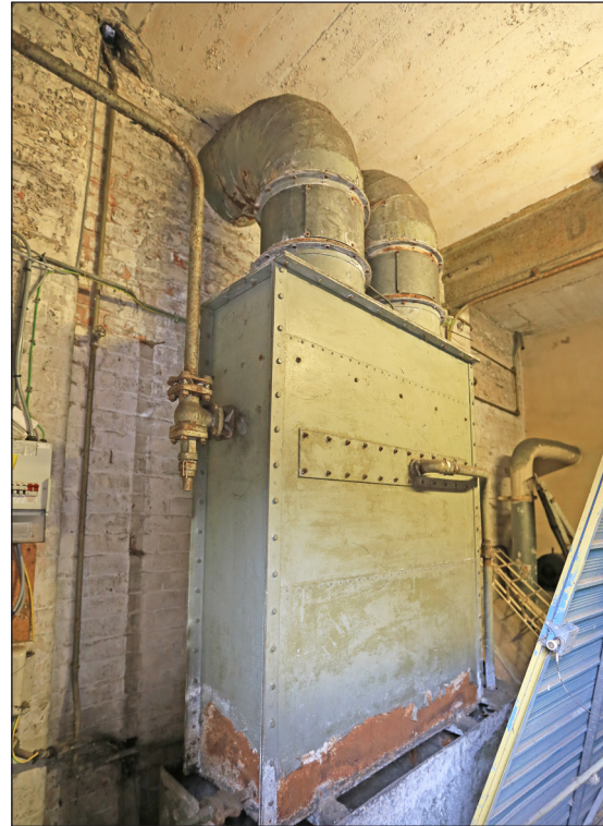
Figure 32: Condenser (© Historic England, photograph: Alastair Coey Architects 2019)
