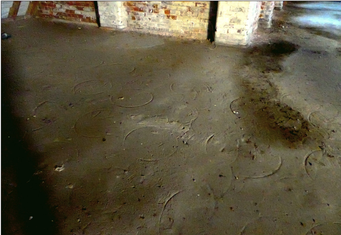
Figure 2: Cask imprints on the second floor of the warehouse (© Historic England, photograph: Alastair Coey Architects 2019)
