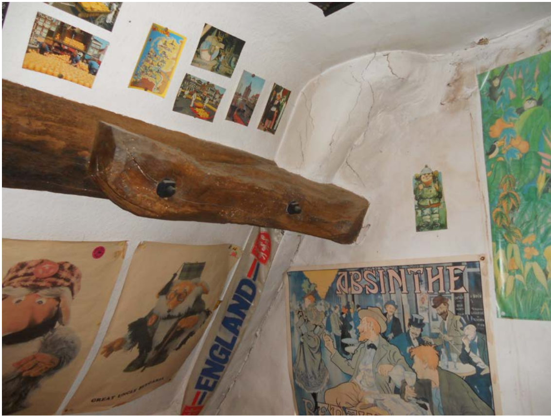
Figure 6: The attached 'knee' added to the west purlin in the north attic room (photograph Martin Bridge)
