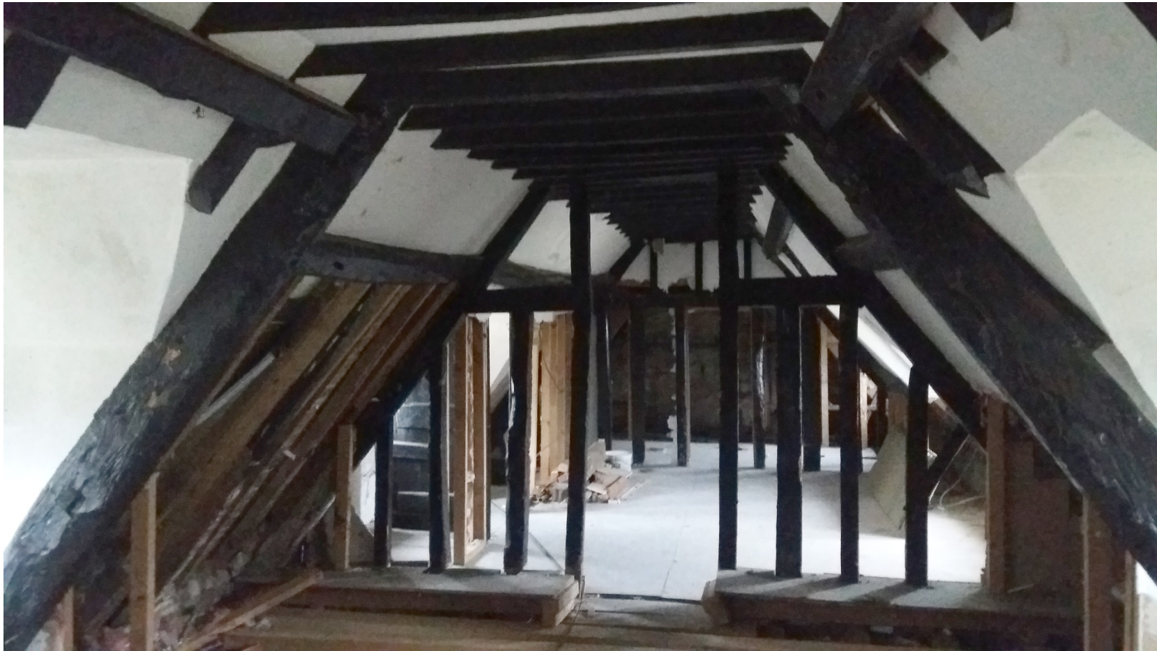
Figure 4: View of the attic facing south (photograph Martin Bridge)
