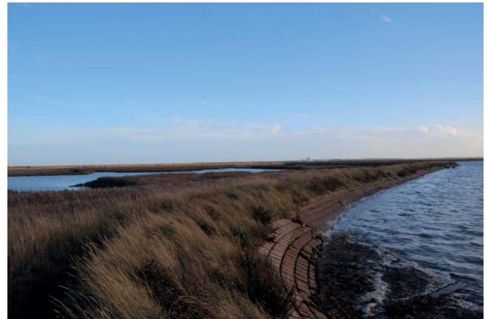
Figure 3 Sea-wall at Old Hall Marshes, Tollesbury
