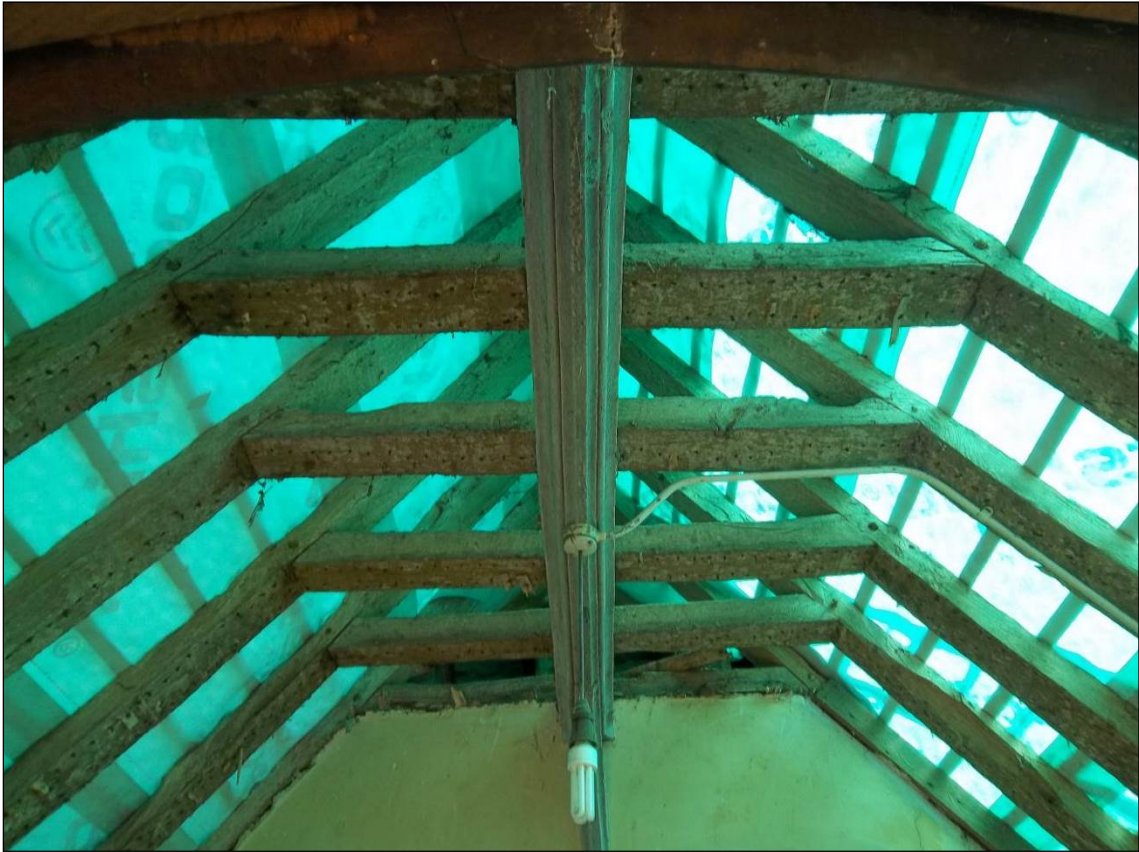
Figure 5: Porch roof (photograph taken from the south)
