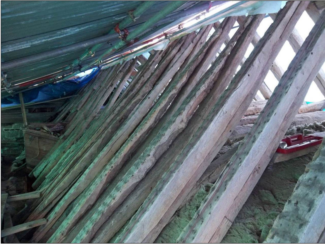
Figure 3: Nave roof showing the backing rafters (photograph taken from the south-east)
