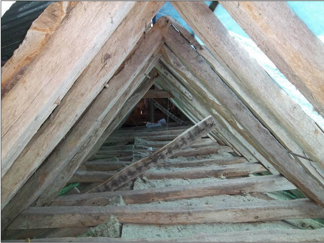
Figure 4: South aisle roof (photograph taken from the west)
