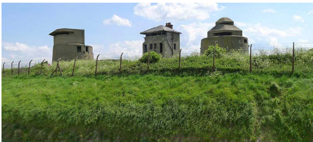
Image 19 Sheerness Centre Bastion (© W D Cocroft)
