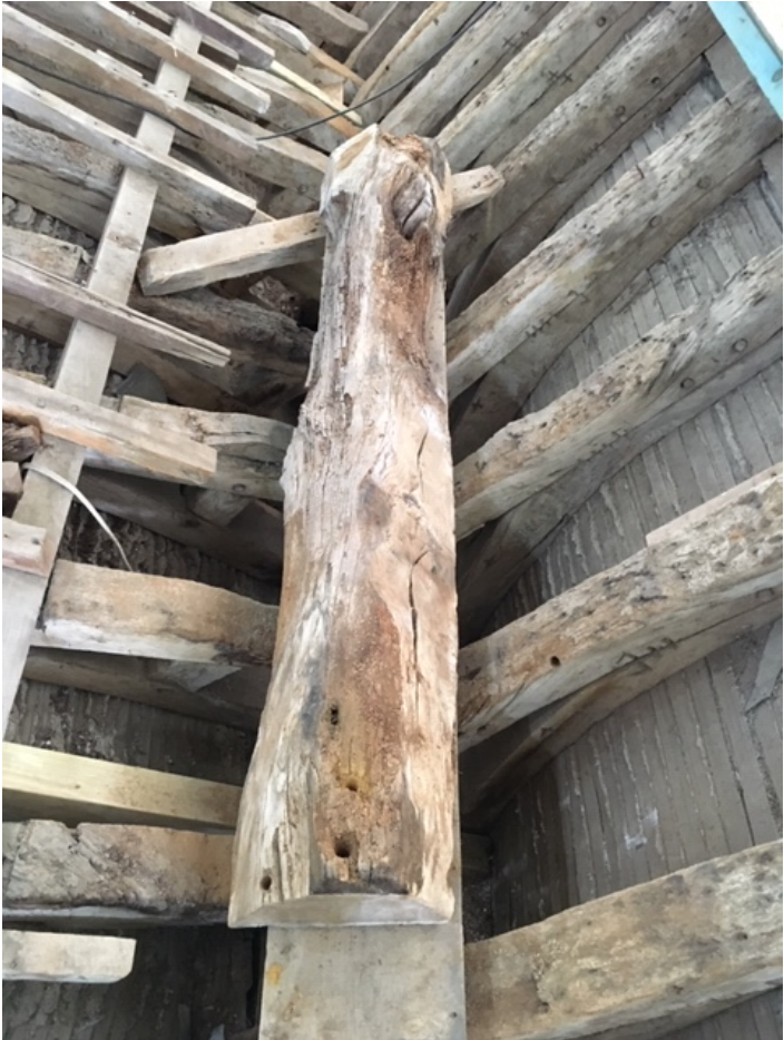
Figure 6: Valley gutter beams, beam 1 to the left and beam 2 to the right (Alison Arnold)
