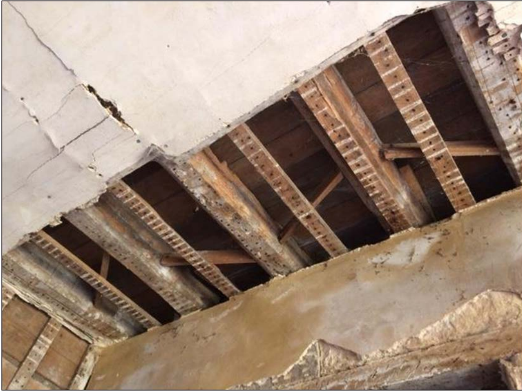
Figure 6: Portion of exposed floor frame from the annexe, photograph taken from the east (Alison Arnold)
