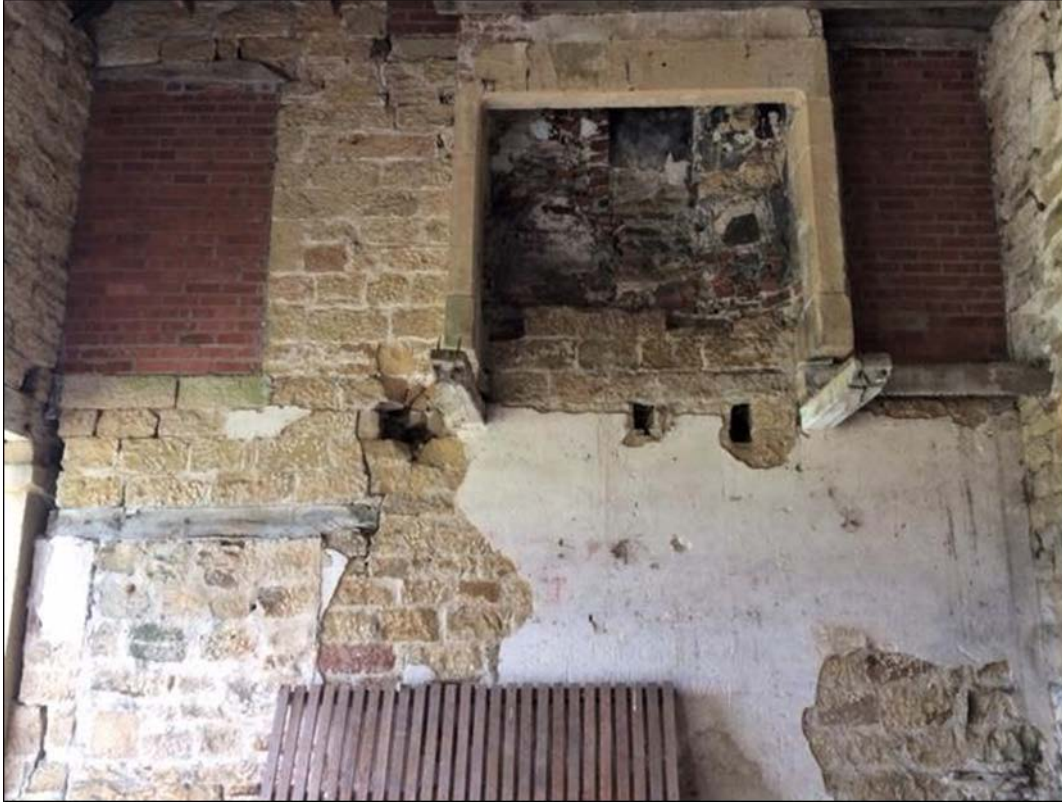
Figure 9: Surviving historic timbers; door lintel, supporting beams, and a floor beam, photograph taken from the north (Alison Arnold)
