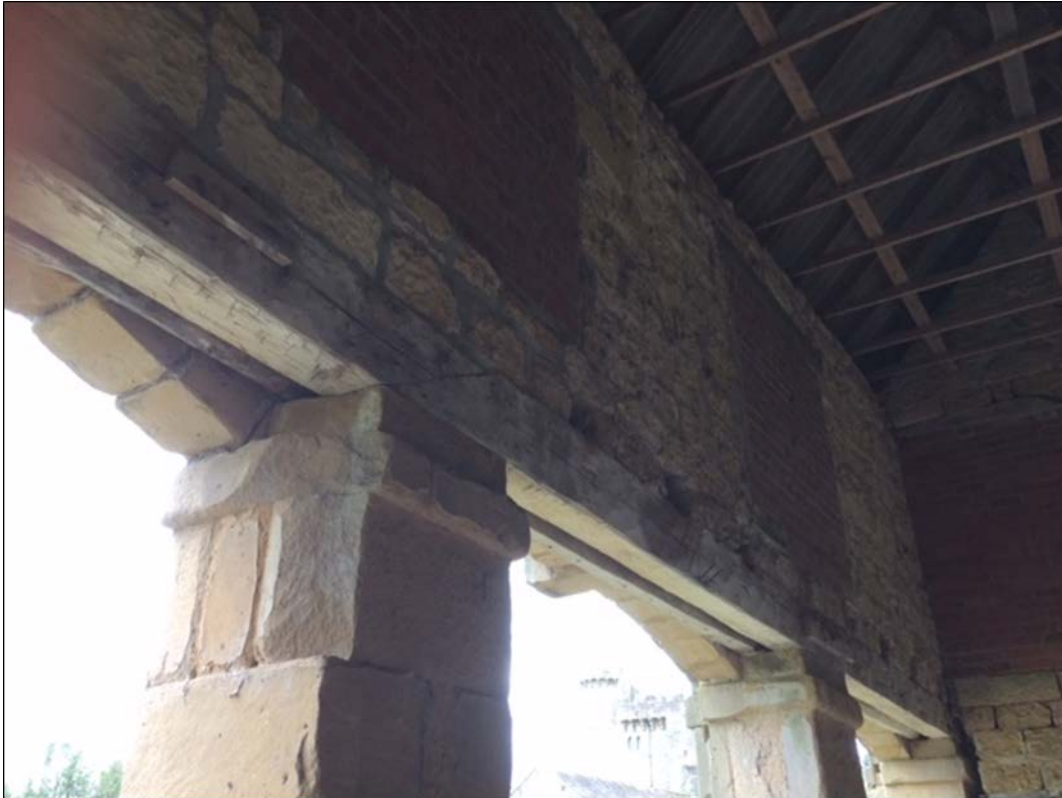
Figure 8: Lintels over the Coach house entrance, photograph taken from the east (Alison Arnold)
