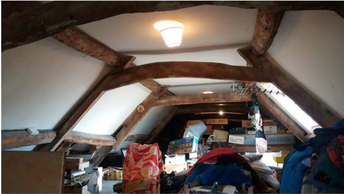
Figure 5: View of the roof to the main range of the manor, looking east, showing the general form of the trusses (photograph Martin Bridge)
