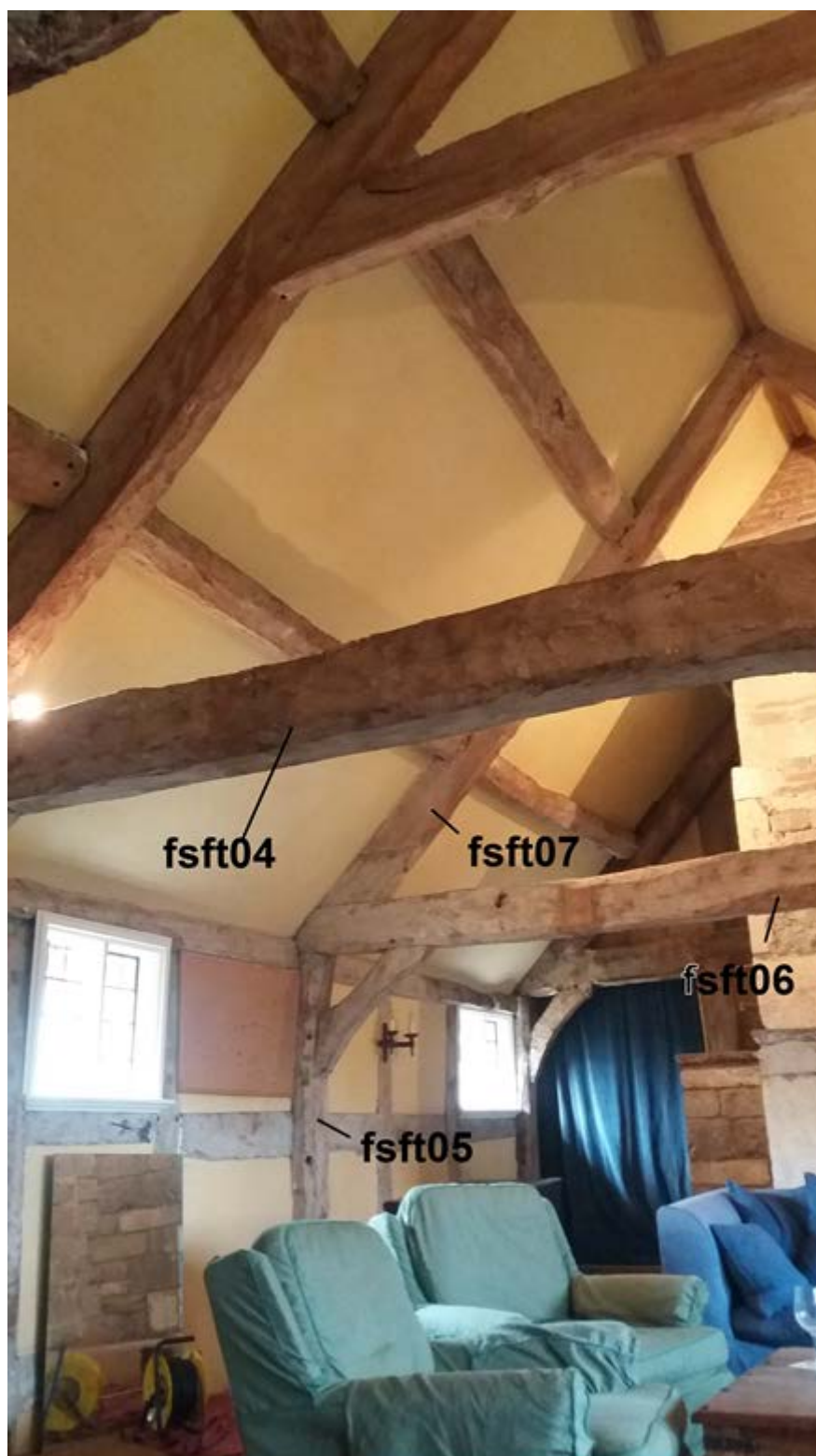
Figure 4: View within the flat, looking south-east, showing some of the timbers sampled (photograph Martin Bridge)
