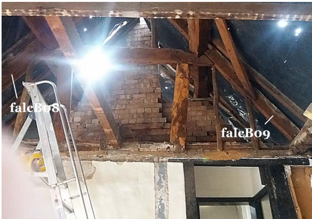
Figure 5: View looking east, showing truss 1, with some of the timbers sampled (photograph Martin Bridge)
