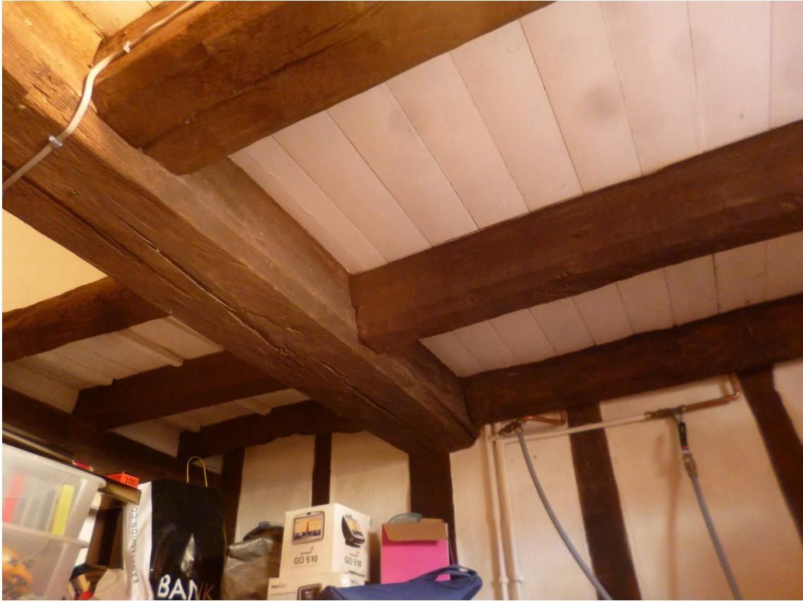
Figure 6: Stairwell at cellar level
