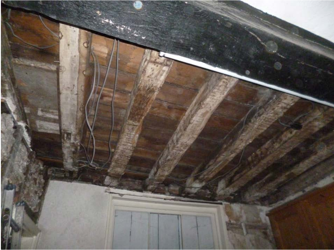
Figure 6: 19 Ladygate, exposed ceiling beams, photograph taken from the east (Alison Arnold)
