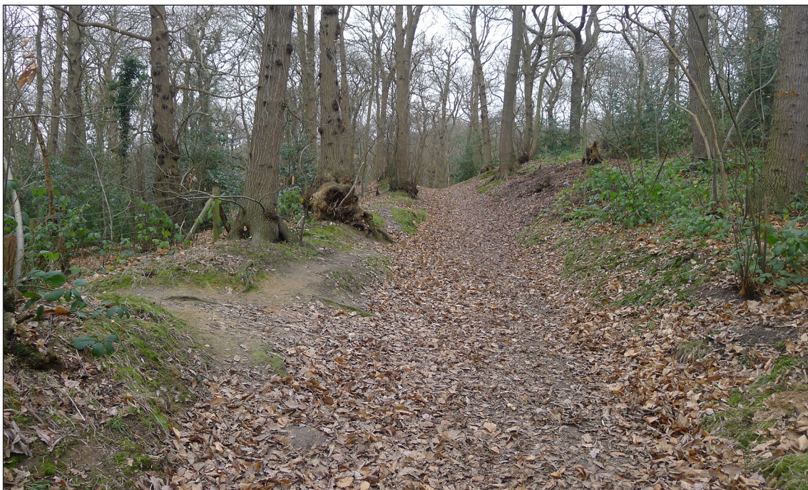
Figure 35: The view looking east along the stretch of bank and ditch boundary as it runs east from New Road ([D] on Fig 33). The bank is to the left (north) and the ditch is to the right (south) and contains the modern footpath. © Historic England (14-JAN-2019)..
