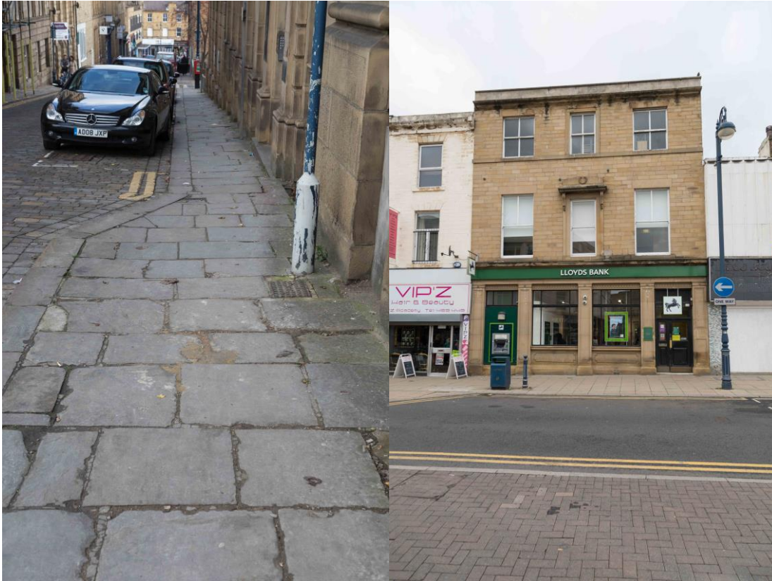
Figure 19: Surface treatments, from left: Bond Street, historic flag paving and restored sets to roadway; Market Place, mix of surfaces and street furniture
