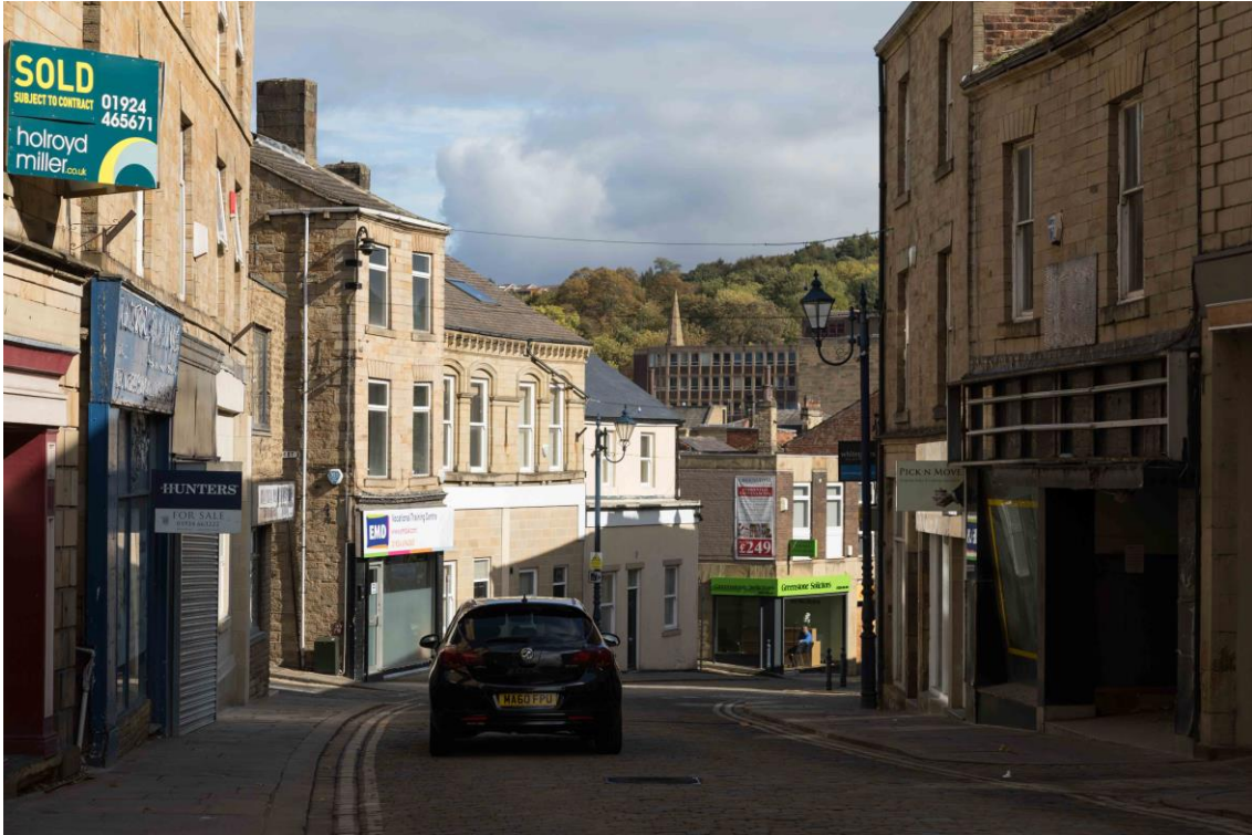
Figure 23: Incidental views along Daisy Hill from the west - human scale and tight, winding street contributes to the sense of time-depth; glimpses to landmarks (e.g. spire of Dewsbury Baptist Church, or the dome of the Town Hall) and the wider landscape help orientate the visitor
