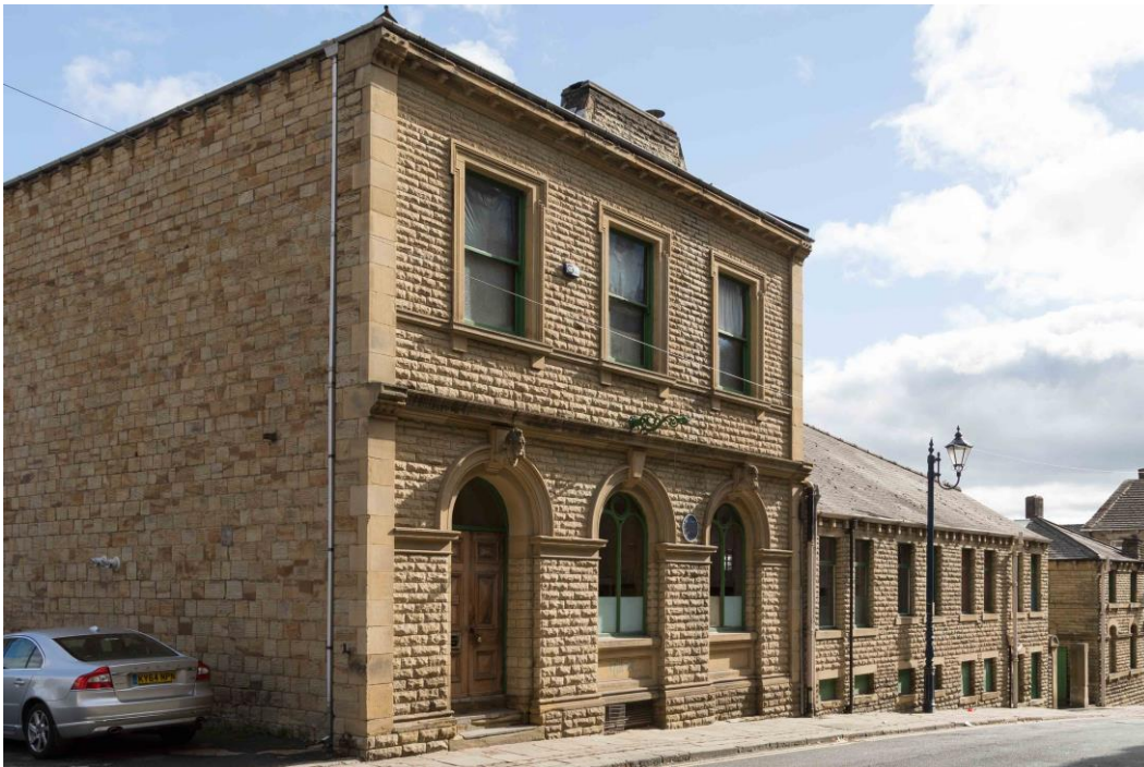
Figure 11: Auction house, 4 Grove Street; note carved heads to the main entrance and window keystones
