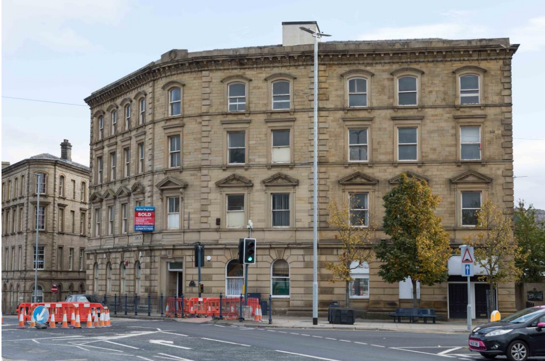
Figure 9: Textile Warehouse examples. Clockwise from top left: 9-13 Wellington Road East, one of few non-Italianate designs; Plan and section for 24 Bond Street/19 Croft Street showing cast iron structure (note columns in centre of section); 'show front' of Field House, 15 Wellington Road East
