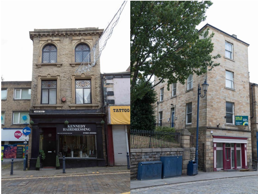
Figure 12: Example shopfronts, from left: 41 Daisy Hill, a small textile warehouse with shop to ground floor; 74 Daisy Hill, shopfront to ground floor of Methodist Minister's House.
