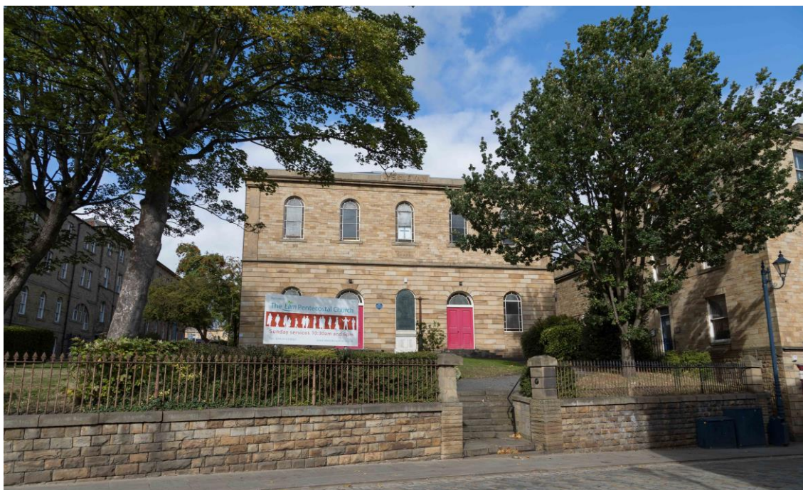
Figure 15: Former Dewsbury Central Methodist Chapel, view north from Daisy Hill, showing garden area, perimeter wall and railings (listed separately at Gd.II) and Minister's House (47 Daisy Hill, to right)
