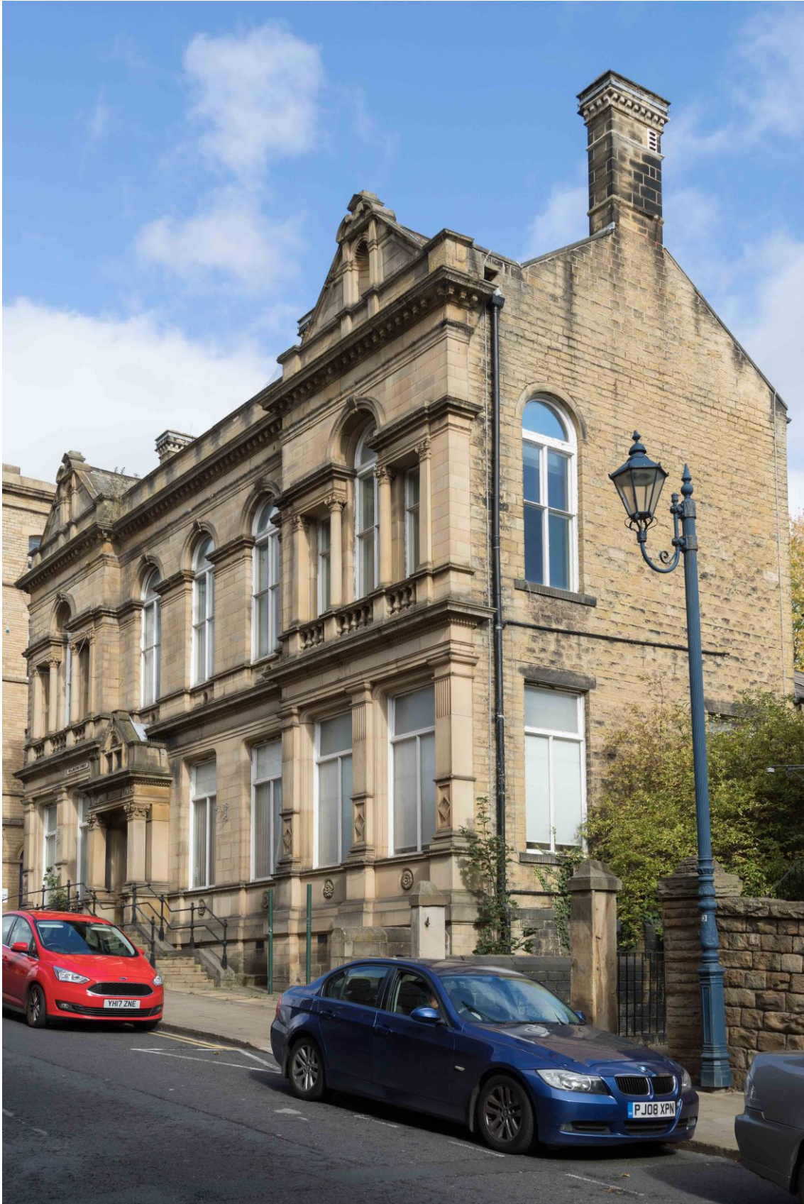
Figure 14: Former Dewsbury Union office, Wellington Street
