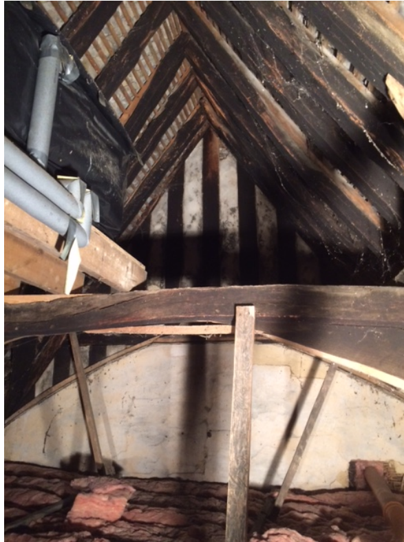
Figure 4: The hall roof, photograph taken from the east (photograph Alison Arnold)
