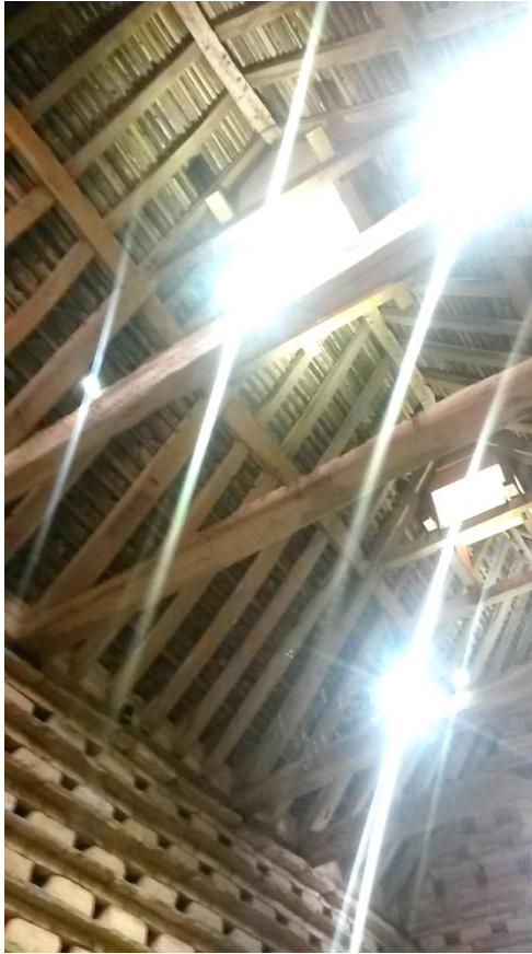
Figure 6: Dovecote roof, photograph taken from the south-west (photograph Alison Arnold)
