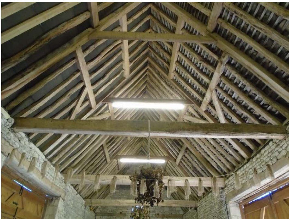
Figure 7: Barn roof, photograph taken from the north-east (photograph Alison Arnold)
