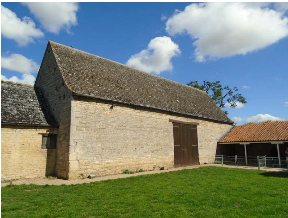
Figure 3: The barn, photograph taken from the south-west (photograph Alison Arnold)
