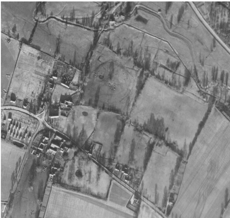
Figure 37 The main area of earthworks at Flempton when still extant in 1947. Photograph RAF/CPE/UK/1921 RP 3003 16-JAN-1947 Historic England Archive (RAF Photography; detail).
