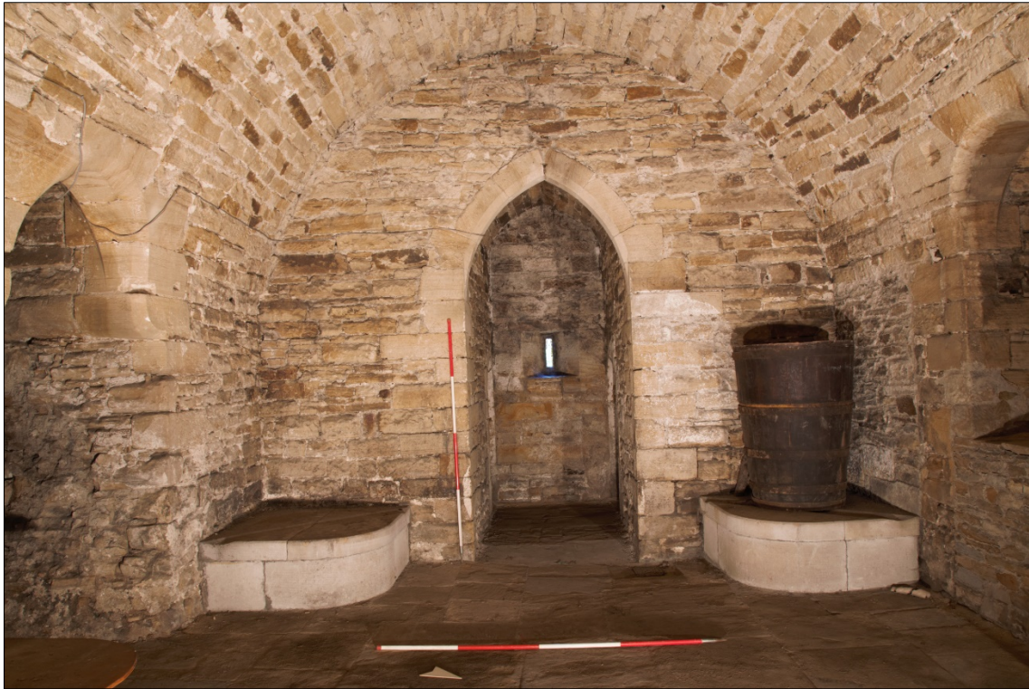
Figure 44: ground floor of the Bulmer Tower looking west. Central arched vestibule (647) leading to two vaulted chambers in the south-west (650) and north-west (658) corners. Original window (648) visible to the rear.
