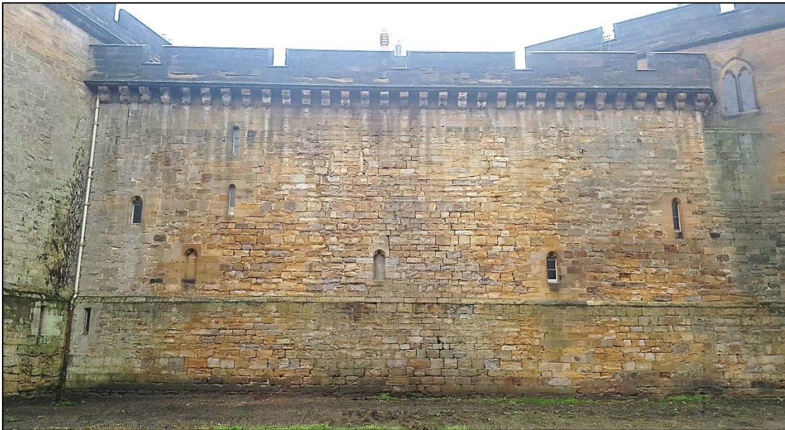
Figure 31: external south-east face of the curtain wall (720) between the Westmorland and Constable towers, showing area of window blocking just beneath the parapet.
