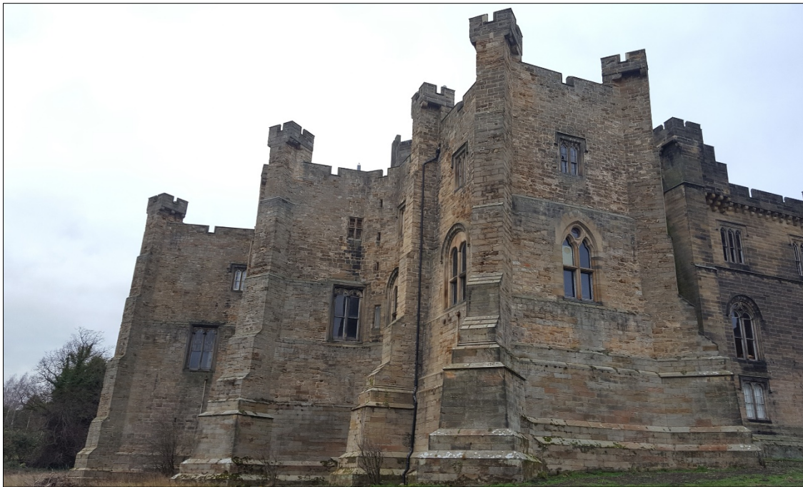
Figure 22: the three towers of the south-west group (Neville (foreground), Link and Bulmer). The buttresses and stepped parapets (now lost) created the impression of a double-fronted façade, looking the same when viewed from the south-east and the south-west. See also Figure 33.
