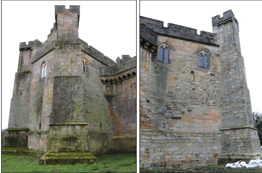
Figures 26 and 27: (left) Westmorland Tower looking south-east. Note the large buttress in contrast to those of the south-west range (115), and (right) the south-facing elevation (130) with one surviving medieval window (133).
