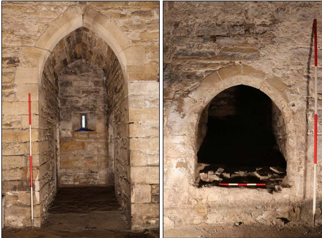
Figures 23 and 24: (left) pointed-arch vestibule in the Bulmer Tower (649) and (right) entrance to intramural stair in the Link Tower (554).
