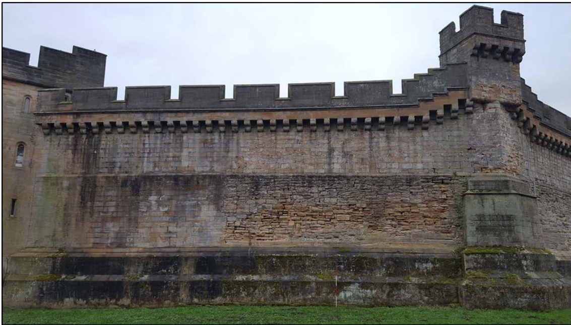
Figure 25: variation in building types. Earlier rubble walling visible on lower section of wall (762) and ashlar build above (763).
