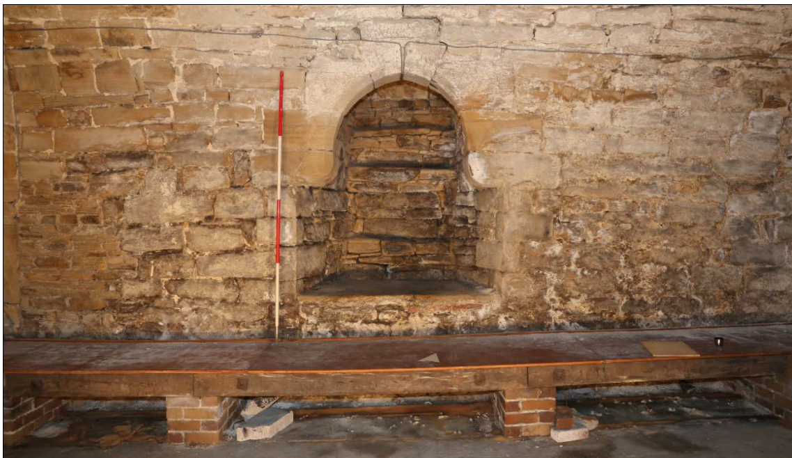
Figure 47: north-east corbelled window with stepped cill (668).
