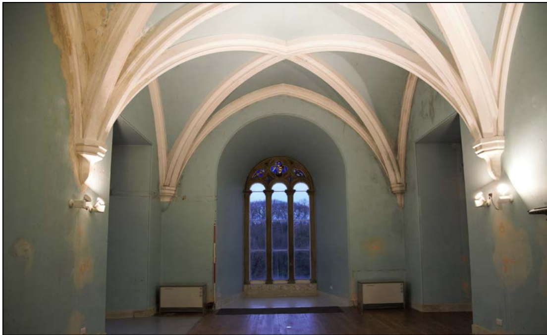
Figure 51: the first floor of Bulmer Tower – known as the Baron's Hall – with quadripartite vaulting featuring roll moulded (681) and plain corbels (682).
