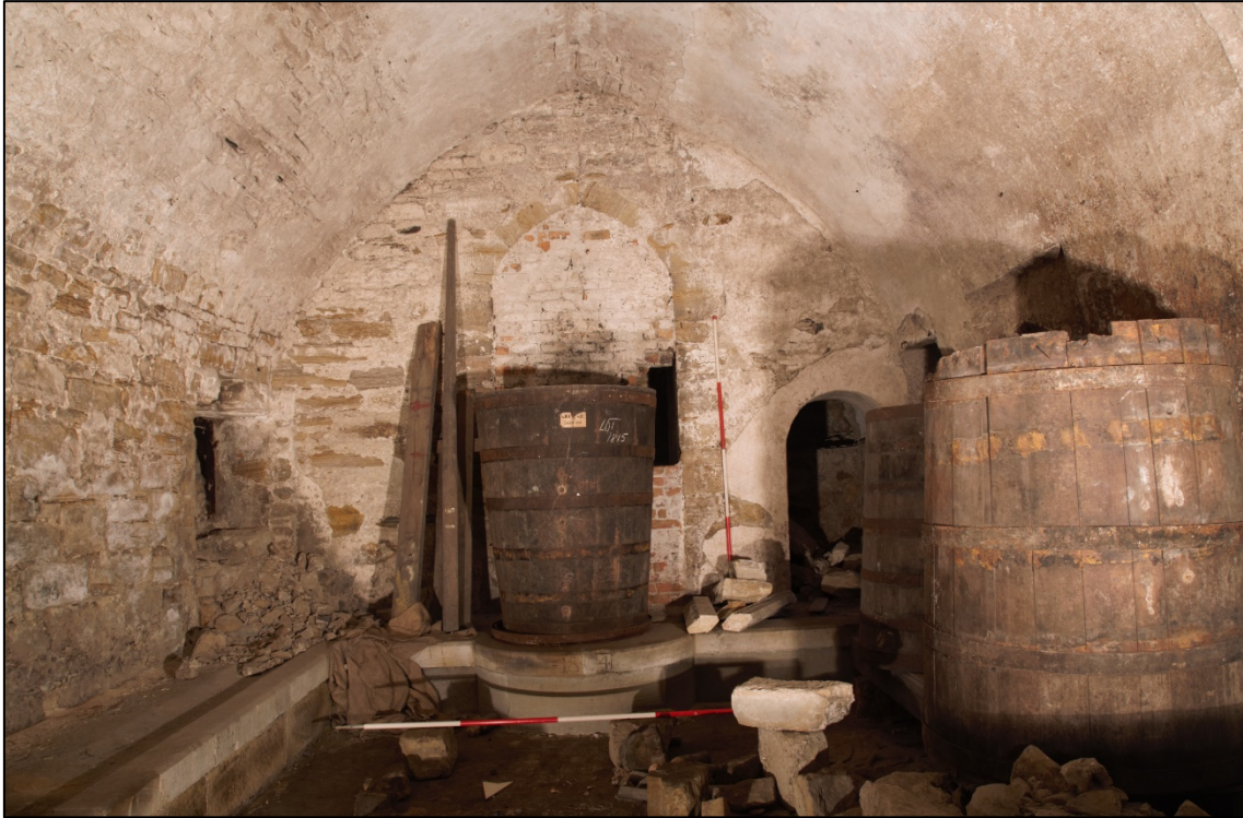
Figure 42: ground floor of the Link Tower looking south. Central is the blocked arch (557) with later rounded-arched door (561) leading into the intramural space. On the left side the iron framed recess (556) is just visible.
