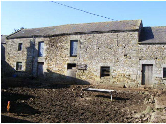
Combination barns. Combination barns of this large scale (above, left) with attached horse engine houses (above, right) are rare in this area. The threshing machine was located on the upper floor of the barn to the right, where ventilation was provided by slits in the stonework and also clay pipes were used for land drainage. Doors provide access to cattle housing below, and note also the raised walkway around the site of the midden or dungheap. This example dates from the peak of agricultural expansion and improvement in the 1840s to 1870s. Photo © Jen Deadman
