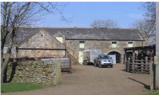
A regular L-plan range in Upper North Tynedale. A cow house attached to a storeyed combination barn. Visible to the left are steps to a first-floor granary above a stable to the left of hemmels for cattle: the threshing barn is sited further to the left. Photo © Jeremy Lake
