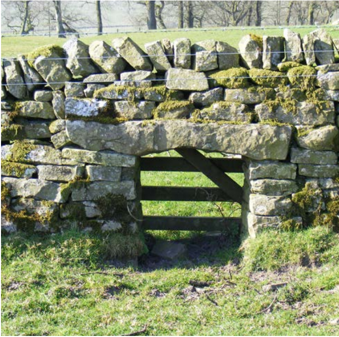
Sheep creep. A 'sheep creep' to enable the movement of sheep through walls and between fields and moorland. Photo © Jen Deadman
