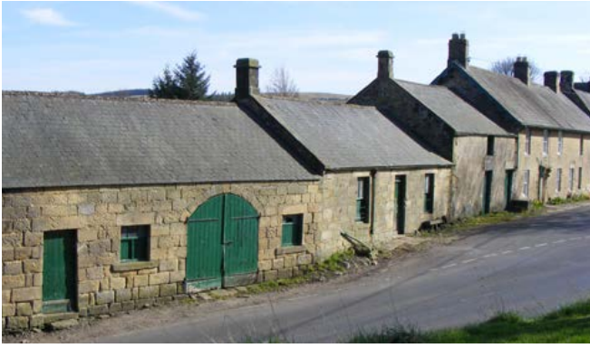
The stepped roofs of this linear range in Elsdon, comprising stables, cart shed with loft over, two cottages and farmhouse, is an arrangement commonplace to the east of this area and the North York Moors. Elsdon continued to thrive due to its position astride drove roads from Scotland. Photo © Jen Deadman
