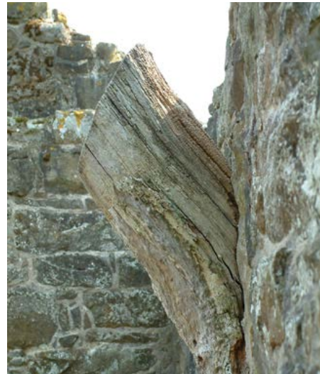
The bases of three sets of roof trusses, possibly of cruck construction, remain. They spring from below eaves level. Photo © Jen Deadman
