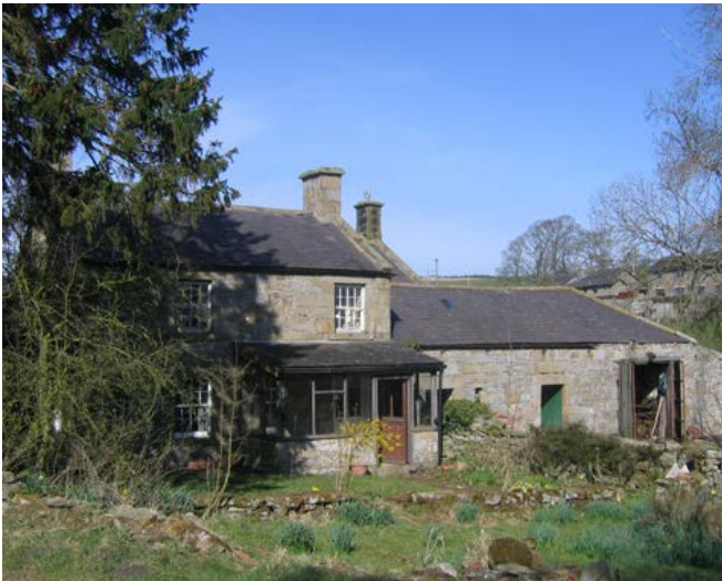
Another linear farmstead in Upper Redesdale, with cattle housing and a stable close to the house. This consists of a mid-19th-century rebuilding of an earlier range. Photo © Jen Deadman
