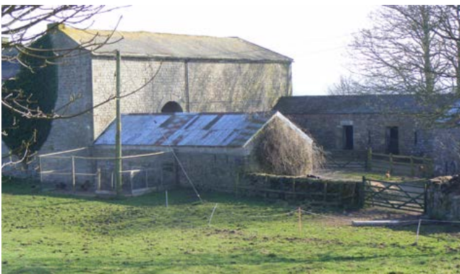
This regular U-shaped farmstead near to Gisland has single-storey cow houses flanking a storeyed combination barn. Photo © Jen Deadman
