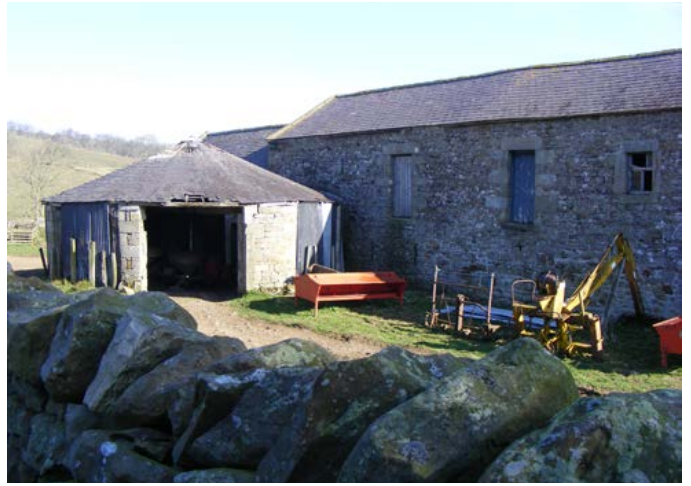
Combination barns. Combination barns of this large scale (above, left) with attached horse engine houses (above, right) are rare in this area. The threshing machine was located on the upper floor of the barn to the right, where ventilation was provided by slits in the stonework and also clay pipes were used for land drainage. Doors provide access to cattle housing below, and note also the raised walkway around the site of the midden or dungheap. This example dates from the peak of agricultural expansion and improvement in the 1840s to 1870s. Photo © Jen Deadman
