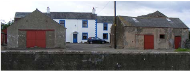
Mid-19th-century roadside steading with rendered farmhouse facing the farmyard, and the buildings left characteristically unrendered. Photo © Jen Deadman
