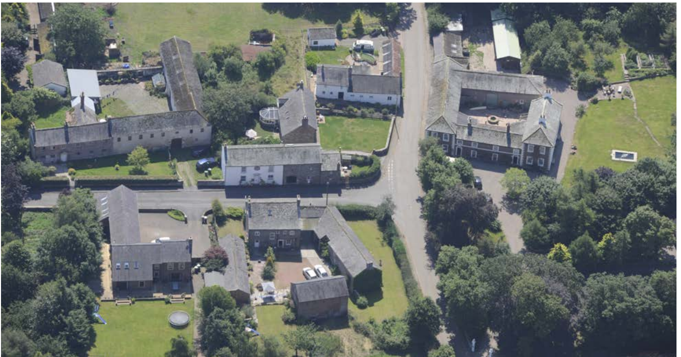
The white-painted linear range at the centre of this photograph of Longburgh is late 17th century, and is clay-walled and cruck-framed. To its right (west) is Longburgh House, a relatively high-status courtyard group including a large barn built in and after 1782. To the left of the image is Longburgh Farm with its late 17th-century house (also clay-walled) with an attached late 17th- or early 18th-century barn range with a malting floor. Photo © Historic England 28577/053
