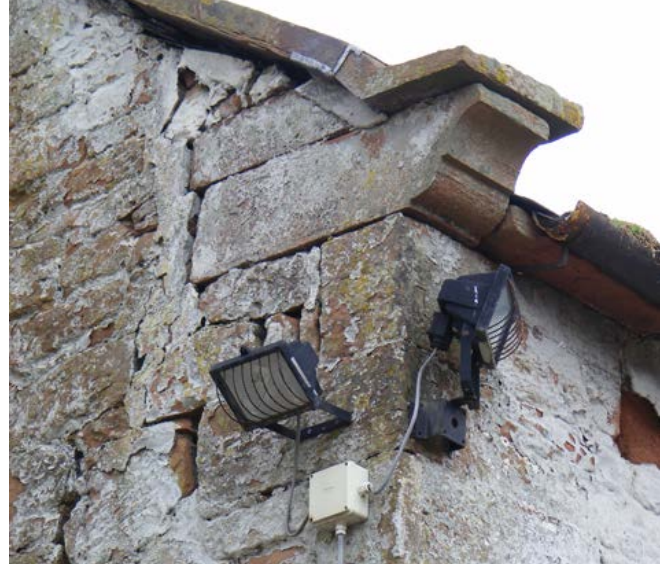
Typical carved stone kneeler to a stone-coped gable end. Photo © Jen Deadman
