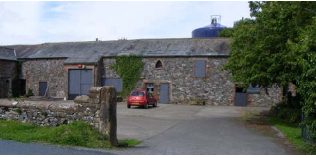
Here, a combination barn of 1836 with a projecting porch dominates the street but is set back behind its yard. It is built entirely of cobble with sandstone dressings to the openings. Photo © Jen Deadman
