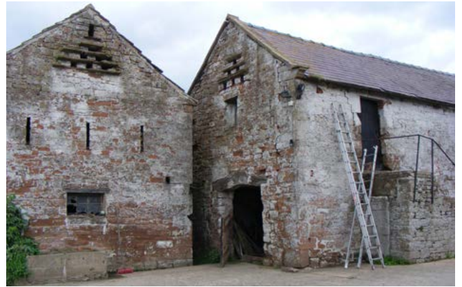
These 18th-century combination barns are two of three set around a small yard. One building retains its stone slate roof. The majority of early barns have now been re-roofed in blue slate. Photo © Jen Deadman
