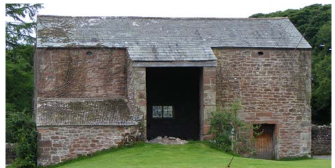
The majority of combination barns of the late 18th and 19th centuries provide the traditional layout of central threshing floor flanked by a lofted byre and full height hay mow. Frequently the combination barn is the main and sometimes the only agricultural building, as here. Note the ramped entry onto the threshing floor and unusual oval vents at eaves level. The projecting porch of the entry to the threshing bay is a common feature. Photo © Jen Deadman
