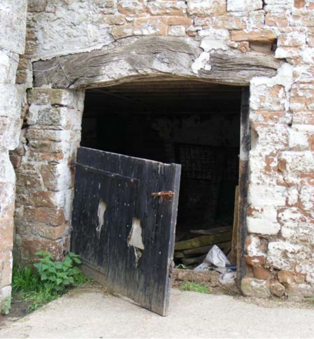
Timber, probably from a cruck-framed building, re-used as a lintel to a doorway. Photo © Jen Deadman
