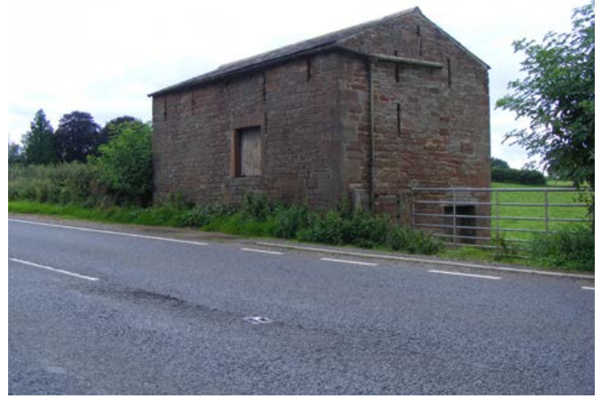
Field barns with side-wall entries for pitching in hay. Note the muck hole for throwing out manure below the door to the left. Photo © Jen Deadman
