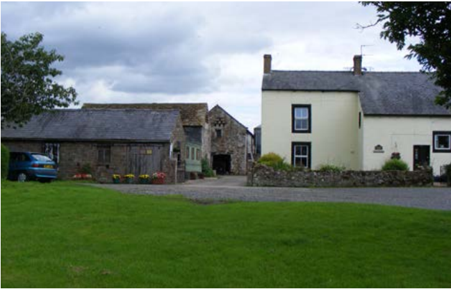
These 18th-century combination barns are two of three set around a small yard. One building retains its stone slate roof. The majority of early barns have now been re-roofed in blue slate. Photo © Jen Deadman
