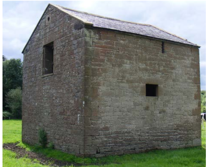
Small-scale field barn for cattle and the storage of hay. Photo © Jen Deadman
