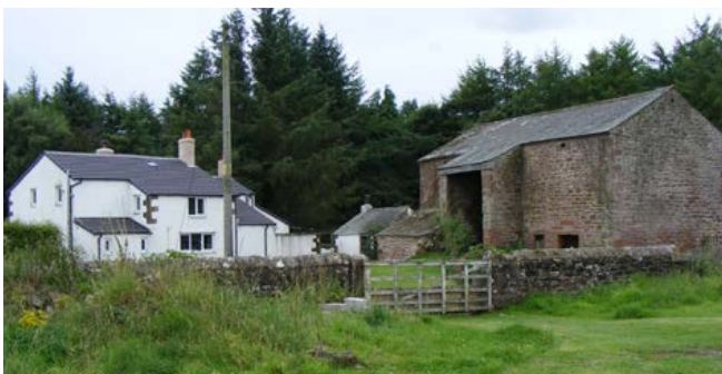
The majority of combination barns of the late 18th and 19th centuries provide the traditional layout of central threshing floor flanked by a lofted byre and full height hay mow. Frequently the combination barn is the main and sometimes the only agricultural building, as here. Note the ramped entry onto the threshing floor and unusual oval vents at eaves level. The projecting porch of the entry to the threshing bay is a common feature. Photo © Jen Deadman
