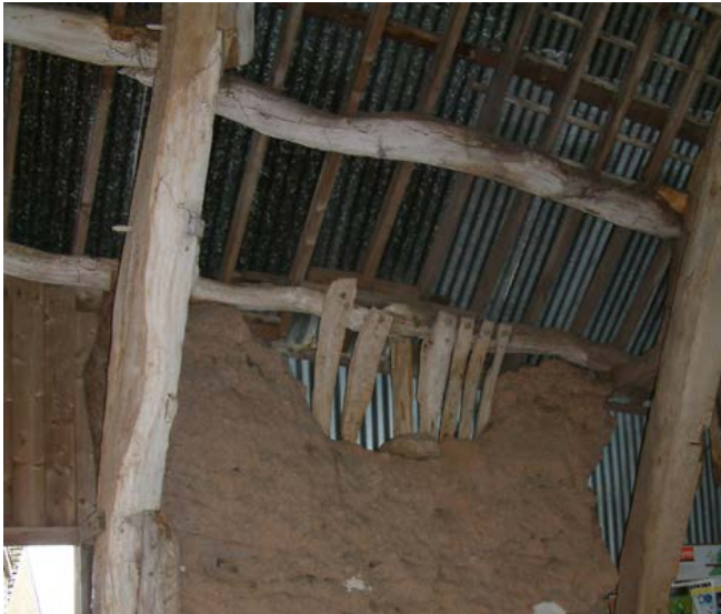
Full-height crucks, sometimes supporting local staple thatch, and mass clay walling set on cobble plinths, are still in evidence in many older farmhouses and outbuildings. In this large five-bay barn, areas of clay walling remain. The gable end has been replaced in brick. Early windows of clay barns consisted of an opening at the top of the wall, partly covered by riven oak laths pegged to a beam, as shown to the right. Photo © Jen Deadman
