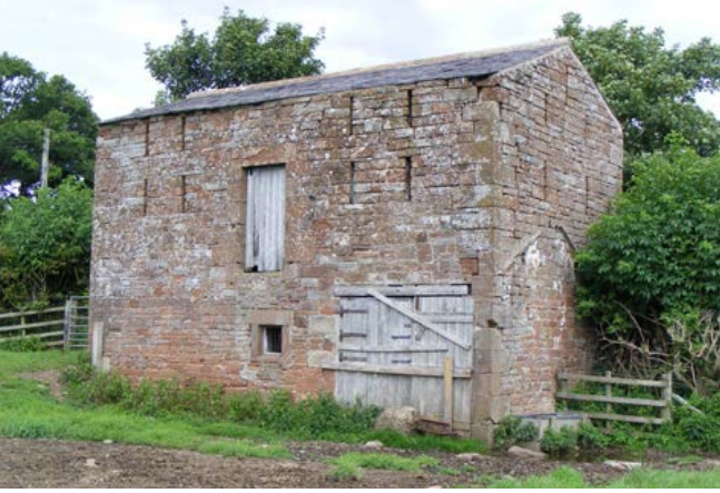
Field barns with side-wall entries for pitching in hay. Note the muck hole for throwing out manure below the door to the left. Photo © Jen Deadman
