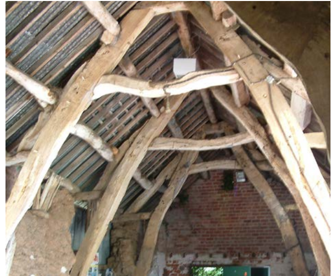
Full-height crucks, sometimes supporting local staple thatch, and mass clay walling set on cobble plinths, are still in evidence in many older farmhouses and outbuildings. In this large five-bay barn, areas of clay walling remain. The gable end has been replaced in brick. Early windows of clay barns consisted of an opening at the top of the wall, partly covered by riven oak laths pegged to a beam, as shown to the right. Photo © Jen Deadman
