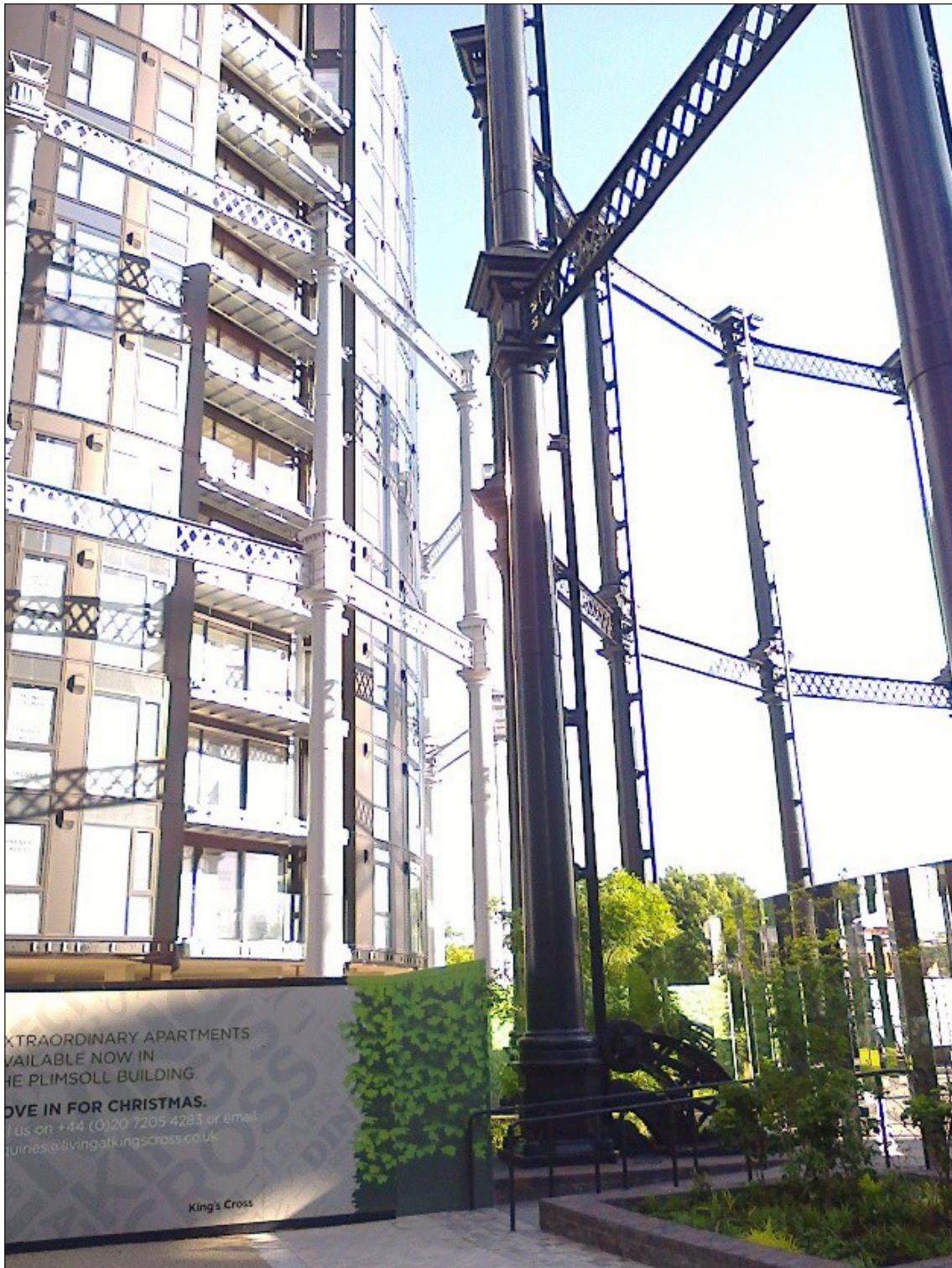
Figure 2.72 The Redeveloped Gasholders at the new Kings Cross/St. Pancras redevelopment. Source R.Thomas.
