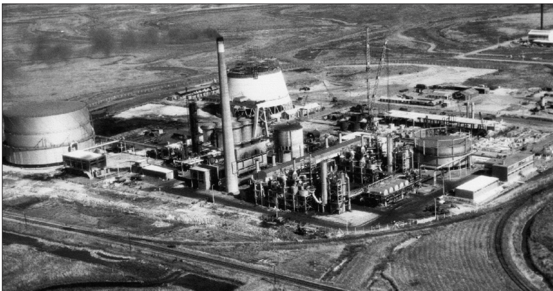
Figure 2.62, The Isle of Grain SEGAS plant. Source National Grid Gas Archive.
