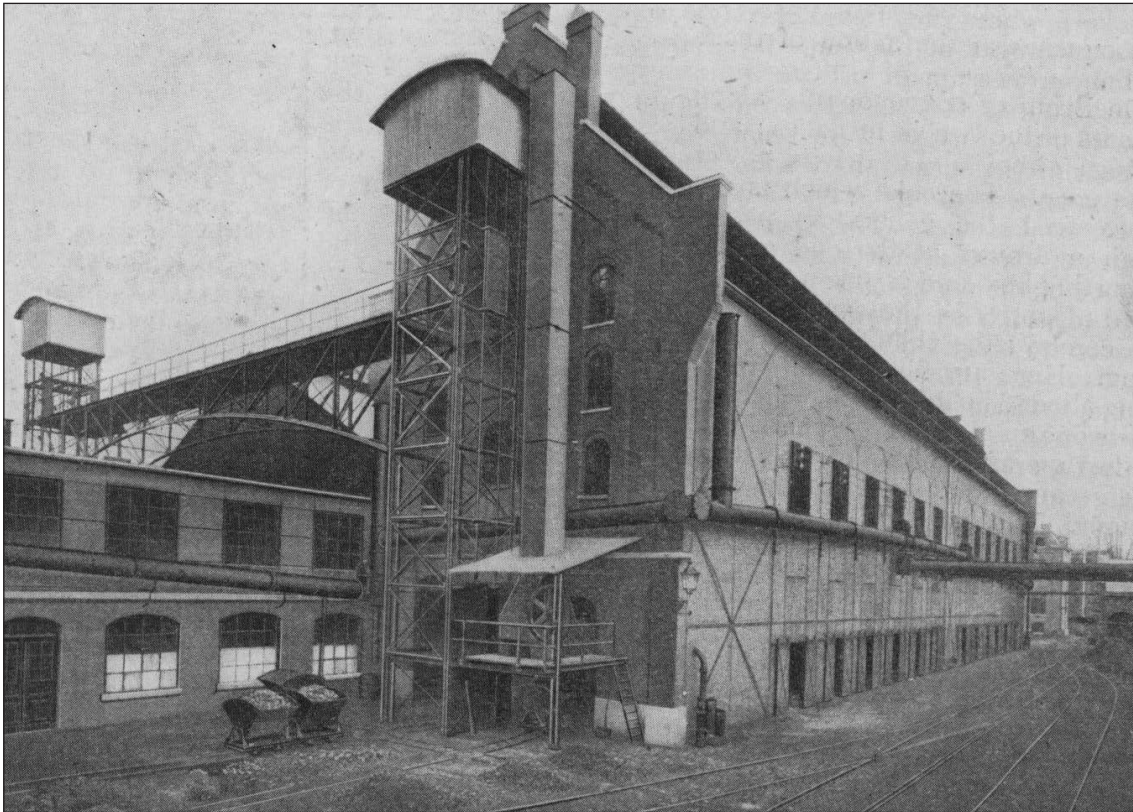
Figure 2.38. A view of the Vertical retort house built at the Forest Gasworks of the ICGA in Brussels, Belgium, 1910. Source IGEM Archive.
