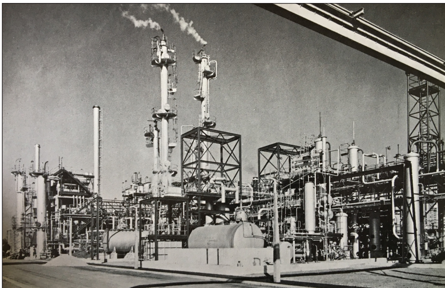
Figure 2.63, The Gas Reforming and Gas Recycle Hydrogenator Plants at the Seabank Gasworks, Avonmouth, Bristol. Source National Grid Gas Archive.
