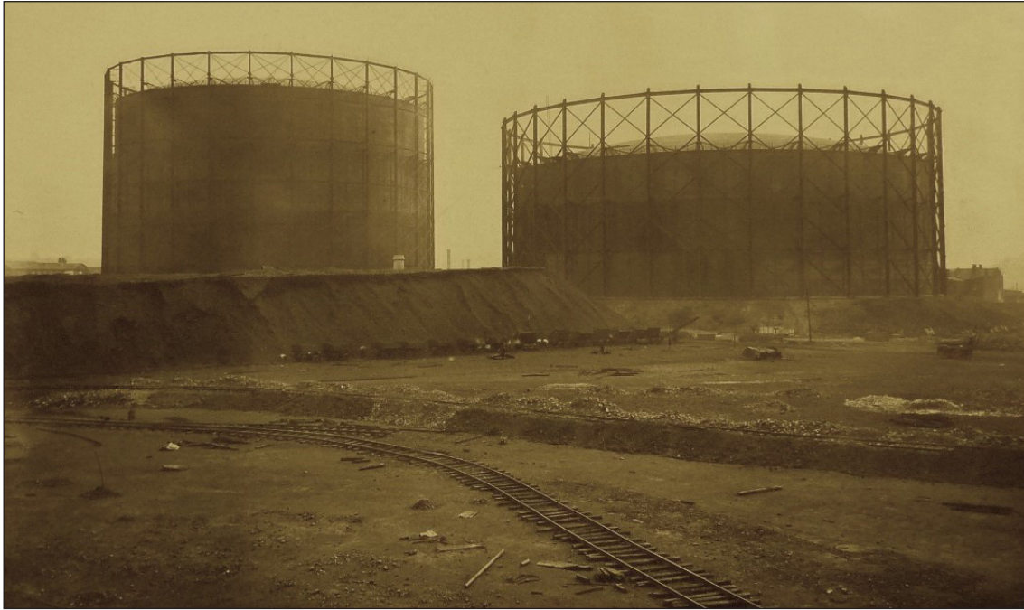
Figure 2.48. Gasholders No.1 and No.2 at the former East Greenwich gasworks. Source National Grid Gas Archive.
