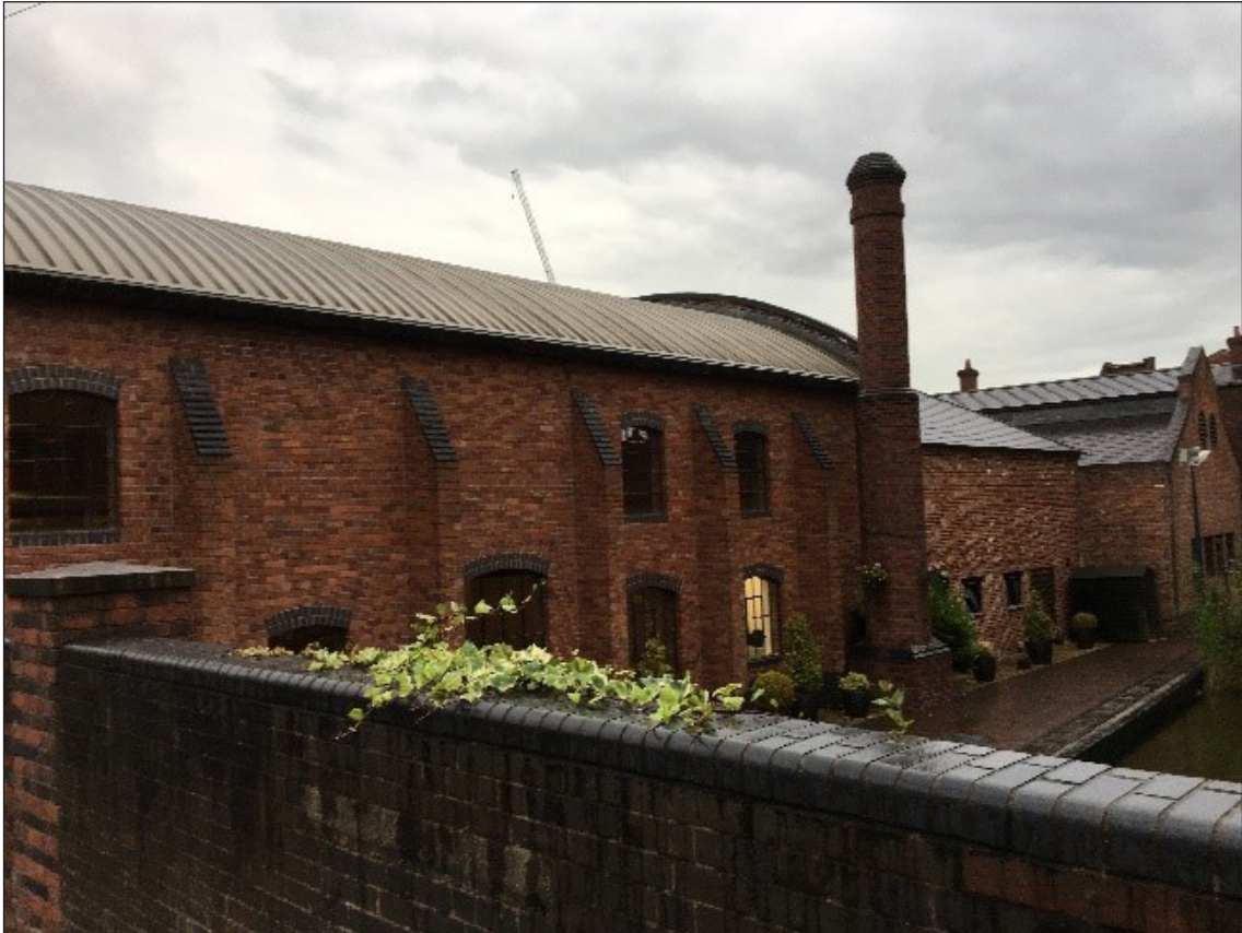
Figure 2.20 The recently restored Gas Street gasworks buildings in Birmingham. Source R. Thomas 2017
