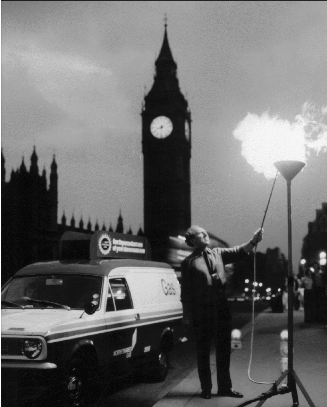
Figure 2.68, Flaring off town gas from the distribution network outside the Houses of Parliament during the conversion programme. Source National Grid Gas Archive.
