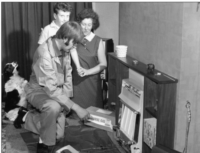
Figure 2.67. The Conversion Programme, the burners in gas appliance had to be replaced with those suitable for natural gas.
