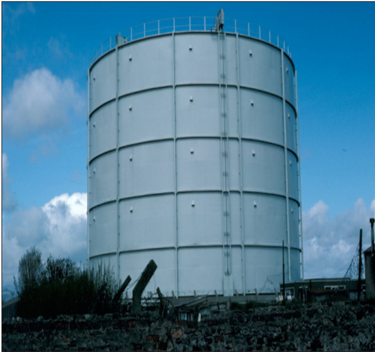
Figure 3.188 Wiggins Type Dry Gasholder at Millom, England. Source Syd Bennett.
