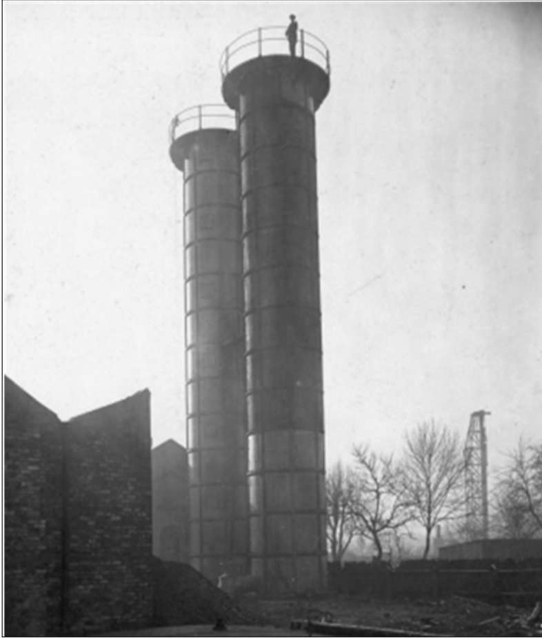
Figure 3.71 Two tower scrubbers. Image courtesy of National Grid Gas Archive.
