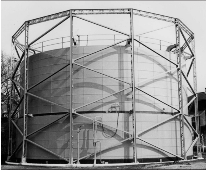
Figure 3.177 A two-lift frame-guided gasholder with below-ground tank, using Cutler's patented system, Southern England. Image courtesy of IGEN Archive.
