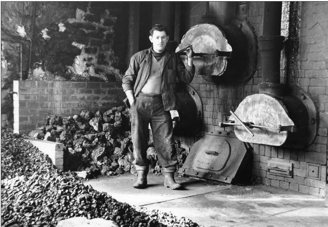
Figure 3.16 A stoker stood aside the retorts of the very small gasworks in Robin Hood's Bay, Yorkshire. Image courtesy of IGEN archive.
