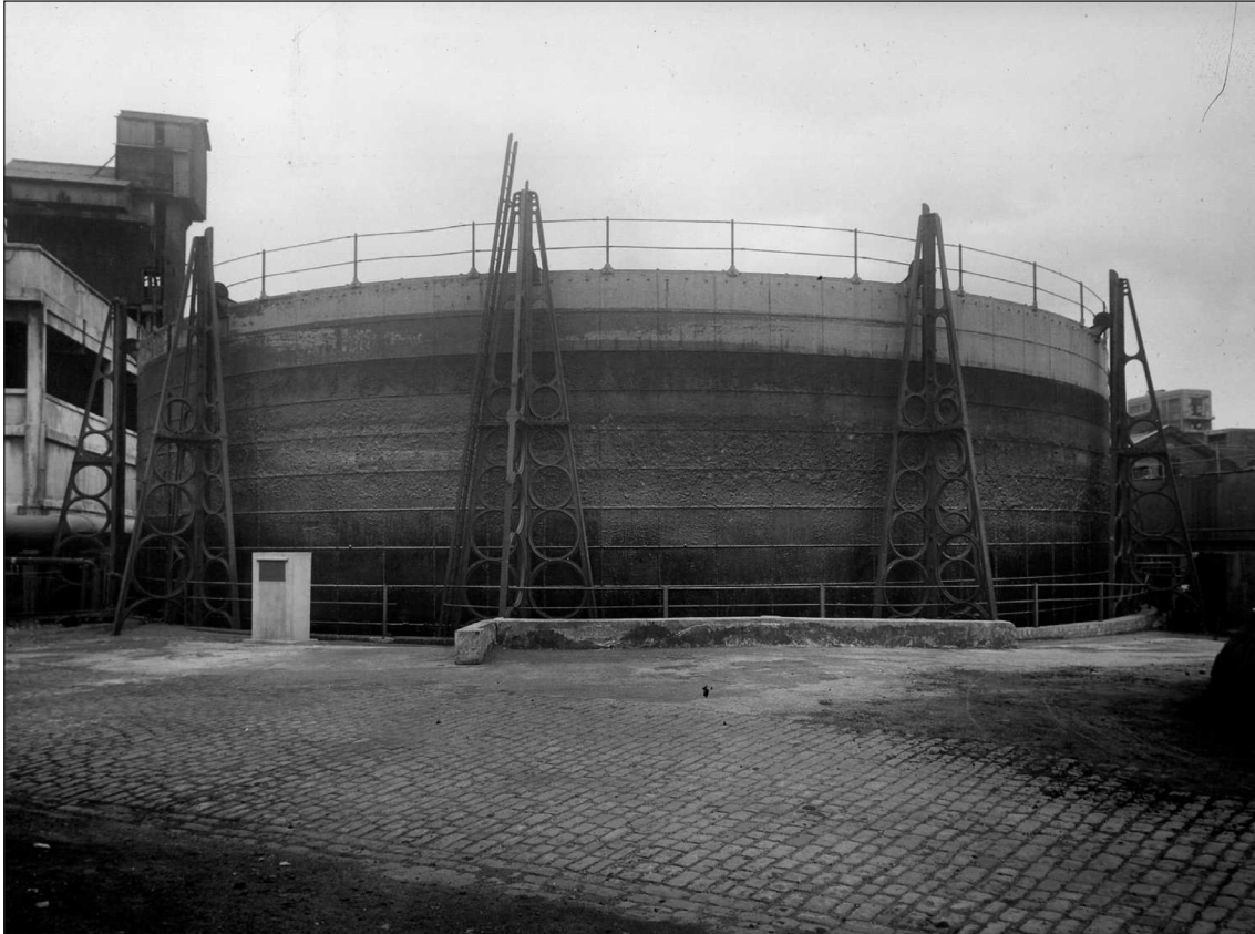
Figure 3.160 No.2 Gasholder Fulham whilst still operational in 1951, built circa 1830 and attributed to John Kirkham and Samuel Clegg. Image courtesy of IGEM Archive.
