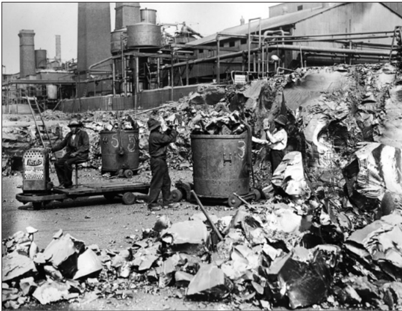
Figure 3.194 Breaking up pitch in pitch beds at the former East Greenwich gasworks. Image courtesy of National Grid Gas Archive.
