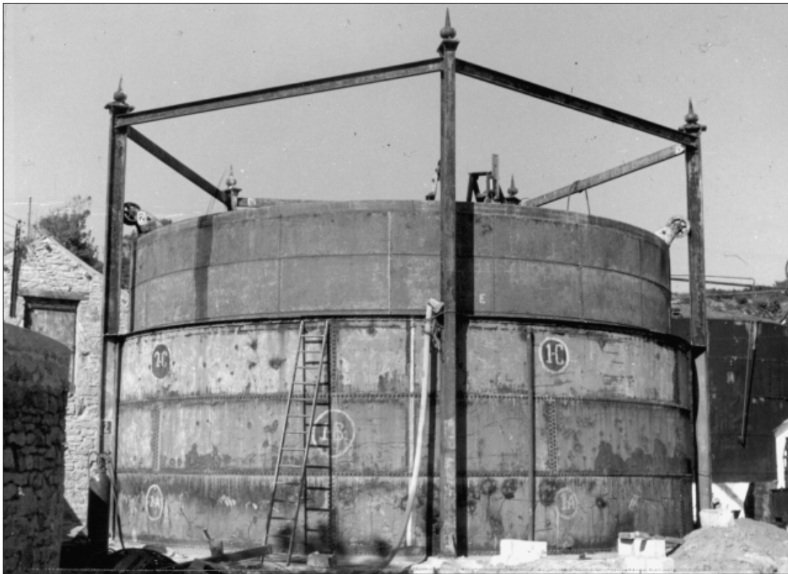
Figure 3.138 A gasholder typical of the type employed as a Water Gas Relief Holder. Image courtesy of the National Grid Gas Archive.
