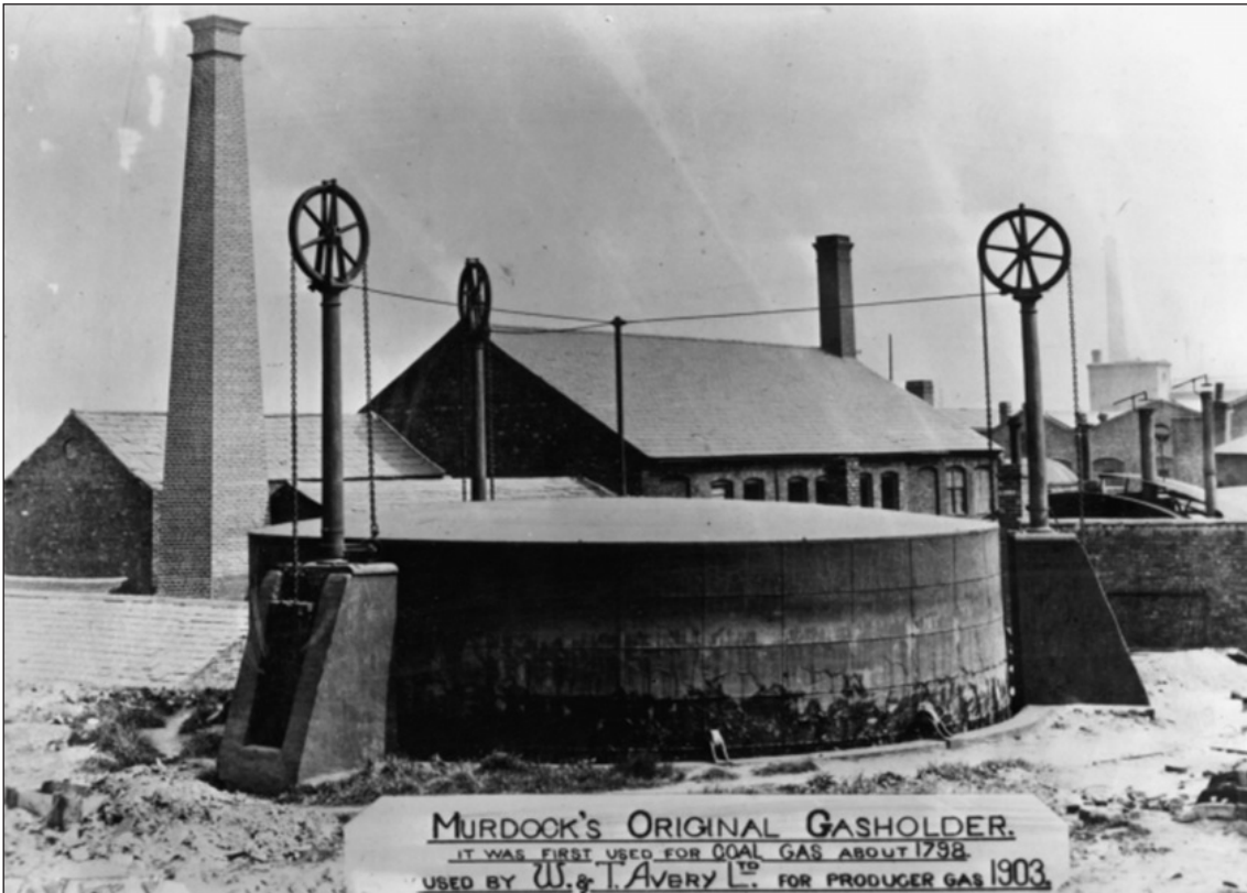
Figure 3.165 The primitive gasholder at the former Soho factory of Bolton and Watt, when under the ownership of Avery in 1903, still being used to store producer gas. Although an early design, is not believed to be directly attributable to Murdock. Image courtesy of National Grid Gas Archive.
