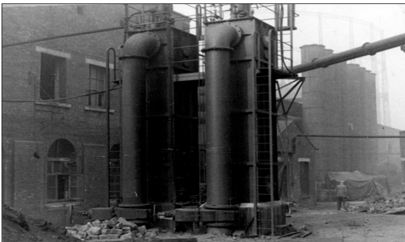
Figure 3.137 Condensers used on an H&G Carburetted Water-Gas Plant. Image courtesy of National Grid Gas Archive.
