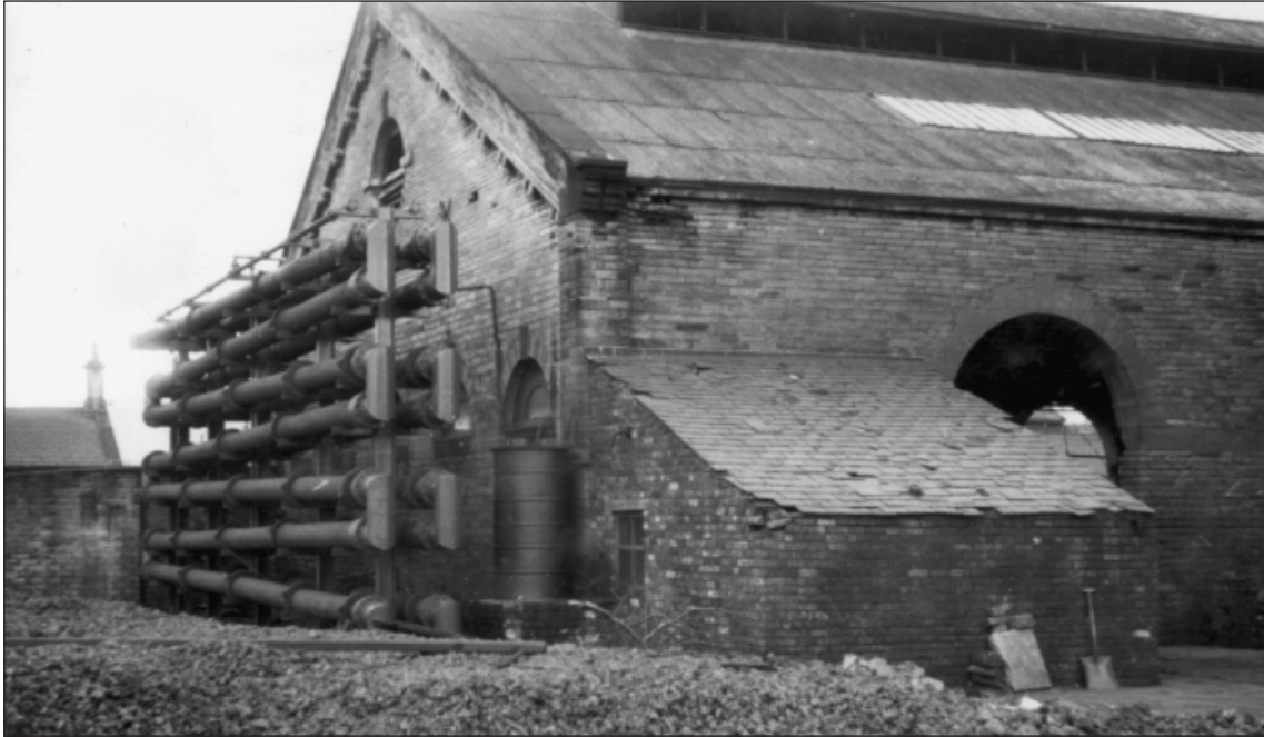
Figure 3.58 A Zig-Zag Horizontal Atmospheric condenser positioned next to the retort house. Image courtesy of National Grid Gas Archive.
