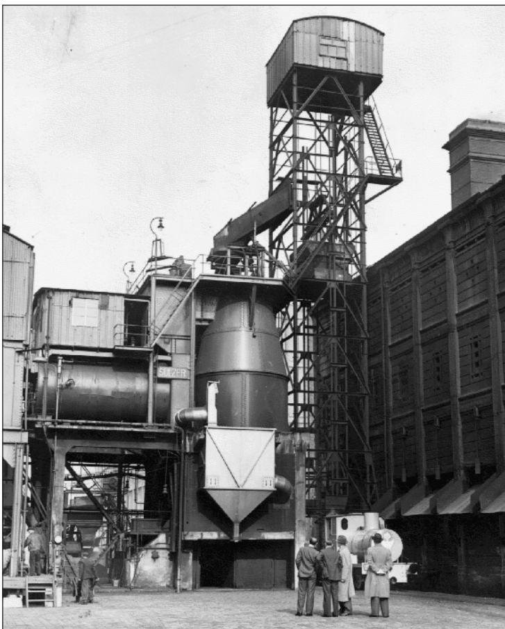
Figure 3.106 Sulzer Plant and fireless locomotive, Oswald Street gasworks, Burnley 1954. Image courtesy of National Grid Gas Archive.
