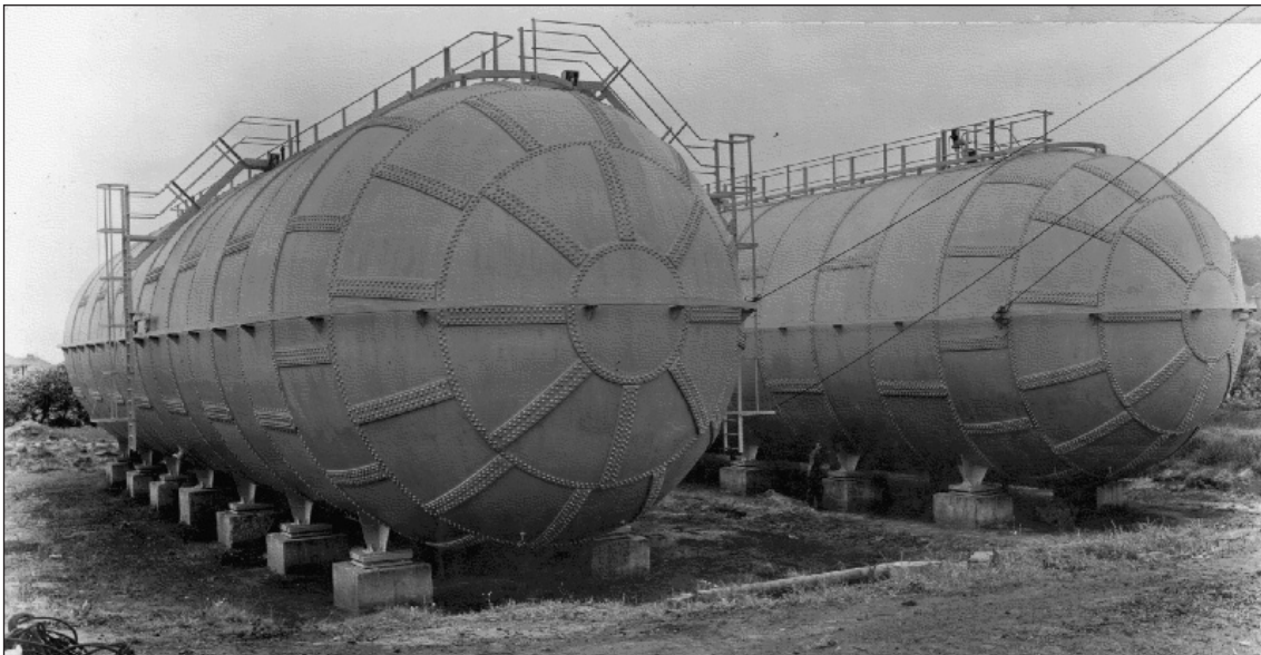
Figure 3.190 Early high pressure bullet gasholders at the former Oakengates gasholder station Shropshire. Image courtesy of National Grid Gas Archive.
