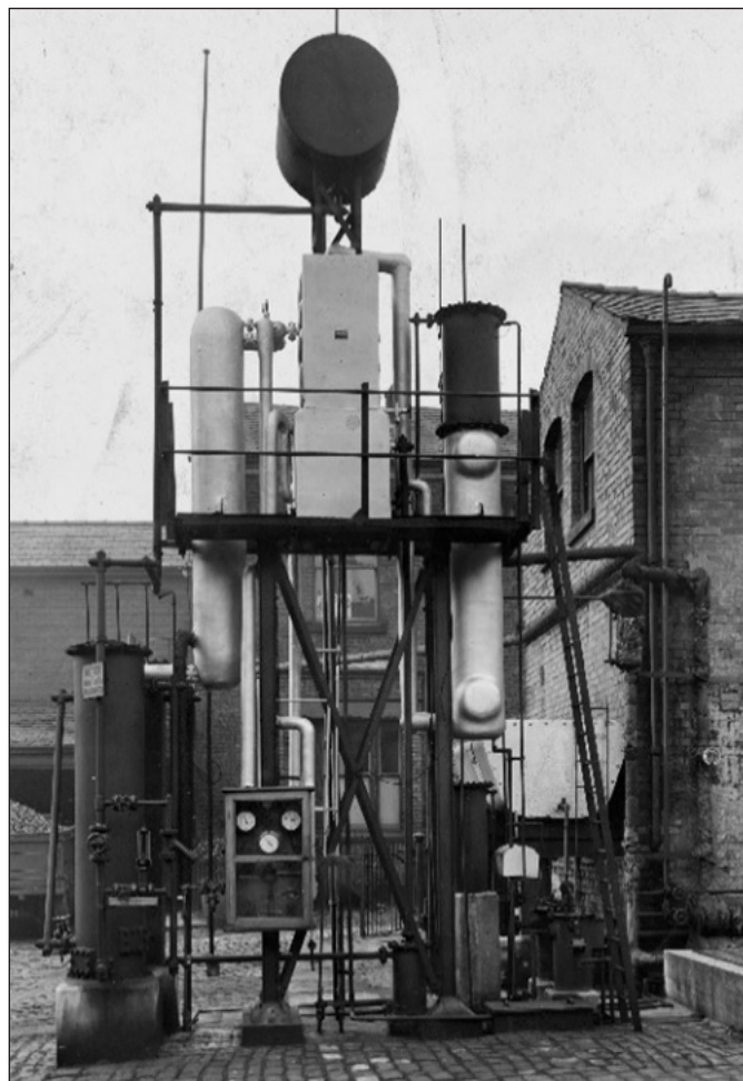
Figure 3.86 A small benzole plant at the former gasworks in Middleton, Lancashire. Image courtesy of National Grid Gas Archive.
