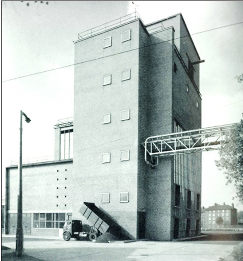
Figure 3.103 Babcock and Wilcox Boiler House Bromley by Bow Gasworks. Image courtesy of National Grid Gas Archive.
