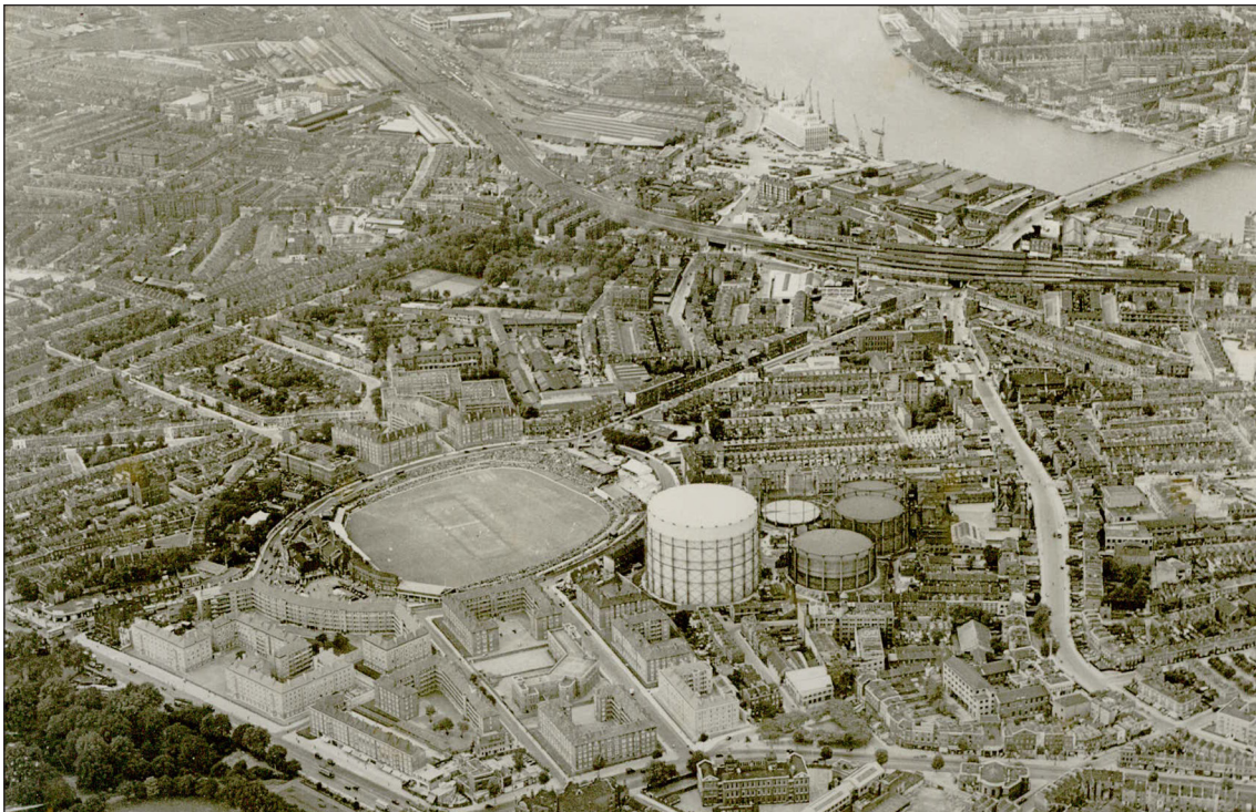
Figure 3.178 An aerial photograph of the Kennington Oval Gasholder Station showing No.1 gasholder with the flying lift in use. Image courtesy of National Grid Gas Archive.
