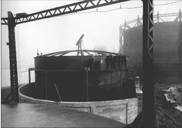
Figure 3.140 Construction of a traditional above-ground oil storage tank at Brentford Gasworks in 1929, showing the perimeter wall protecting the tank and the construction of the tank roof and walls. Image courtesy of National Grid Gas Archive.
