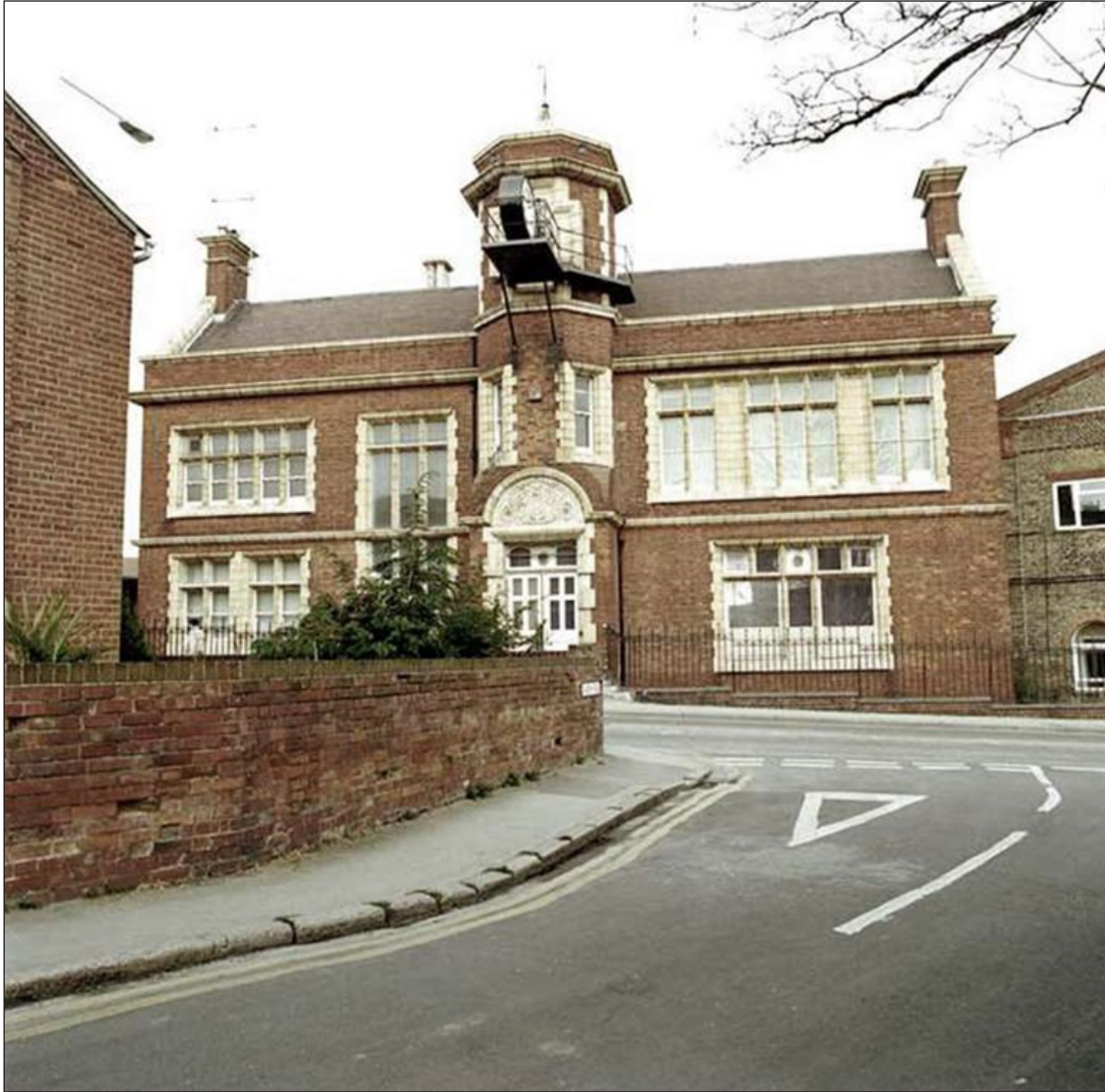
Figure 3.219 The surviving gas offices, Ramsgate, Kent. © Historic England.
