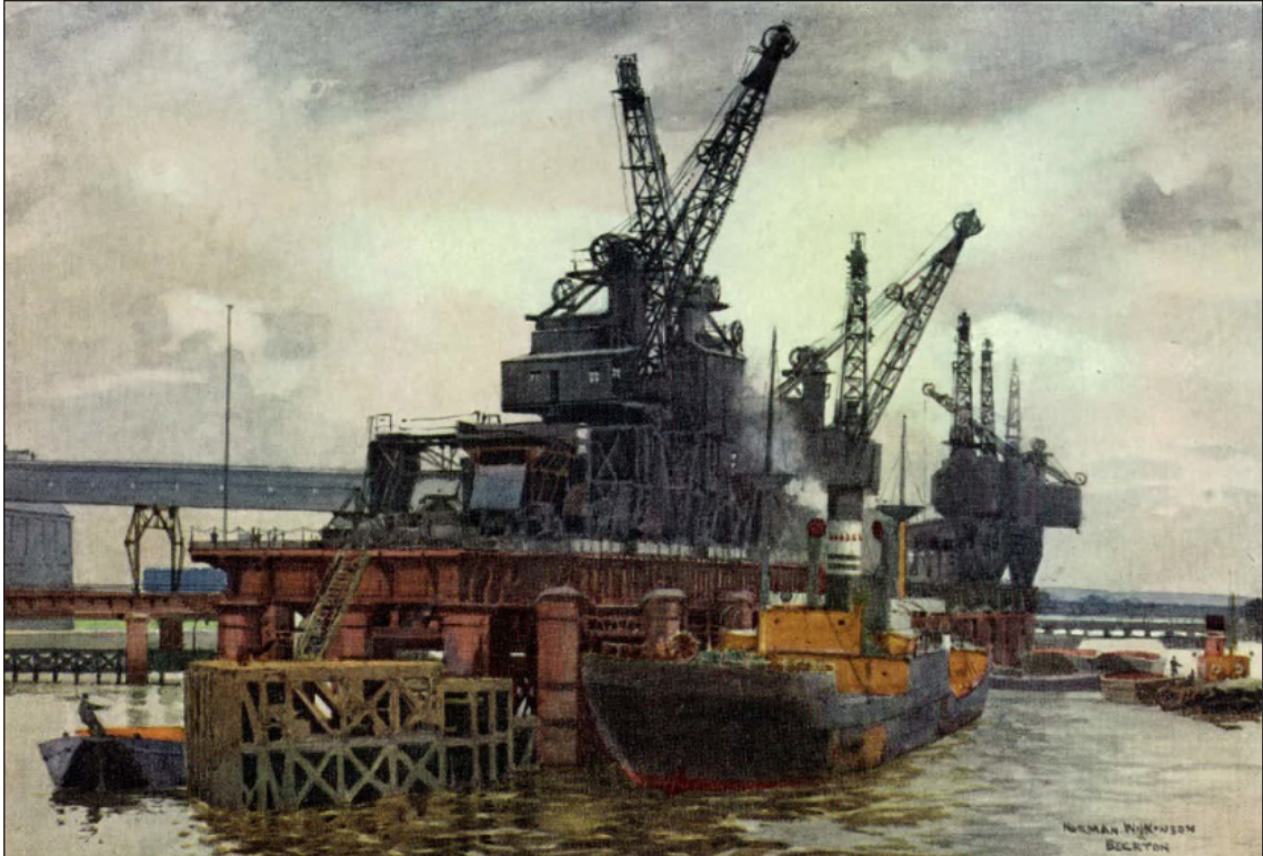
Figure 3.4 Painting by Norman Wilkinson of unloading coal from a coastal collier by steam cranes at the wharf at Beckton. Image courtesy of National Grid Gas Archive.
