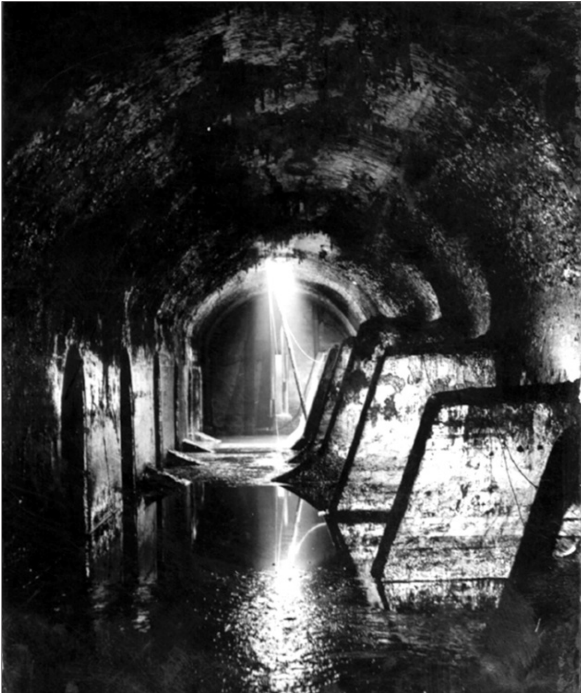
Figure 3.82 Interior of a tar tank at the former gasworks, Sydenham. Image courtesy of National Grid Gas Archive.
