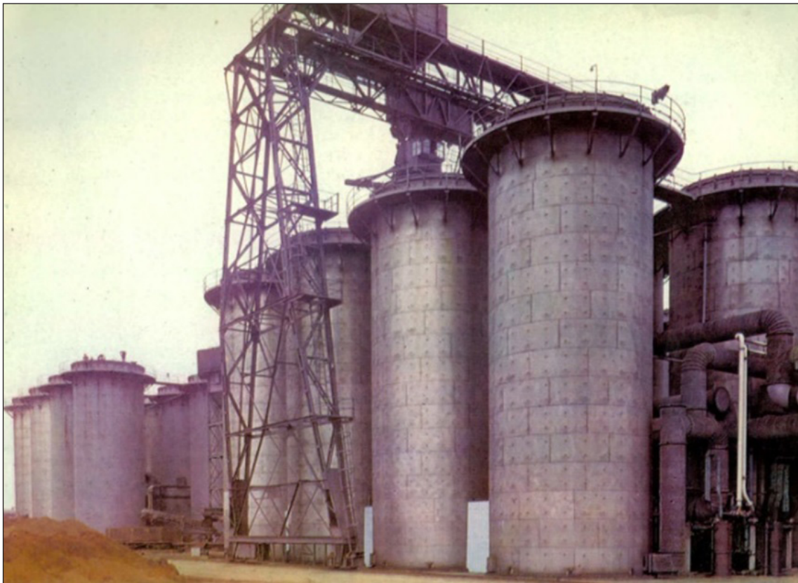
Figure 3.79 Tower purifiers at the former East Greenwich gasworks. Image courtesy of National Grid Gas Archive.
