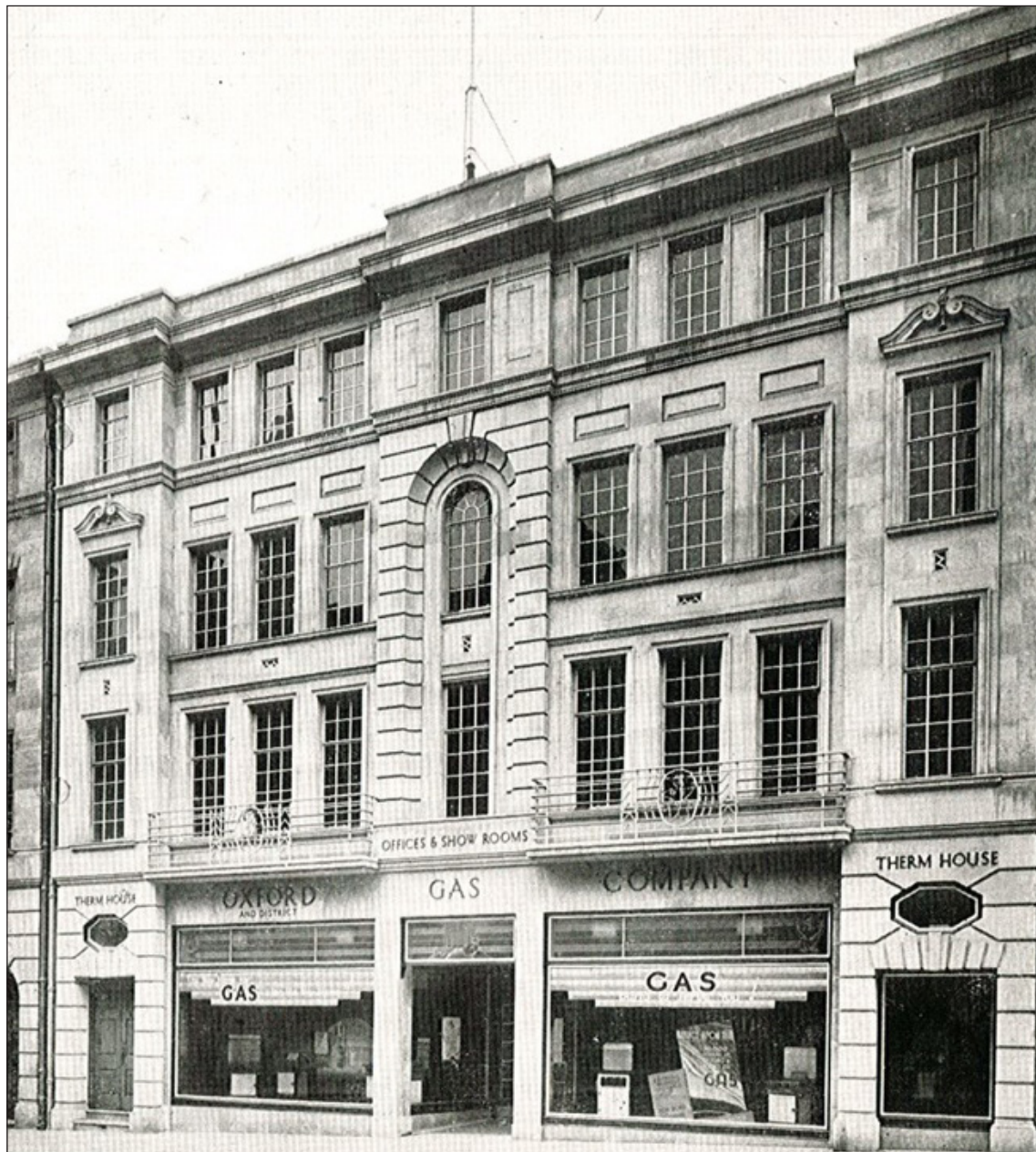
Figure 3.221 Therm House Oxford, the former offices, showrooms, demonstration theatre and homecraft centre of the Oxford Gas Company c1948. Source R. Thomas.
