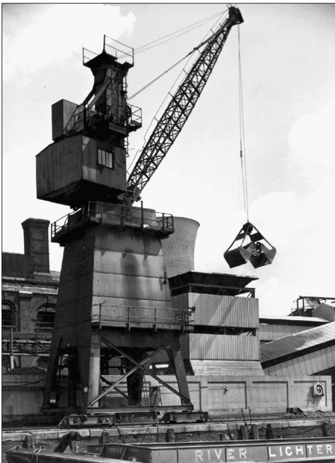
Figure 3.111 Electro-hydraulic crane unloading coal from a barge on the River Lea, Bromley by Bow Gasworks, 1950's. Image courtesy of National Grid Gas Archive.
