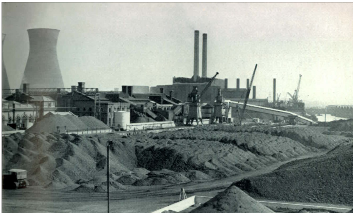
Figure 3.109 Coal Stocking grounds Bromley by Bow Gasworks. Image courtesy of National Grid Gas Archive.
