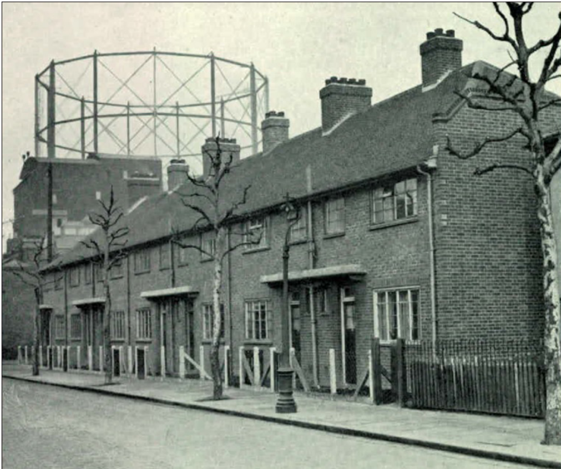
Figure 3.224 SEGAS employee's houses, Rotherhithe, London. Image courtesy of National Grid Gas Archive.
