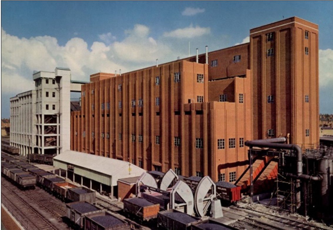
Figure 3.47 The rear of the vertical retort house and coke Screening plant, showing the Wagon tippers for discharging coal. Former Swan Village Gasworks, West Bromwich. Image courtesy of National Grid Gas Archive.
