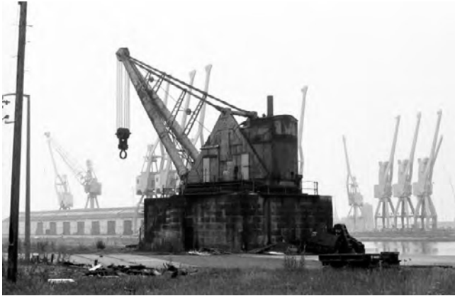
100 ton steam crane, Alexandra Dock. © Chris Allen
