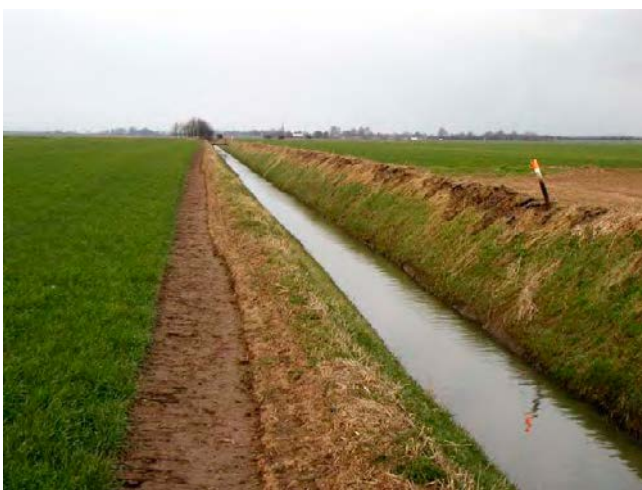
Ottringham Drain. © Andy Beecroft
