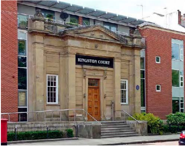
Retention of character in development of former bomb damage plot, Kingston Square. © Stephen Richards
