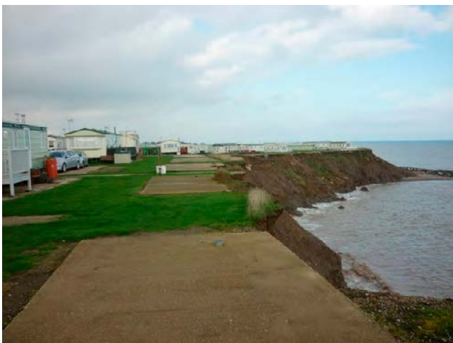
Erosion at Long Beach Leisure Park, Hornsea. © Ian S.
