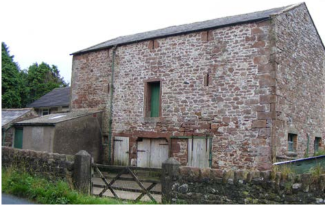
This early 19th-century combination barn forms part of a roadside steading near Seascale. Note the first-floor threshing door over a central cart entry flanked by doors to cattle housing. Photo © Jen Deadman
