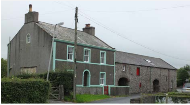
This combination barn at Drigg has been extended to adjoin the house, with an arched entry providing access to the yard behind. Note the rendered treatment to the house, which also offered opportunities to pick out doors, windows, pilaster strips and string courses. Photo © Jen Deadman
