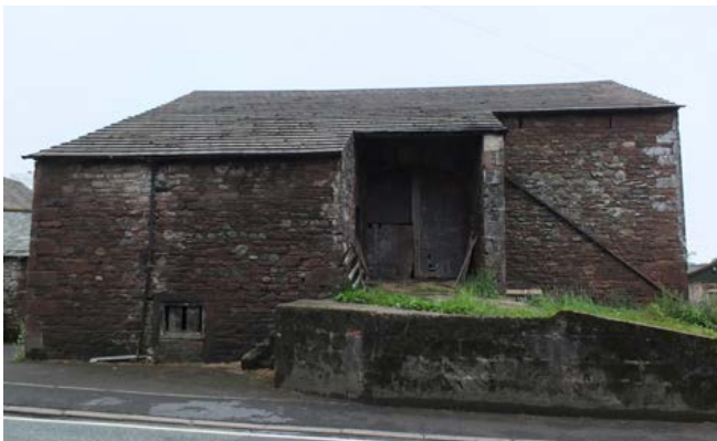
Early 19th-century bank barn at Drigg. The barn is ramped, providing a threshing floor and hay storage at the upper level with cattle housing below. Photo © Jen Deadman
