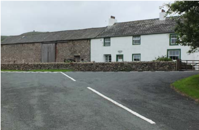
Linear farmstead below the fell edge on the narrow coastal strip to the south-west. The barn is double pile with the rear range a later 18th- or 19th-century addition. The farmhouse is dated 1706 with the date of 1827 possibly celebrating alterations to the farmhouse. Photo © Jen Deadman
