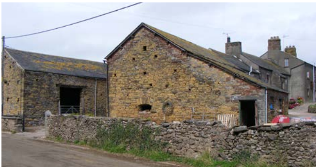
Loose yard arrangement in the village of Stank on the outskirts of Barrow in Furness to the south. The village is comprised solely of several small working farms dominated by combination barns. Note how the roofline of the barn has been raised in red sandstone over the earlier yellow stone common to the south of the area. The voussoirs to the gable-end doorway for cattle indicates an early 18th-century or even earlier date. Photo © Jen Deadman
