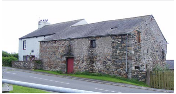
Large, late 18th- to 19th-century combination barn in Drigg associated with a small yard and rebuilt farmhouse. Built mainly of sea cobbles, it was raised at a later date in coursed sandstone. The earlier roof line is evident in the gable end. As elsewhere, there is a small yard fronting onto the roadside before the barn. Photo © Jen Deadman
