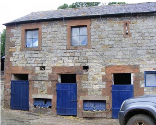
Pig sties with through-feeders and, unusually, a loft above. Note the decorative use of red sandstone for quoins and dressings, a typical feature of this area. Photo © Jen Deadman
