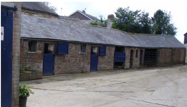
Mid-19th-century single-storey cow houses, probably for the loose housing of calves, the three-bay cart shed to the right converted into cattle housing in the late 19th century. Photo © Jen Deadman
