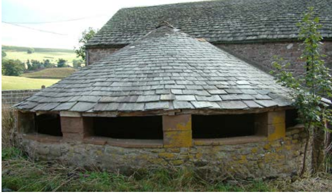
A conical roof to a horse-engine house attached to a combination barn. Photo © Jen Deadman
