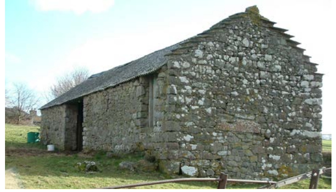
Field barns are not as common in the Eden valley as in other upland areas. Here, on the western fringe this field barn boasts crow-stepped eaves, more commonly seen on buildings in the Cumbrian fells. A blocked doorway in the gable end entered a cow house with a loft over and hay storage adjacent. The neighbouring farm also has crow stepped gables and is late 17th century in date. Photo © Jen Deadman
