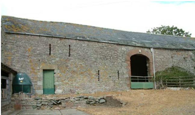
Combination barns are invariably the main agricultural building of the farmstead either as a component part of a yard range or as a freestanding structure. Here, at Pooley Bridge west of Penrith is an early 19th-century combination barn with a cow house to the left, with fine sandstone dressings to the cart entry. This building and the earlier combination barn to the right form two sides of a large yard: it has, from the left, a stable, stone steps to a granary and a hayloft over cattle housing with a blocked cart shed opening to the right. Photo © Jen Deadman
