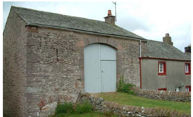
As elsewhere in the north and north-west the combination barn is frequently the main component of the small village farmstead. This small farmstead in Hackthorpe boasts a fine bank barn with direct access from the road via a ramped entry. Farmhouses in this area are frequently rendered and surrounds picked out in a contrasting colour. Here, as in Lancashire there is a greater feeling for rendered surfaces and paint, generated by the porous and unsatisfactory nature of the unprotected sandstone. Photo © Jen Deadman
