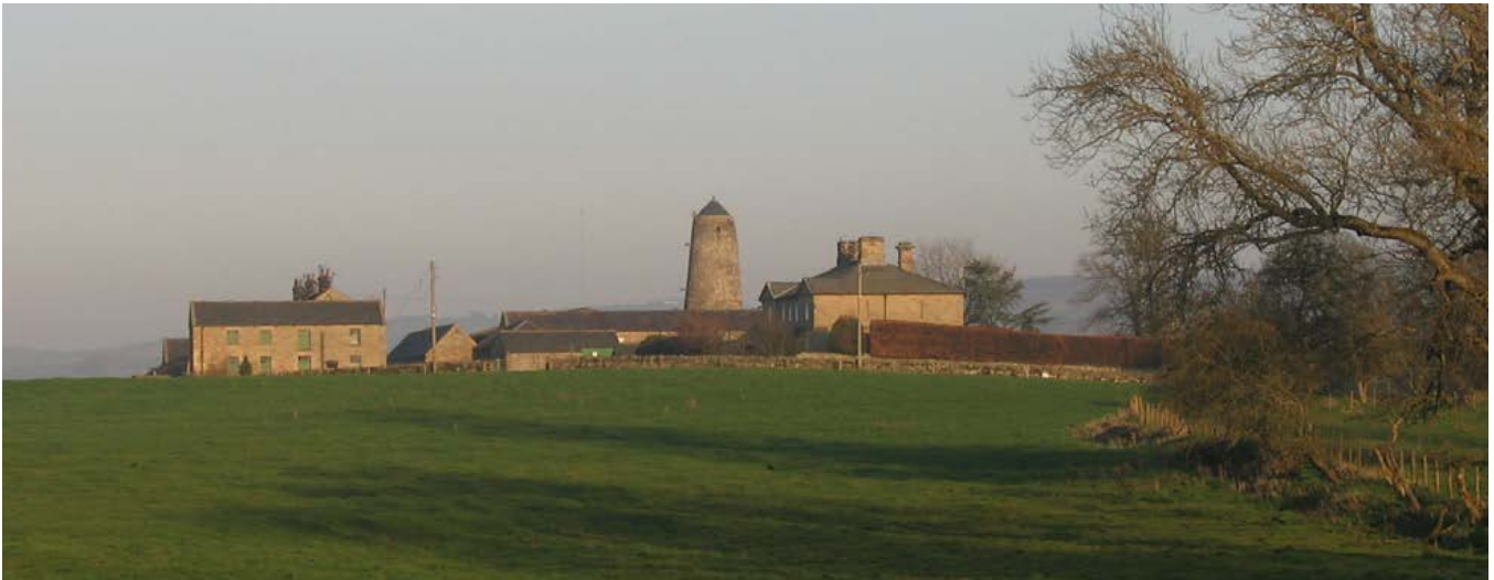
At Chollerton a windmill powered a corn mill and the threshing and feed-processing machinery. Photo © Jeremy Lake
