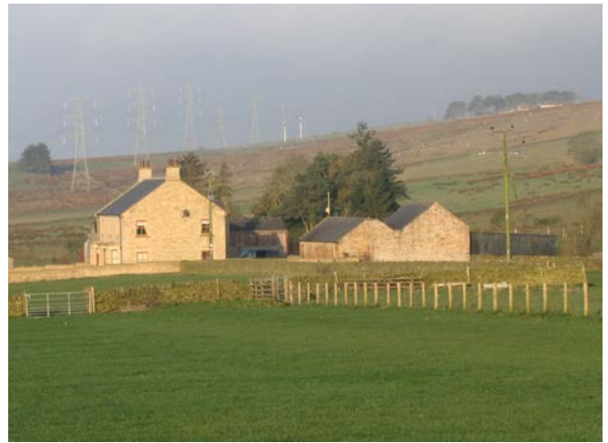
Parallel plans A mid- to late 19th-century, parallel plan farmstead, where the house and working buildings are set in parallel to each other. This arrangement is rarely found, but is typical of the moors. Photo © Jeremy Lake
