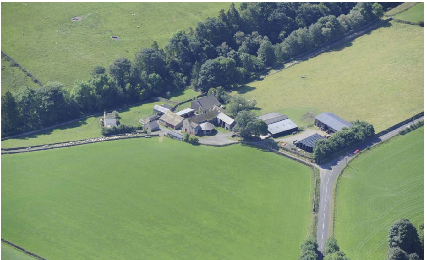
Early to mid-19th-century horse-powered farmstead (note the circular horse gin with the conical roof to house the horse walk for powering the machinery). Photo © Historic England 28559/038
