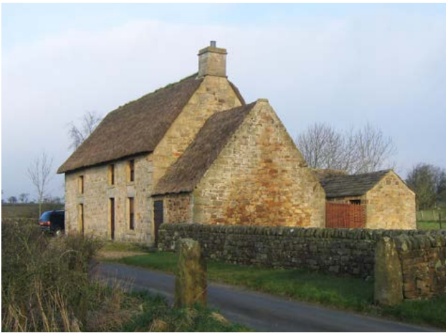
Causeway House, to the west of Vindolanda Fort, is an example of a roadside linear farmstead associated with the enclosure of the moors around Hadrian's Wall. This rare, surviving example of a late 18th-century farmhouse is also notable for its use of heather thatch. Photo © Jeremy Lake
