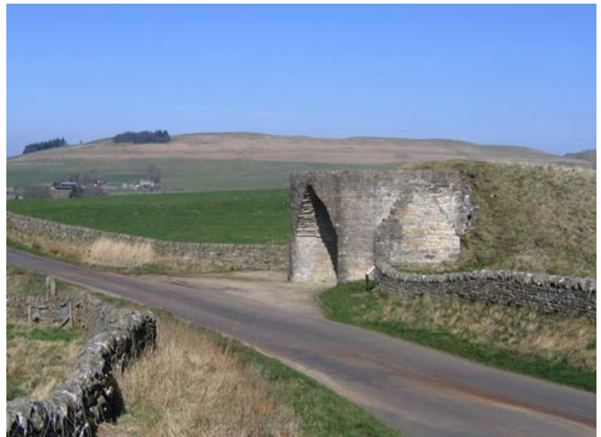
Lime kilns Lime was used to enhance the fertility of the area's more acidic soils, particularly during the years of high input and output in the mid-19th century, when some corn was grown around the moorland fringes. Photo © Jeremy Lake
