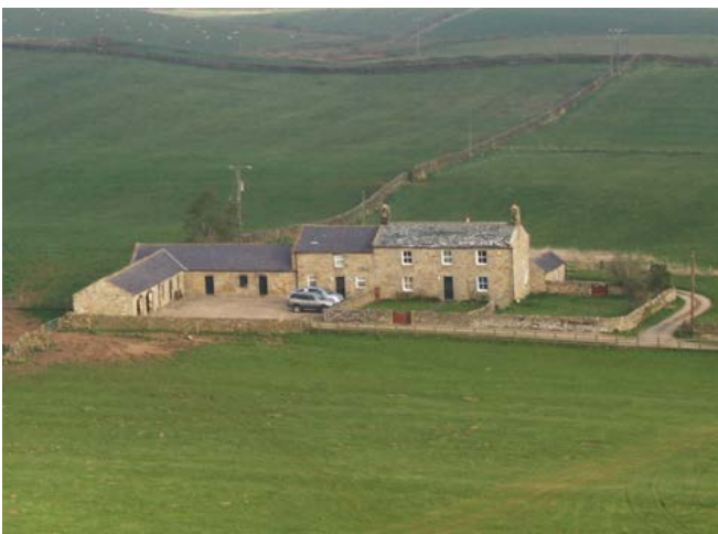
A regular L-plan farmstead of early to mid-19th-century date, just to the north of Hadrian's Wall, the attachment of the house to the working buildings being a typical feature of upland areas. It is set in a landscape of regular enclosure from moorland. Attached to the house is a combined hay barn and stable, and to the left are single-storey calf houses for rearing stock. Photo © Jeremy Lake
