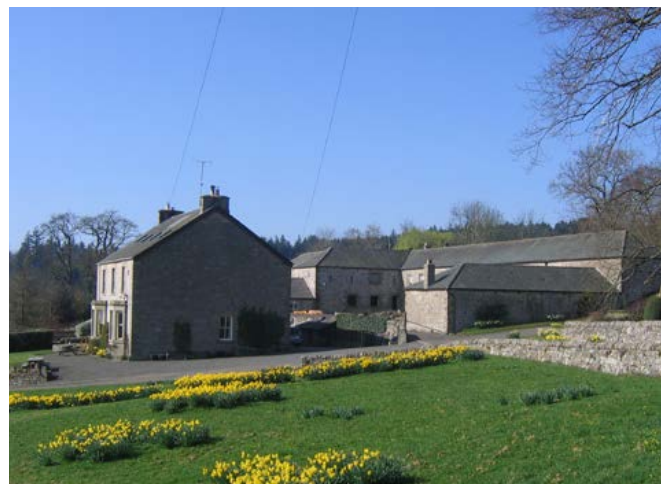
Regular U-plan farmsteads A mid-19th-century, regular U-plan arrangement at Walwick, where by around 1800 several tenements had been absorbed into large farmsteads. The buildings are storeyed and provided hay lofts over stables and cattle housing, with a combination barn built into the rising ground behind. The house faces away from the farmyard, a typical arrangement for more prestigious establishments such as this. Photo © Jeremy Lake
