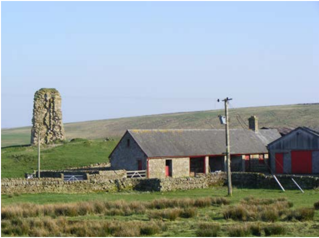
Smithies. A smithy, marked by its chimney stack, is here incorporated into a cart shed range. Photo © Jen Deadman
