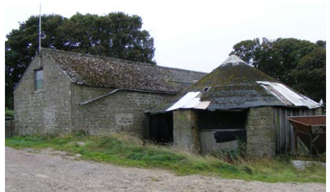
A threshing barn, its doorway enlarged, with a hexagonal wheel house (right) adjoining to the rear. Photo © Jen Deadman
