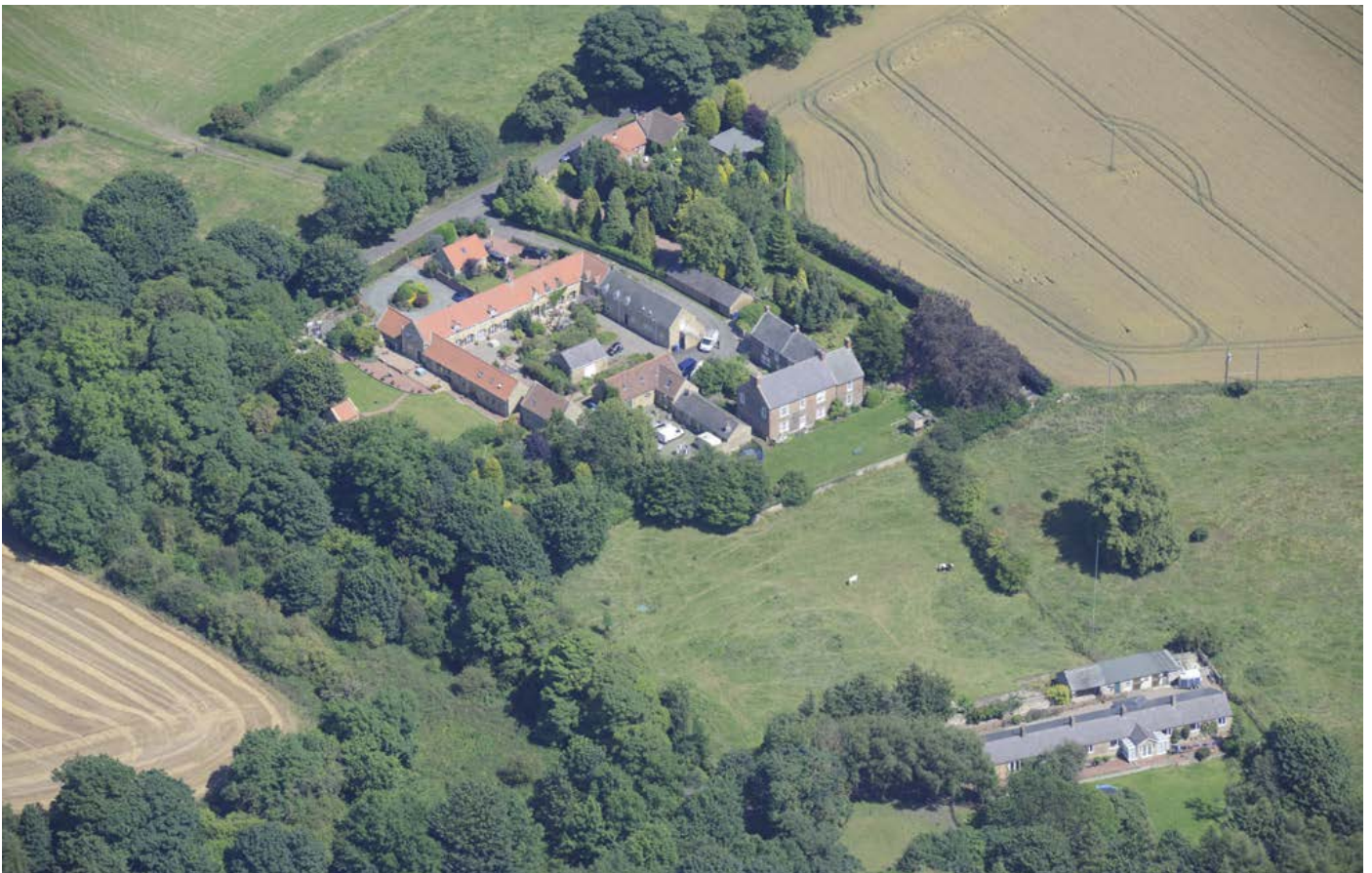
To the east of the above farmstead is Ulgham Grange, which stands on the site of a 12th-century grange of the Cistercian Newminster Abbey. The house and working buildings have fabric dating from the 17th and 18th centuries, but were heightened, extended and replanned in association with the reorganisation of the farmed landscape around it in the early to mid-19th century. Note the row of farmworkers' cottages to the bottom right. Photo © Historic England 28563/022
