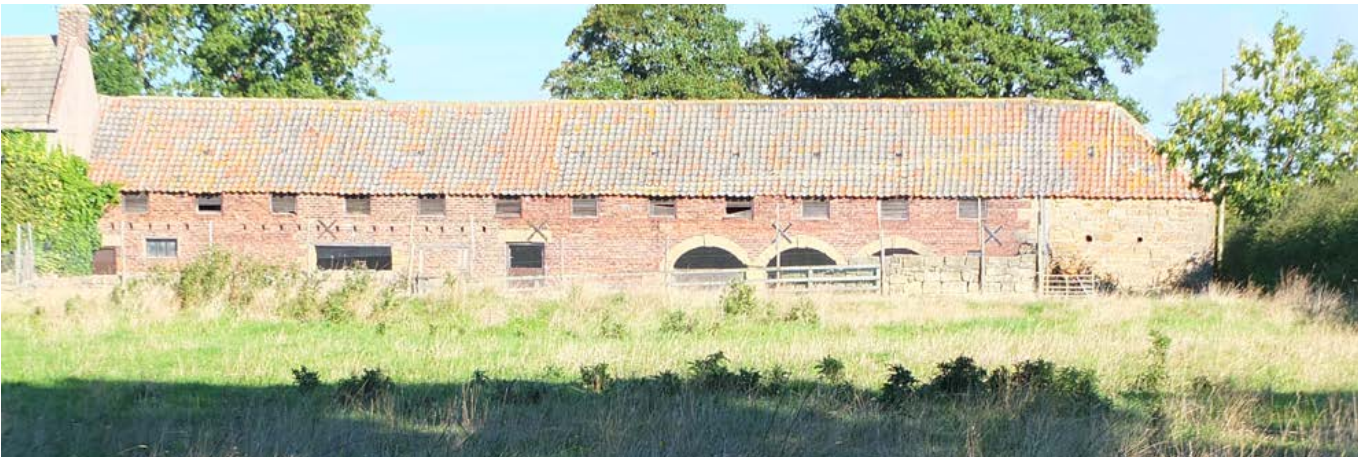
Long, late 18th-century range extending to the east of a farmhouse west of the estate village of Longhirst. It was formerly an L-shaped plan form with two walled yards to the front elevation and a yard area to the rear, beyond which was an orchard. houses stables, a cart shed and shelter sheds – the latter with access to the right-hand yard via an arcade of three arched entries. A full-length granary with 12 slatted windows is set above, approached from the rear by external stone steps. An open-fronted shed formed the east return, but was demolished in the 20th century. The building is of brick on the front elevation with tooled stone dressings to openings, and clearly indicates the scale of arable farming as practised from the late 18th century in this area. Photo © Jen Deadman
