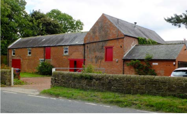
Mid-19th-century, brick-built farmstead, showing a loading door to the first-floor mixing room on the right. Photo © Jen Deadman
