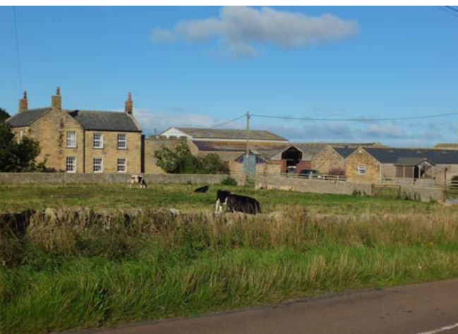
This farmstead at Hemscott on the coastal strip was built in 1840 to a U-shaped plan form with a wheel house and further additions in the late 19th century. The yard comprises linked ranges set to the north-west and east with a wheel house adjoining the west range. Visible on the photograph are two parallel stock sheds. Photo © Jen Deadman
