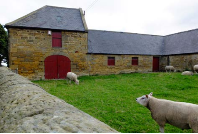
Detail of early 19th-century cart shed/trap house with granary over and adjoining stable range. The use of coursed sandstone with well-defined quoins to corners and openings and roofs of blue slate with stone ridge and copings is characteristic of 18th- and 19th-century farm buildings of the area. Photo © Jen Deadman
