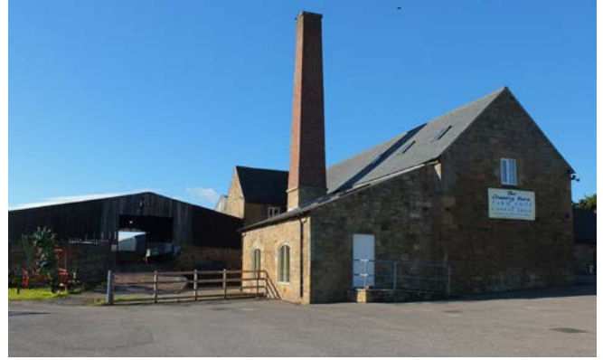
Farm at Widdrington with late 19th-century former steam-engine shed and associated chimney replacing the wheel house. Photo © Jen Deadman
