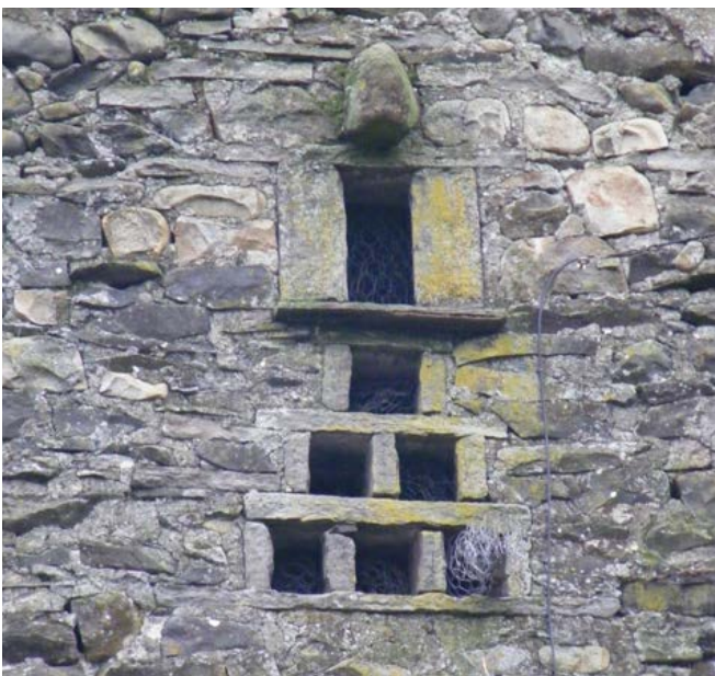
Small, free-standing stable and calf house with loft over. Entrances into yard and field. Planked forking hole has small entrance for hens. Smaller entrance with perching ledge under eaves to left. Photo © Jen Deadman
