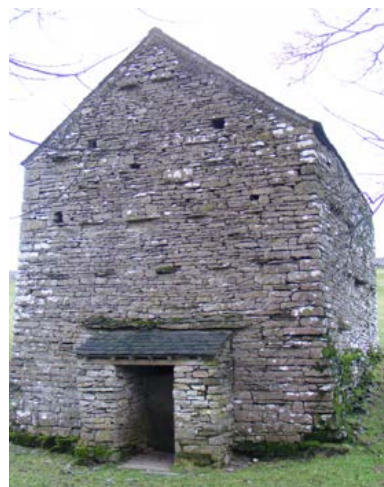
Field barns Small, two-storeyed bank barn with typical small porch, dated 1818. Set close to moor edge and adjacent to drove road leading onto common land. The first-floor joists are of uncut forked branches, and halved timbers form the floor boarding. The stall partitions are of stone slate. Photo © Jen Deadman
