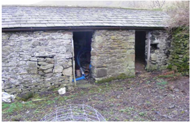
Pig houses Pair of single-storey pig houses with small walled yard. Blocked feeder in wall to left. Photo © Jen Deadman
