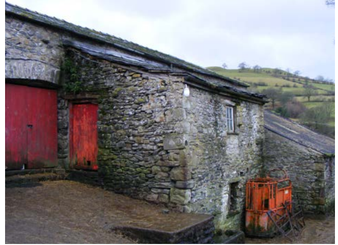
The rear entry accesses the upper floor of the next level, which is for hay storage. Below is another shippon with calf pens in an outshot. Outshots are used to house sheep for husbandry purposes. The sheep dip is situated to the immediate right of the photograph. Photo © Jen Deadman
