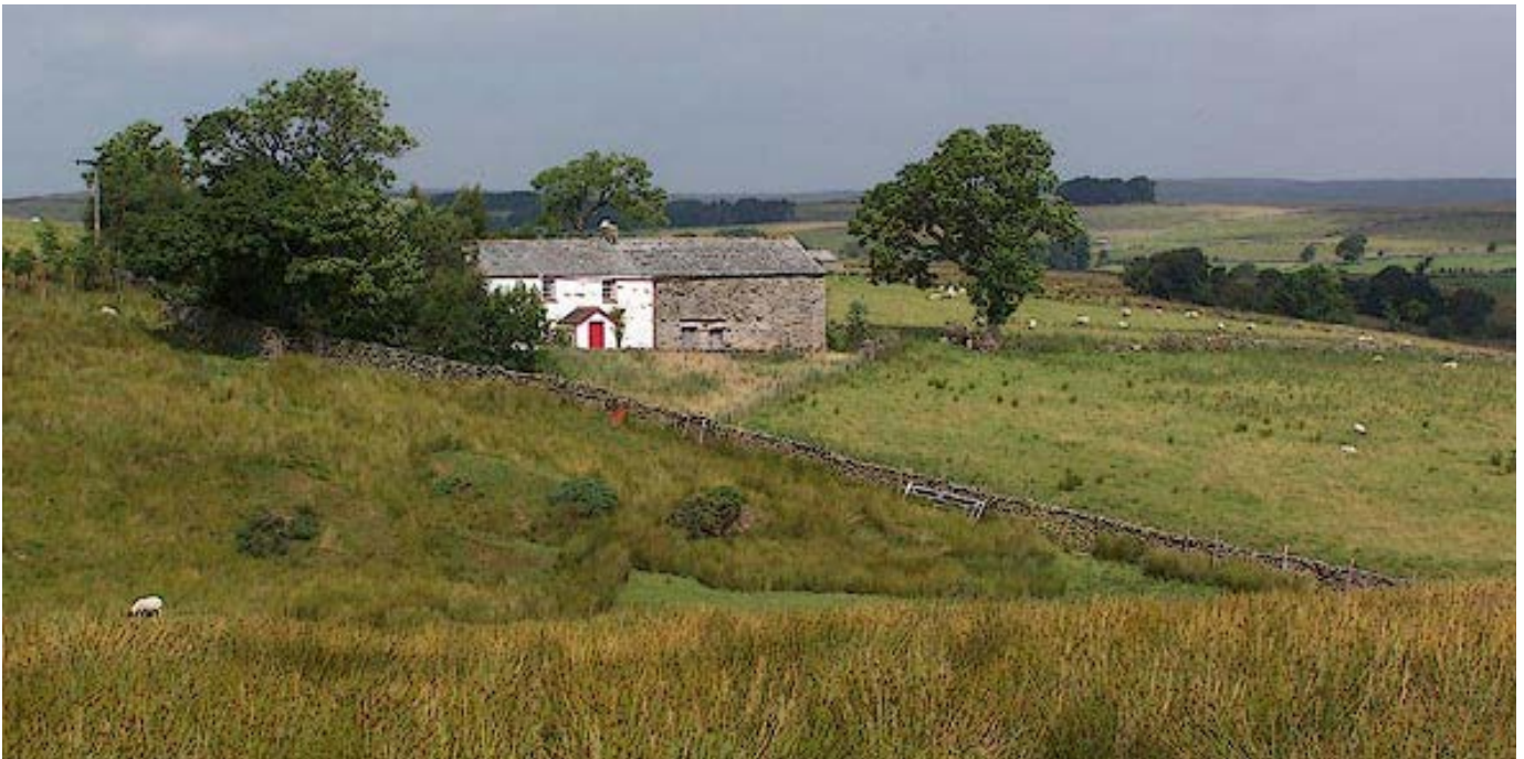
Isolated linear farmstead on the moor edge close to the road connecting Newbiggin-on-Lune with the isolated hamlet of Weasdale. It has a direct link to an old drove road leading off Ravenstonedale common. The linear range comprises a farmhouse and combination barn set in a small, stone-walled enclosure and is of 18th- or 19th-century date. It is set amongst a mix of large and small irregular-shaped fields, hinting at piecemeal enclosure through to the 19th century. Photo © Old Cumbria Gazetteer/J and M Norgate
