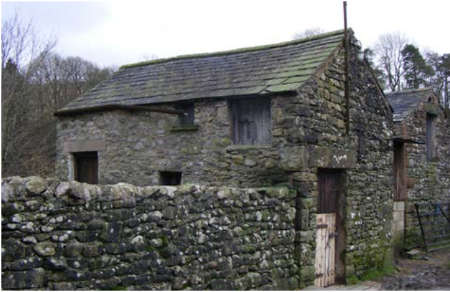
Small, free-standing stable and calf house with loft over. Entrances into yard and field. Planked forking hole has small entrance for hens. Smaller entrance with perching ledge under eaves to left. Photo © Jen Deadman
