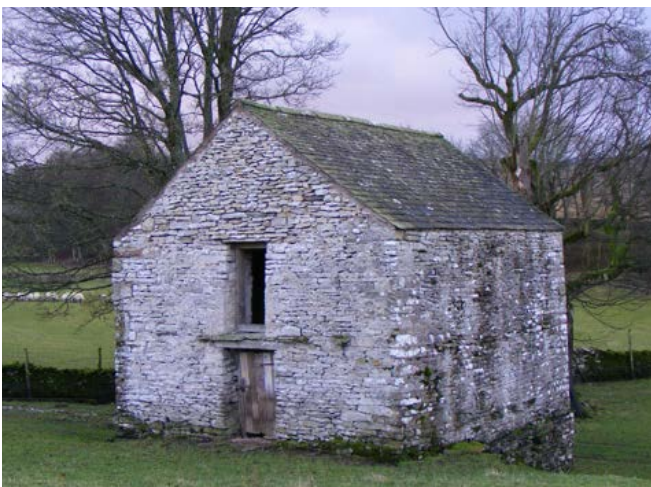
Field barns Small, two-storeyed bank barn with typical small porch, dated 1818. Set close to moor edge and adjacent to drove road leading onto common land. The first-floor joists are of uncut forked branches, and halved timbers form the floor boarding. The stall partitions are of stone slate. Photo © Jen Deadman
