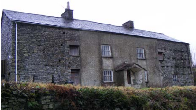
Deserted, isolated, roadside linear farmstead at Firbank, west Howgills. The early to mid-19th-century house is flanked either side by adjoining agricultural buildings, not necessarily of the same phase. Animal housing is located at ground-floor level, with hay lofts above. The rendered house section has long since lost its whitewash. Photo © Jen Deadman
