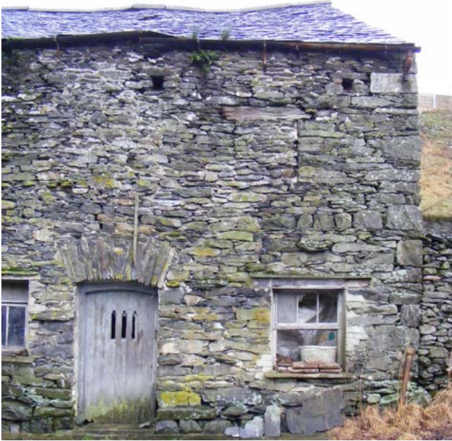
Stables Stable at end of combination bank barn with accommodation for agricultural workers above. Blocked windows evident on front elevation and gable end. Photo © Jen Deadman
