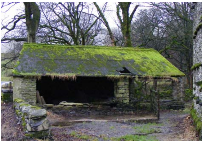
Cart sheds or cart standings are frequently incorporated into the barn, singly rather than as a series of open fronted bays as seen in lower lying areas. This is a stand-alone example. Photo © Jen Deadman
