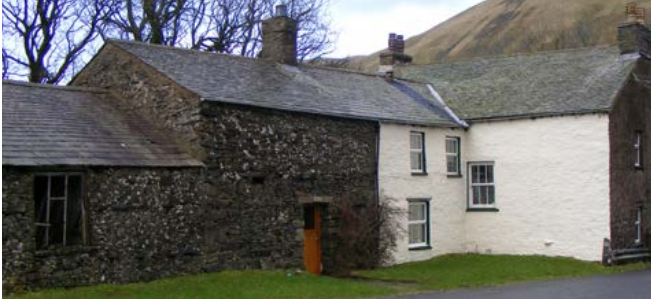
Linear plans. Working farm situated in the Lune valley on the west side of the Howgills. Here, the rear wing represents the oldest phase of the building. Originally single-storey (indicated by dotted line), it was raised and subsequently fronted by a new farmhouse added to the gable at right angles – probably in the 18th century. Photo © Jen Deadman
