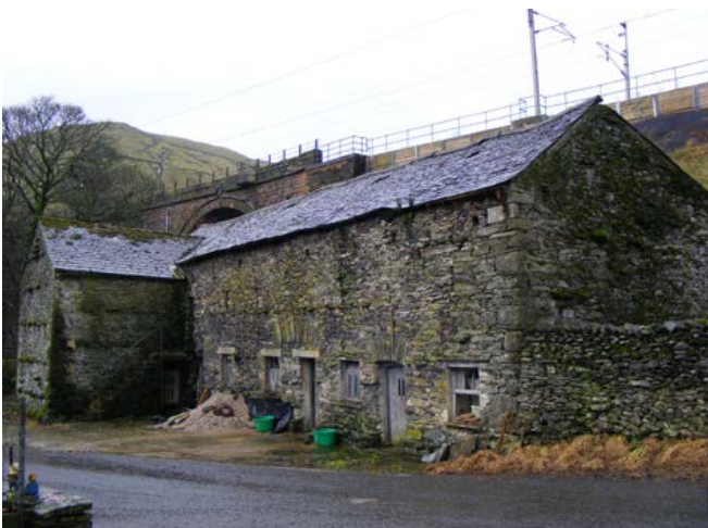
Bank barns Large bank barn of eight bays comprising cow house and stable with full-length loft over, in the west of the Lune valley. Access to the loft is via two large wagon entries at the rear. Photo © Jen Deadman
