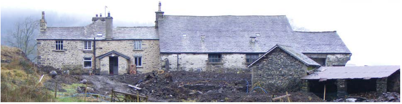
Linear plans Linear or L-shaped farmsteads, where the house and working buildings are attached and in line, are common farmstead types. This example in Staveley-in-Cartmel comprises a farmhouse and large combination barn in line. The farmhouse, much altered, looks out over a small yard area with small ancillary buildings on the perimeter. Photo © Jen Deadman
