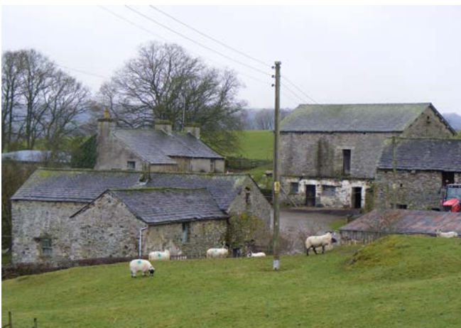
Courtyard plans The loose courtyard plan, where working buildings are arranged around one or more yards for cattle is common to the area. Here the buildings, dominated by the large bank barn, are set around three sides of the yard. Photo © Jen Deadman
