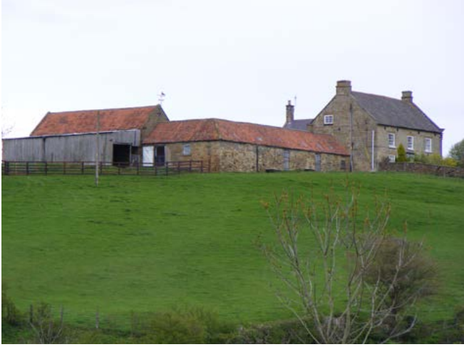
Isolated hilltop farmstead outside Boltby, in the south-east of the area. Immediately to the east lies the long swathe of Boltby Forest and the escarpment marking the edge of the Hambleton Hills. Brick gives way to sandstone as the predominant building material. Photo © Jen Deadman
