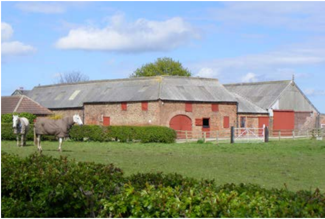
L-shaped combination barn occupying a corner plot on planned, 19th-century farmstead, providing animal housing, hay and fodder storage. Photo © Jen Deadman
