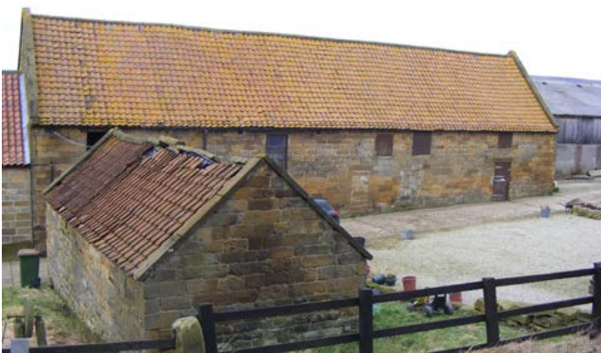
Large, late 18th- or early 19th-century combination barn at Great Fryup Dale, with hay loft and granary above threshing floor and stabling. The single-storey attached building is a cow house. Photo © Jen Deadman
