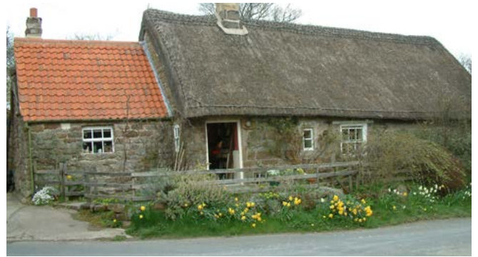
Former longhouse at Egton in the northern dales. The byre to the left of the cross passage was replaced with a small service room. Photo © Jen Deadman
