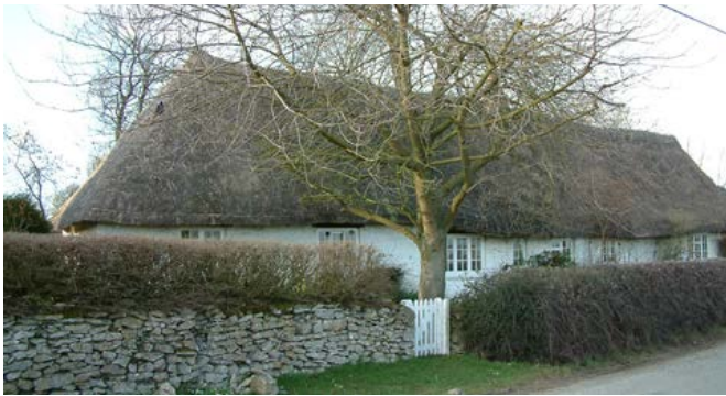
Longhouses Former longhouse at Pockley in the southern dales. Pockley has longhouses, many dating from the 17th century, which were conserved through residential and small-scale agricultural use when the estate invested in the rebuilding of farmsteads to serve larger improved farms. The cross passage lay behind the stack, with the byre for cattle beyond. Here, an extra bay was added later. Each bay was defined by a cruck-frame. Photo © Jen Deadman
