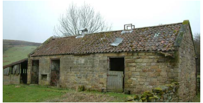
Single-storey ranges which incorporate pigsties and calf houses are common. The feed chute, evident in the wall, is a feature common to pigsties in this area. Photo © Jen Deadman
