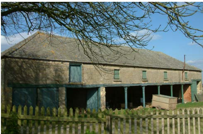
Only the larger farms have cart sheds of more than three bays. Griff Farm, Rievaulx, has possibly the largest in the area, with six open bays supported by six cast iron columns, as well as two closed bays at one end and one at the other. It was built after 1850 and stands outside and apart from the two yards. Photo © Jen Deadman
