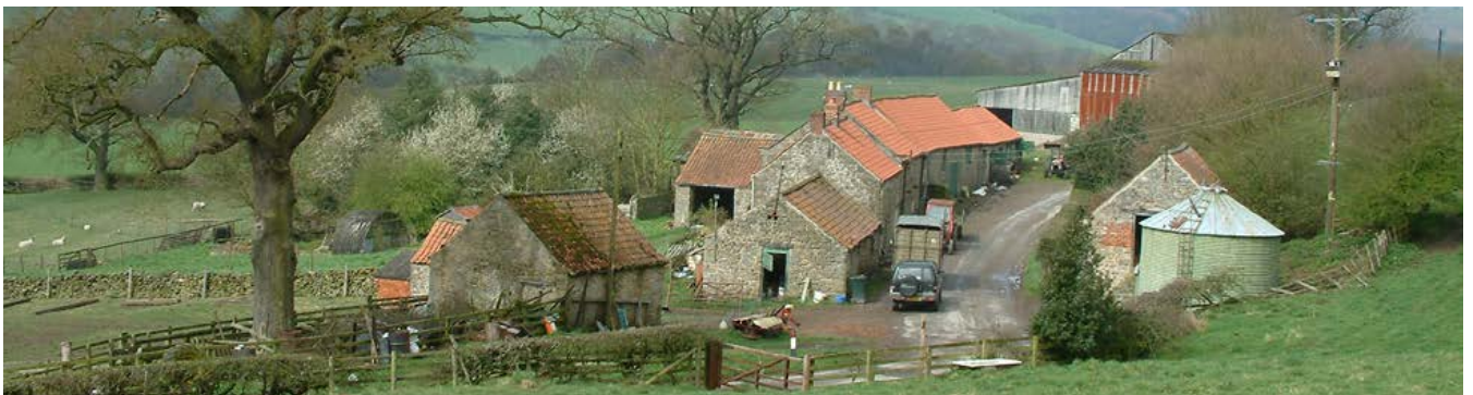
Isolated steading set along the roadside in Fadmoor in the southern dales. The farmhouse and attached barn with wheelhouse form the major elements in the long, linear range. The stepped appearance of the roof-lines is a characteristic feature of the North York Moors. It faces a routeway which also relates to a scatter of associated working buildings. The farmhouse is stylistically late 18th- or early 19th-century and possibly replaces an earlier building. The steading is set amongst small irregular fields of piecemeal enclosure towards the valley bottom. Photo © Jen Deadman
