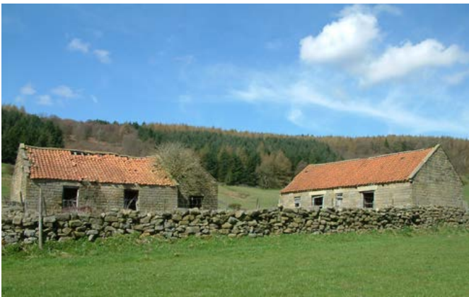
Field barns and outfarms An outfarm in Bilsdale with provision for cattle housing in three buildings. Photo © Jen Deadman
