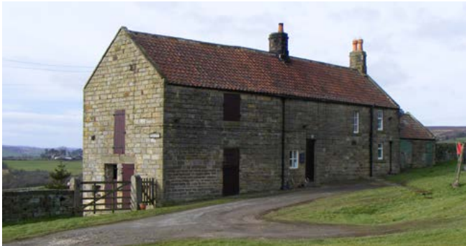
Linear plans Lealholm, at Eskdale in the northern dales. This small farmstead or smallholding, which adjoins common moorland in the foreground, was built in the mid-19th century. This range comprises a cow house with loft over and pigsty in the gable end, the farmhouse and a single-storey stable. Photo © Jen Deadman
