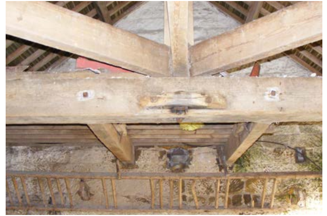
Here, the main cross beam to which the revolving central shaft was attached and the support beams remain in situ. Photo © Jen Deadman
