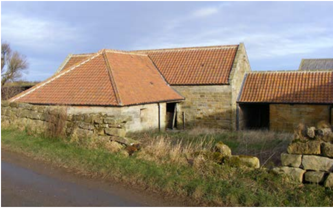
Horse engine houses are associated with barns where corn was threshed, machinery for mixing fodder was located, and straw was stored. Photo © Jen Deadman
