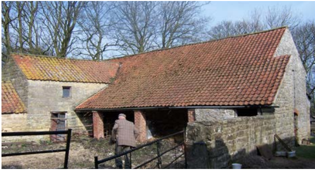
Cow houses An open-fronted shelter shed for cattle opening onto a yard and built in the angle of an L-shaped range. Photo © Jen Deadman
