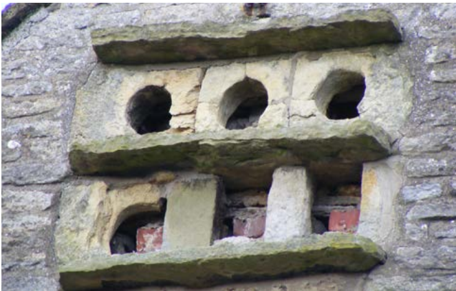
Entries to pigeon loft in gable end of farmhouse. Photo © Jen Deadman
