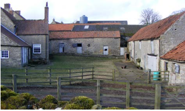
Courtyard plans Farmstead occupying corner site in Lockton village, with farmhouse fronting a yard arrangement which includes combination barn, dairy, pigsties and stables. Photo © Jen Deadman
