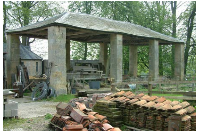
Hay barn An early 19th century hay barn with stone piers, at Duncombe Park, Helmsley. Photo © Jen Deadman
