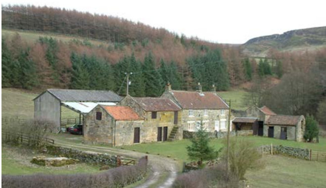
L-shaped plans The house, built in the early to mid-19th century, is an integral part of this L-shaped group. Adjoining is a barn with loft over, stable and cow house. Photo © Jen Deadman
