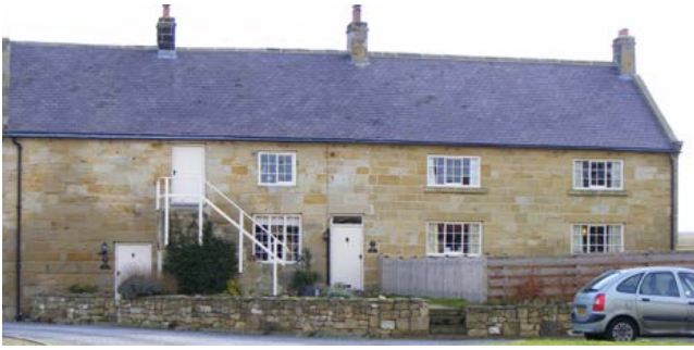
Ellerby village in the northern dales. Granary over stable adjoining farmhouse. The access is via stone steps on the front elevation. Photo © Jen Deadman
