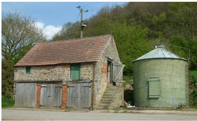
Granaries are commonly located above cart sheds, as here at Fadmoor. Known to exist by 1827, the granary probably replaced one in the farmstead attic. It sits adjacent to the roadside and forms part of a dispersed plan farmstead. Photo © Jen Deadman
