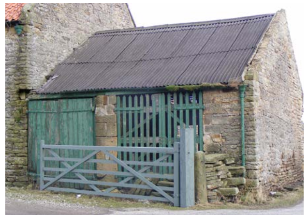
Single-storey, two-bay cart shed attached to large combination barn (at Sneaton in the southern dales), a common arrangement evident throughout the area. Photo © Jen Deadman
