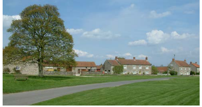
Fadmoor village, one of several planned linear settlements situated in the lower southern belt. Substantial courtyard farmsteads are set around a wide, linear green. Strip fields lie behind the steadings, bounded east and west by deciduous and conifer plantations. Photo © Jen Deadman
