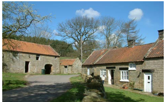
Dispersed plans Laskill Pasture in the southern dales. This dispersed-plan steading straddles the roadside. The working buildings and yard, dated 1846, are sited opposite the farmhouse, which developed from a cruck-framed longhouse, and attached working buildings. Photo © Jen Deadman
