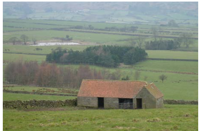
Field barn for cattle at Danby, incorporating a cart shed for taking manure to the surrounding fields. Photo © Jen Deadman
