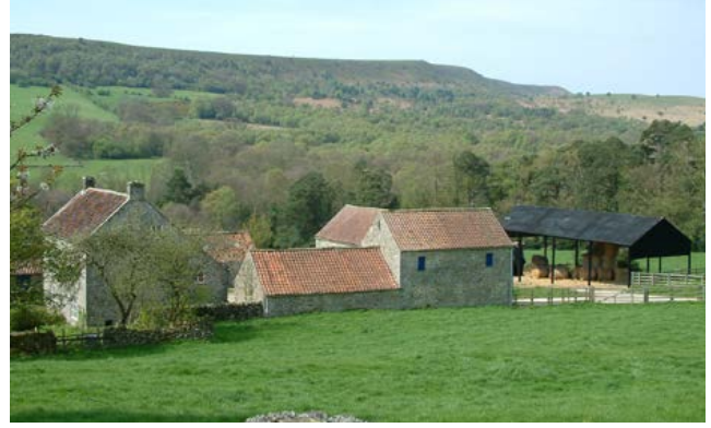
Isolated farmstead at Fadmoor in the southern dales. This is a loose courtyard arrangement, with detached working buildings planned around three sides of the yard. Photo © Jen Deadman
