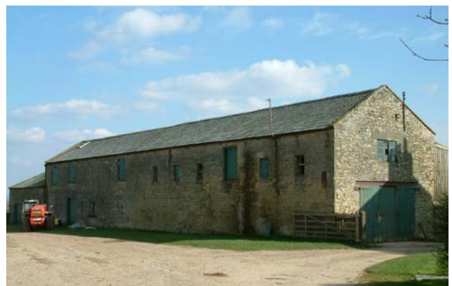
Griff Farm, at Rievaulx in the southern dales, formerly the home farm of Duncombe Park Estate. This very large combination barn, in its scale similar to those found on the estate farms of the Howardian Hills and Yorkshire Wolds, provides threshing barn, stables and loose box with granaries over. Adjoining to the west is a single-storey cart shed accessed from the gable end. A horse engine house formerly adjoined the building on the yard side. Photo © Jen Deadman
