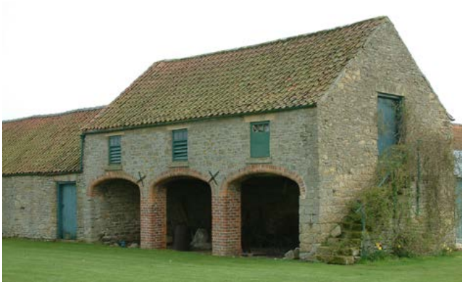
The size of granaries over cart sheds (left) or stables (right) illustrates the importance of arable-based farming from the late 18th century. Note the louvred windows for ventilation Photo © Jen Deadman
