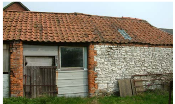
The date and number of cart sheds also illustrate the development of arable-based farming, smaller carts being needed to take farmyard manure to the fields. This small cart shed has pegged oak roof trusses, rarely used after the 1840s and predating the common use of softwood. Two bays are set on the long elevation, with a third, its entry widened, accessed from the gable end. Photo © Jen Deadman
