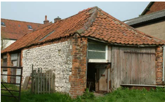
The date and number of cart sheds also illustrate the development of arable-based farming, smaller carts being needed to take farmyard manure to the fields. This small cart shed has pegged oak roof trusses, rarely used after the 1840s and predating the common use of softwood. Two bays are set on the long elevation, with a third, its entry widened, accessed from the gable end. Photo © Jen Deadman
