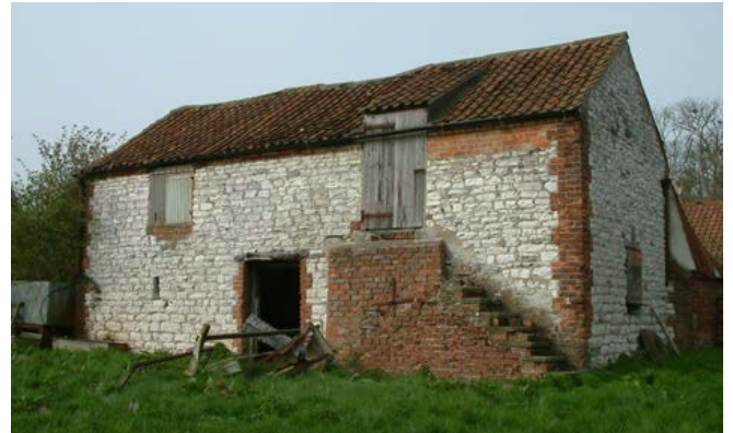
The size of granaries over cart sheds (left) or stables (right) illustrates the importance of arable-based farming from the late 18th century. Note the louvred windows for ventilation Photo © Jen Deadman
