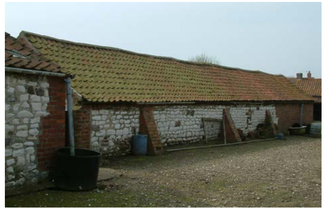
Chalk walling to an 18th-century building, extended in 19th-century brick. Photo © Jen Deadman
