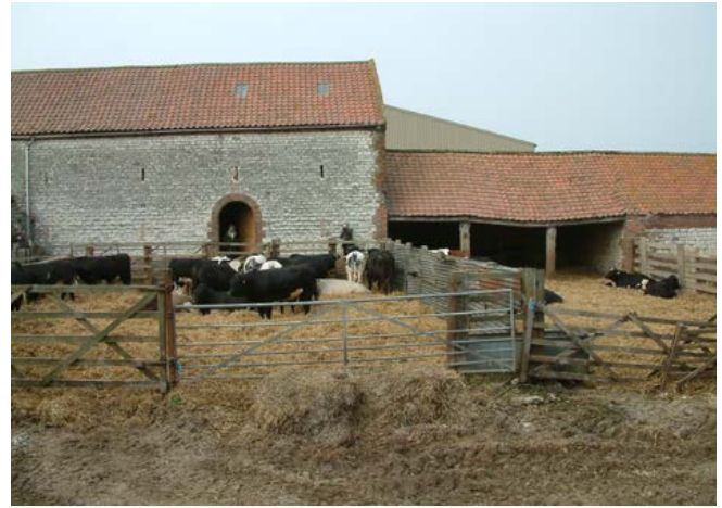
Part of a large barn at Burton Fleming. Its roof was raised in 1823, and, as with many barns in this and surrounding areas, the threshing floor has opposing winnowing doors that are too narrow to admit carts for unloading the harvested drop. Photo © Jen Deadman
