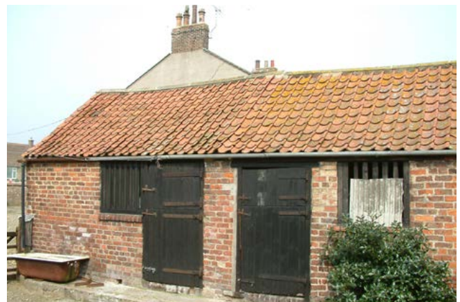
Two loose boxes with doors and slatted windows to aid ventilation. Photo © Jen Deadman
