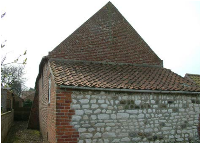
Tumbled-in brickwork to gable ends is a typical feature of this area and continues as a tradition into northern East Anglia. Photo © Jen Deadman
