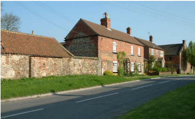
This village farmstead has a lower, steeply pitched roofline in its present gable, built of cobbles with brick levelling courses. The change in brickwork on the front elevation would suggest it was single storey originally. Photo © Jen Deadman
