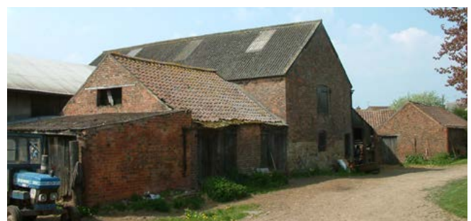
The stone walling remaining on the lower courses of this mid-19th-century combination barn shows that it has earlier origins, prior to its rebuilding and incorporation into a courtyard with cart sheds (in the foreground) facing the access track. Photo © Jen Deadman
