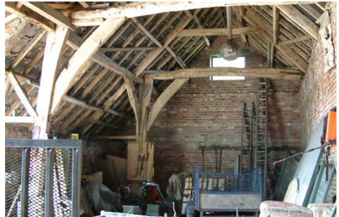
Timber-framed barns of the 17th century and earlier, often aisled as here, were commonly reclad or their walls mostly replaced by brick and cobble in the 18th and 19th centuries. This barn was originally aisled on both sides. Photos © Jen Deadman
