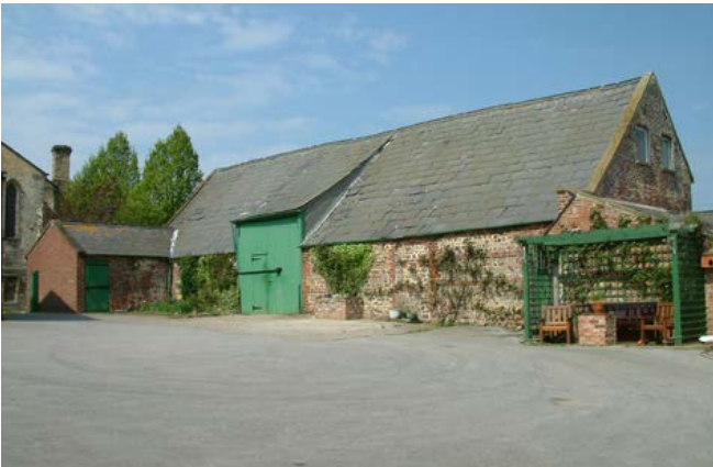
Timber-framed barns of the 17th century and earlier, often aisled as here, were commonly reclad or their walls mostly replaced by brick and cobble in the 18th and 19th centuries. This barn was originally aisled on both sides. Photos © Jen Deadman
