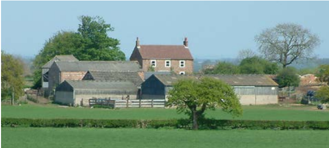
Most farmsteads sited away from villages date from after the mid-18th century, and are viewed across fields bounded by low thorn hedges. To the left is a typical mid-19th-century farmstead, to the east of Knaresborough, with a large combination barn of cobble and brick construction. To the right is a brick-built courtyard group of the early 19th century, including a combination barn (with integral stables) and a pyramidal-roofed dovecote to the left. Photos © Jen Deadman
