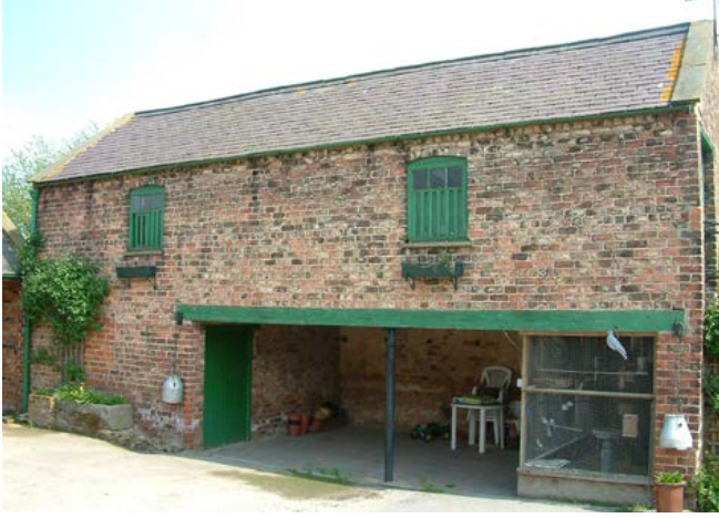
The brick-built granary over an open-fronted cart shed is common to farmsteads in this area of mixed pastoral and arable farming. Note the cast-iron column and the louvred windows to ventilate the grain. Photo © Jen Deadman
