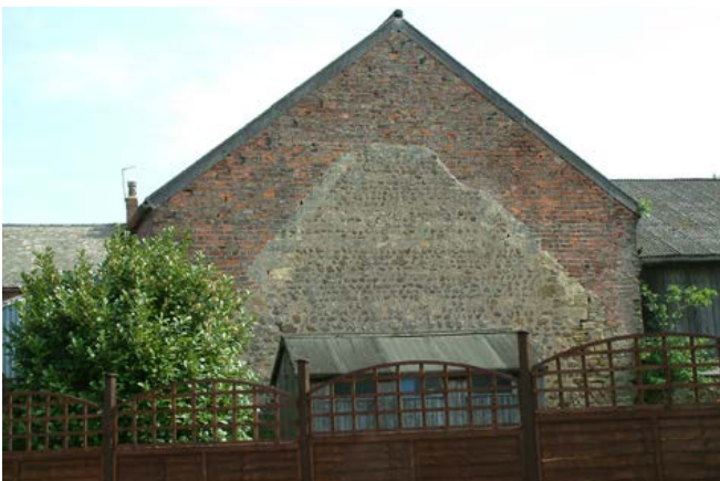
The pitch of this earlier stone walling suggests the presence of a thatched, single-storey building. Photo © Jen Deadman
