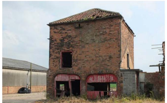
An early 19th-century dovecote on a large farmstead with two-bay cart shed below. The nesting boxes are of brick. A drive shaft and belt in the cart shed would suggest a secondary function for the latter such as a turnip house with motive power sourced from the now derelict adjoining building. Photo © Jen Deadman
