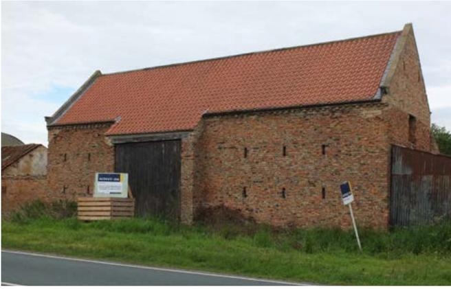
Barn, part of small yard complex in village setting. Dated 1839 as evidenced on tie bar ends. Note the arched taking-in doors and diamond-shaped air vents. Photo © Jen Deadman
