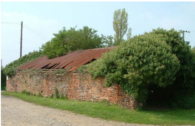
Corrugated iron was used as a cheaper roofing material from the late 19th century. Photo © Jen Deadman
