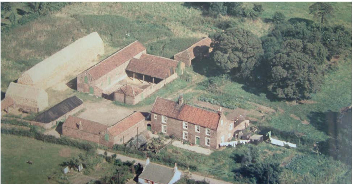
Regular multi yard steading on the outskirts of Old Ellerby. The aerial photo of 1963 shows a well-organised farmstead with late 18th- or early 19th-century buildings arranged around two yards. To the north, an enclosed walled yard is flanked on one side by a large combination barn – the largest agricultural building in the complex. Adjoining shelter sheds allow cattle free range within the yard, in the lower corner of which is a meal house. Beyond to the north is a range of open-fronted cart sheds.
