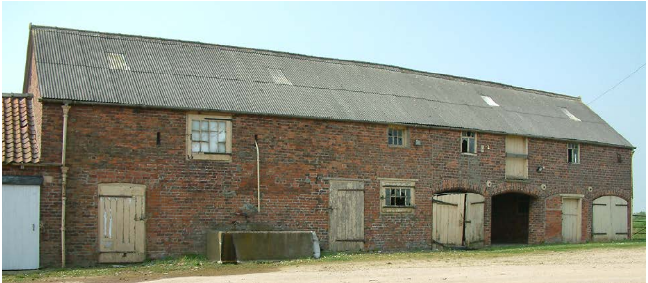
The combination barn, frequently the largest agricultural building on the farm, is multifunctional. This large barn has provision for four cart bays (one blocked) stabling and tack room for saddles and harness at ground floor level, with a hay loft and granary over. The traditional pantile roof has been replaced. Photo © Jen Deadman
