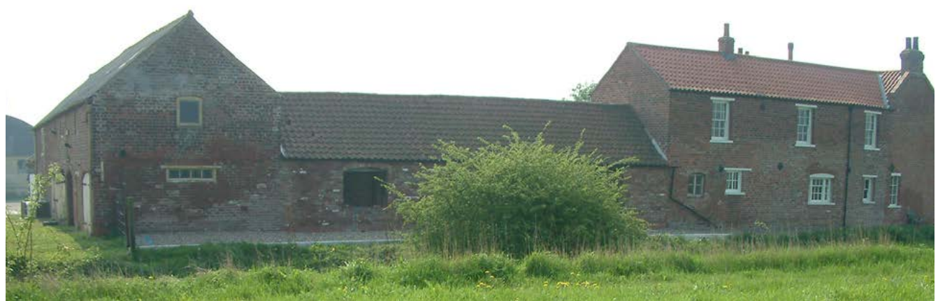
Regular L-plan ranges attached to farmhouses are a distinctive characteristic of smaller-scale farmsteads, with combination barns (here including a granary over two cart bays) attached to single-storey cattle housing. Photo © Jen Deadman
