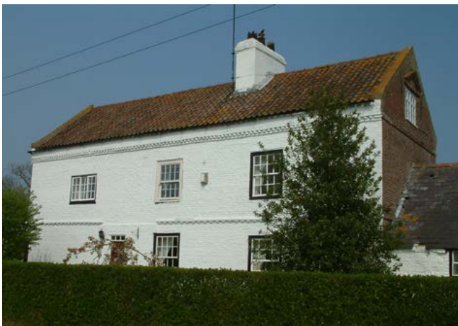
Fine, early 18th-century high status farmhouse with coggled and dentilled course at eaves level – a decorative feature common to all Yorkshire lowland areas. Note the decorative brick pediment to the attic window. The ancillary building adjoining the farmhouse comprises courses of diagonally laid cobbles. Towards the coast, cobble is frequently used as a building material. Photo © Jen Deadman
