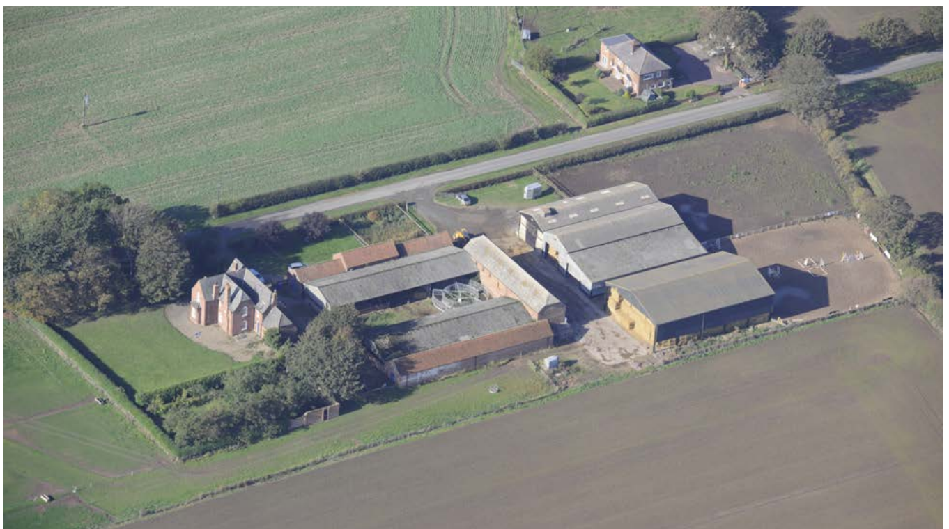
This is one of the farmsteads on the Crown estate of Sunk Island, built to the designs of Samuel Sanders Teulon, an architect better known for his robust Gothic Revival churches. Note the detached house with its garden, the regular layout of detached buildings set around three sides of a cattle yard and the two-storey mixing barn range to the right, which would have processed crops taken from the rick yard (now with modern sheds) and mixed roots and other feed for livestock; external steps offer access to the granary over a cart shed range. Photo © Historic England 28480/002
