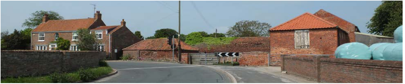
An early to mid-19th-century roadside grouping, showing the use of brick and pantiles typical of this period. Photo © Jen Deadman
