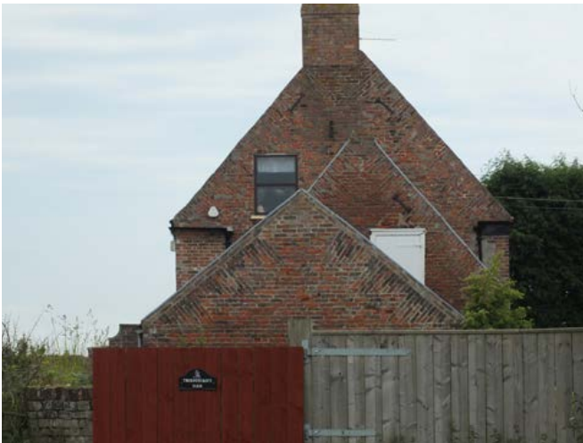
Many gable ends display the traditional tumbled eaves common to the area on 18th- and early 19th-century domestic and agricultural buildings. Photo © Jen Deadman
