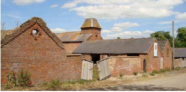
Manor Farm, Kirmond le Mire, is a very well preserved example of a planned model farmstead of the mid-19th century. The single phase of brick and slate construction sets it apart from the more organically developed and expanded farmsteads nearby. The rigorous planning of this farmstead makes it difficult to find appropriate agricultural uses in the present day. Photo © Locus Consultants
