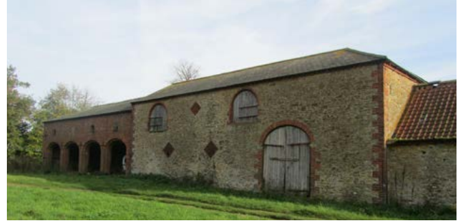
This outfarm on the Haxby estate was built in stages, reflecting the increased capacity required for arable-based farms in the 19th century. To the right is an early 19th-century threshing barn, and on the left a large, later brick granary sited over a four-bay cart shed. To the rear, facing east, are remnants of stock-fattening sheds. Photo © Locus Consultants
