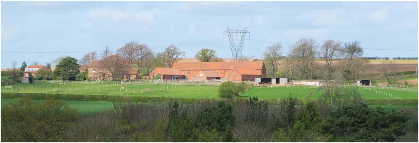
Outlying farmsteads, such as this group of c 1840 with its detached farmhouse and E-shaped regular courtyard layout, usually result from the resiting of farmsteads amongst fields enclosed by the early 19th century; this often occurred some decades after enclosure, after farms had continued to exchange and amalgamate their land. Photo © Jen Deadman
