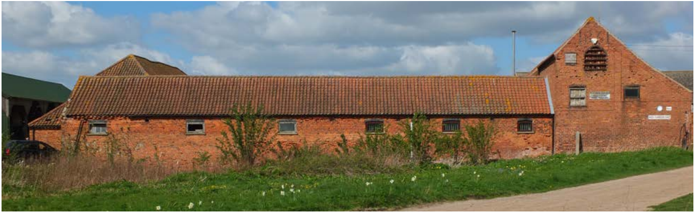
A regular courtyard plan farmstead in the north of the area. It comprises linked ranges set around two unconnected yards. Buildings are of brick with pantiled roofs. A date of 1832 is picked out in black headers on the gable end of the combination barn, which incorporates stables and is attached to a single-storey cow house. Photo © Jen Deadman
