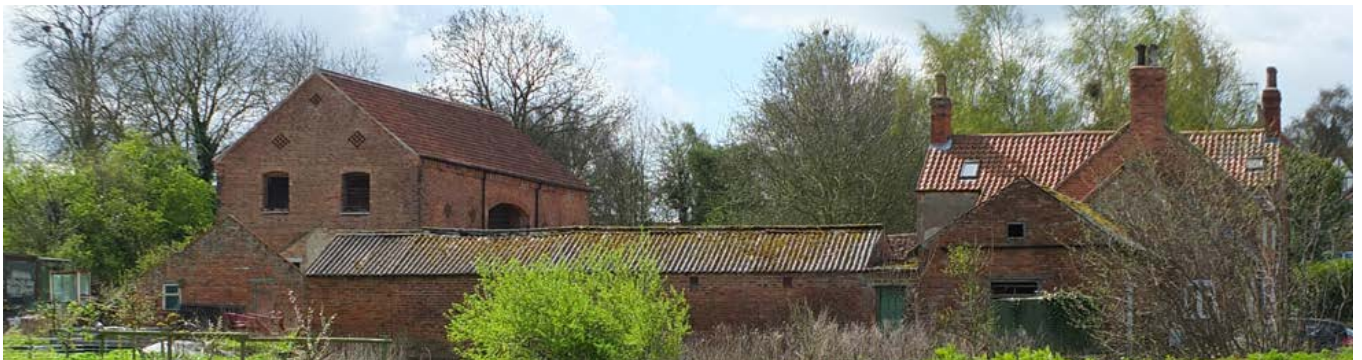
A regular courtyard plan farmstead in the north of the area. It comprises linked ranges set around two unconnected yards. Buildings are of brick with pantiled roofs. A date of 1832 is picked out in black headers on the gable end of the combination barn, which incorporates stables and is attached to a single-storey cow house. Photo © Jen Deadman
