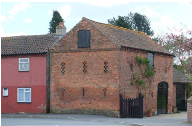
Asymmetrical barns, such as this example of c 1840 to the left and the early 19th-century example to the right, illustrate the need to store less straw after threshing, as it was taken straight to the cattle yards. The offset cart entry to the left with a smaller, opposed winnowing door opens onto the threshing bay. To the left is a former byre with a loft over open to the threshing floor, above which is a hay loft. This building has a profusion of narrow vents to all elevations. Photos © Jen Deadman
