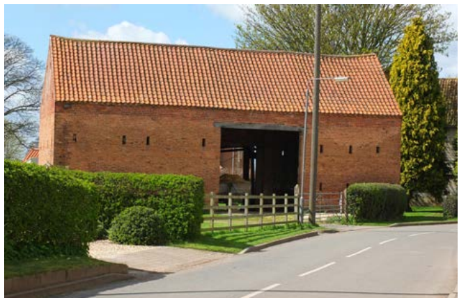
Asymmetrical barns, such as this example of c 1840 to the left and the early 19th-century example to the right, illustrate the need to store less straw after threshing, as it was taken straight to the cattle yards. The offset cart entry to the left with a smaller, opposed winnowing door opens onto the threshing bay. To the left is a former byre with a loft over open to the threshing floor, above which is a hay loft. This building has a profusion of narrow vents to all elevations. Photos © Jen Deadman
