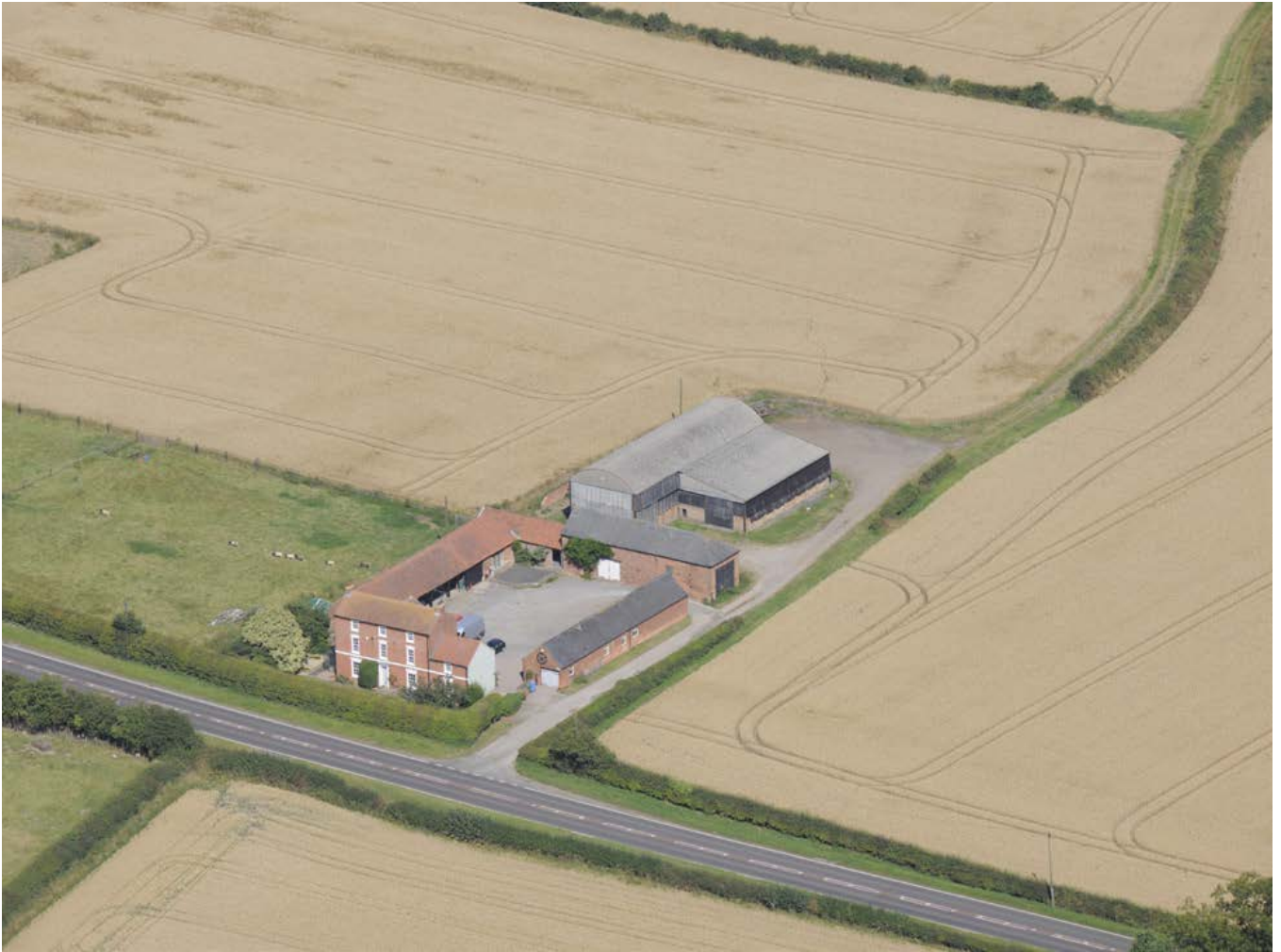
An early 19th-century regular courtyard farmstead with a threshing barn, shelter shed, stables and cart shed at Ragnall, one of the boundaries retaining the curved form of a medieval strip field. The Late Georgian style of the house, with its smaller windows to servants' accommodation on the upper floor, is typical of this area.
