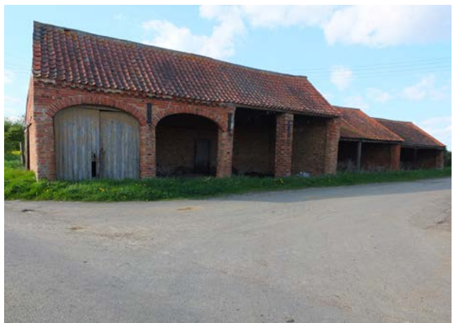
Successive additions to this early 19th-century cart shed, with doors to the left-hand implement shed, illustrate the growing size and capacity of arable-based farms in this area in the 19th century. Photo © Jen Deadman
