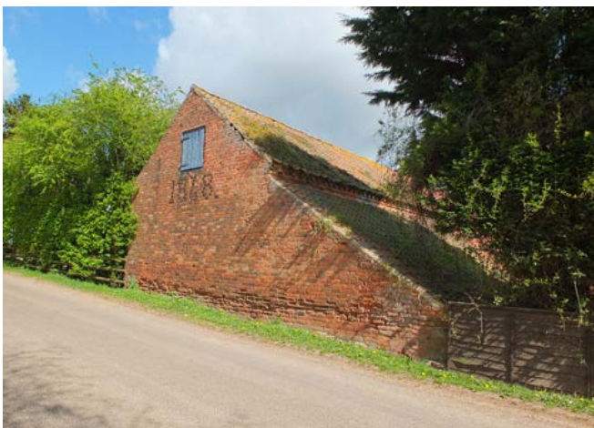
A large combination barn with integral outshot and deep, catslide roof. The barn is dated 1868 and has fine dentilled moulding to the eaves. Photo © Jen Deadman
