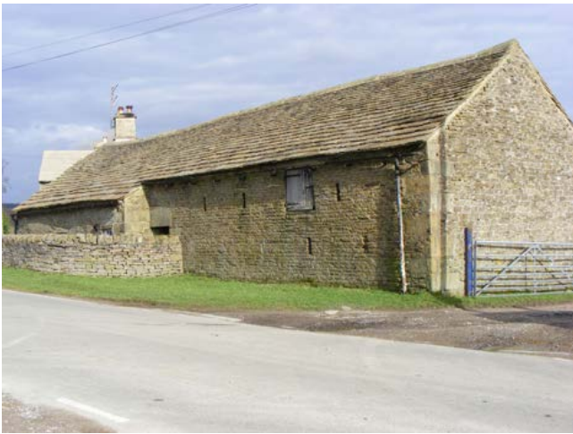
Roadside combination barn, with outshot forming the return of an L-shaped plan form. The farmhouse lies apart. The outshot is not as common to the area as in other parts of the Peak. It frequently houses a stable or sometimes acts as a cart shed. Photos © Jen Deadman
