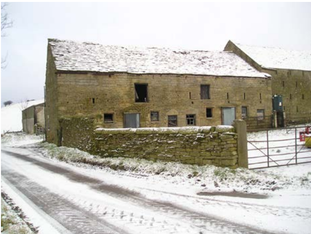
Highlow Hall barn near Hathersage. 17th-century combination barn with hayloft above cattle housing. The eaves line was originally lower, as there is evidence for raising to its present height. The front elevation is punctuated with entries, the shape of the massive lintels being a characteristic feature of 17th-century buildings in the area. Photos © Peak Park
