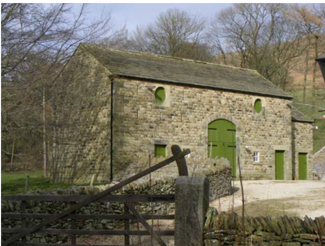
Combination barn The high cart-entry to this mid-19th-century building is flanked by two cattle entries leading to lofted byres. Unusually, the pitching holes are circular, possibly indicating an estate building. Narrow vents pierce the upper walls to provide ventilation to the hay lofts. Photo © Jen Deadman
