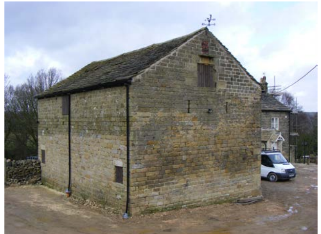
Cow house Simple, two-storey mid-19th-century cow house comprising a hay loft over byres which complements the threshing barn to which it adjoins at right angles. There is no access between the two. Photo © Jen Deadman
