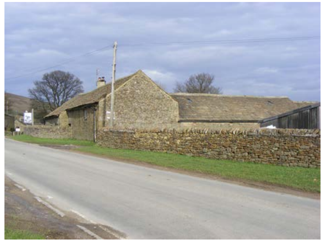
Roadside combination barn, with outshot forming the return of an L-shaped plan form. The farmhouse lies apart. The outshot is not as common to the area as in other parts of the Peak. It frequently houses a stable or sometimes acts as a cart shed. Photos © Jen Deadman
