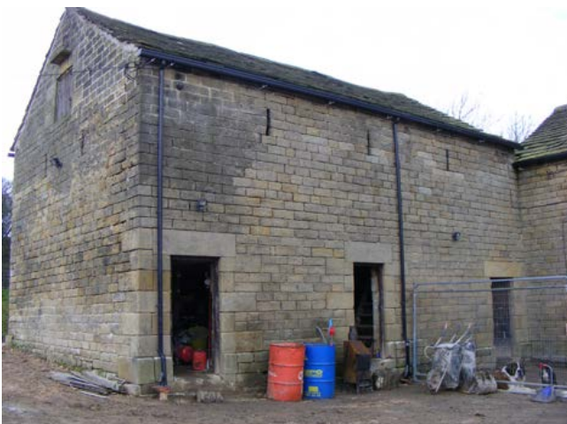
Cow house Simple, two-storey mid-19th-century cow house comprising a hay loft over byres which complements the threshing barn to which it adjoins at right angles. There is no access between the two. Photo © Jen Deadman
