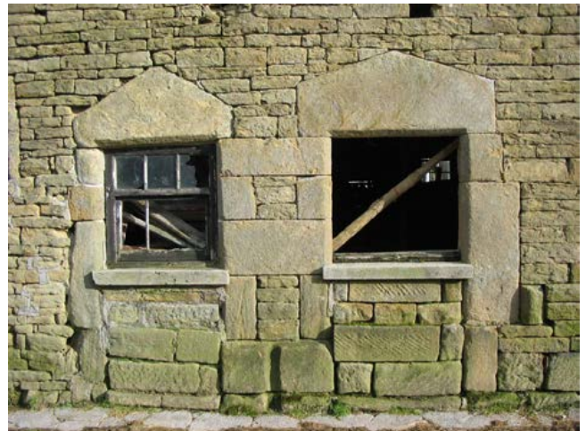
Highlow Hall barn near Hathersage. 17th-century combination barn with hayloft above cattle housing. The eaves line was originally lower, as there is evidence for raising to its present height. The front elevation is punctuated with entries, the shape of the massive lintels being a characteristic feature of 17th-century buildings in the area. Photos © Peak Park
