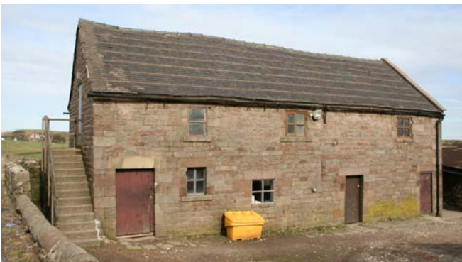
Larger outfarms were also built on the plateau, where large holdings developed in the late 18th and 19th centuries. This combination building faces into a yard and comprises a granary above a stable to the left, and a hay loft over cattle housing to the right. Photo © Bob Edwards
