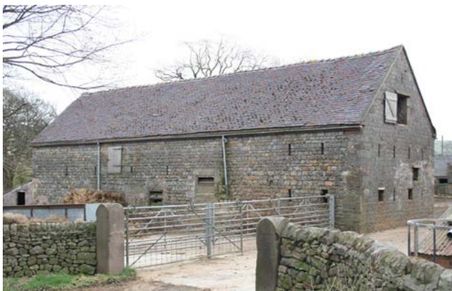
A large combination range, mainly cattle housing with a loft above, but with full-height crop storage in the end bay marked by the ventilation slits in the right gable end. Photo © Jen Deadman
