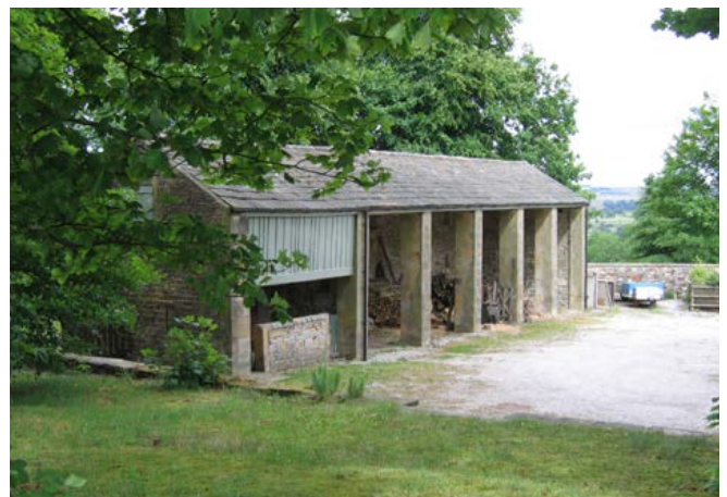
The importance of hay for winter fodder is shown in this large-scale hay barn with stone piers. Photo © Bob Edwards
