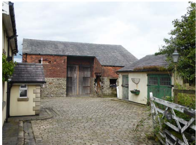
It is common, as here at Blackrod, to find evidence for the phased construction of buildings in dressed stone and later brick. The outshot, enabling the housing of more cattle than could fit into the span of the main building, is another common feature. Photo © Jeremy Lake
