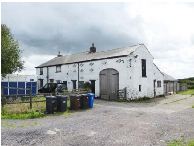
An early 19th-century, linear farmstead sited on the edge of newly-enclosed land, with ventilation holes marking the crop storage area, entries to a stable and cow house, a pitching door to the gable end and additional housing for cattle to the rear. Photo © Jeremy Lake
