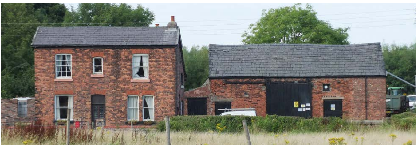
Here, also with a loose arrangement of small agricultural buildings to the rear, is a small, mid-19th-century steading with the house and combination barn separated by the yard entry. The combination barn is of standard plan form with central cart bay/threshing floor flanked by a lofted byre and full-height hay mew. Photo © Jen Deadman
