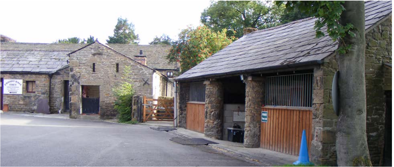
A three-bay cart shed of sandstone rubble with cylindrical stone columns with thin square caps supporting a graduated slate roof. Photo © Jen Deadman
