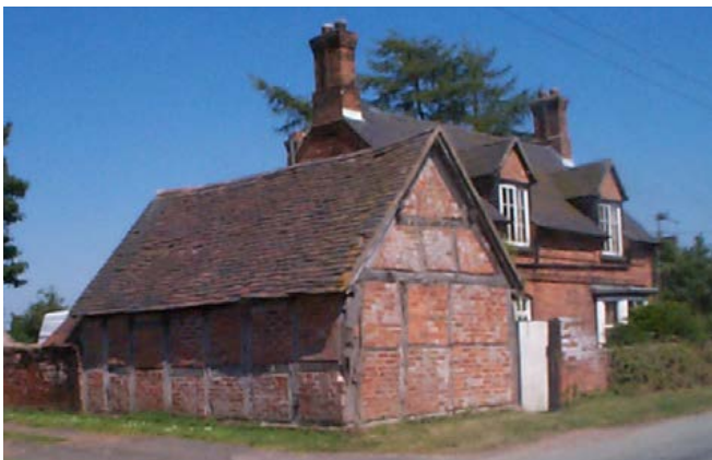
A small, timber-framed farm building, probably a cow house, on a small loose courtyard standing in north Shropshire. Photo © Shropshire County Council
