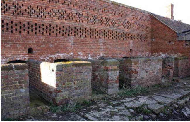
Pigsties were a common feature, especially on dairy farms. Here the pigsties are combined with a hen house above creating a 'poultiggery'. Photo © Bob Edwards
