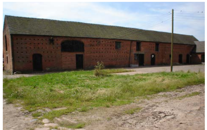
From the late 18th century, barns in the area – especially to the south – were usually incorporated into large brick-built, multifunctional ranges where, with mechanisation, the barn could be reduced to an upper floor room with no large threshing doors. Photo © Shropshire County Council
