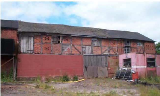
Rebuilding with L-shaped multifunctional ranges was so extensive that few earlier buildings for the housing of cattle have survived. These are very rare, and form part of a distribution of timber-framed cow houses along the Welsh borders. The only other areas in England with early timber-framed cattle housing are in the former dairying areas in the claylands of East Anglia and the stock rearing and fattening areas of the Weald in south-east England. Some examples also survive in the Lancashire Plain.
