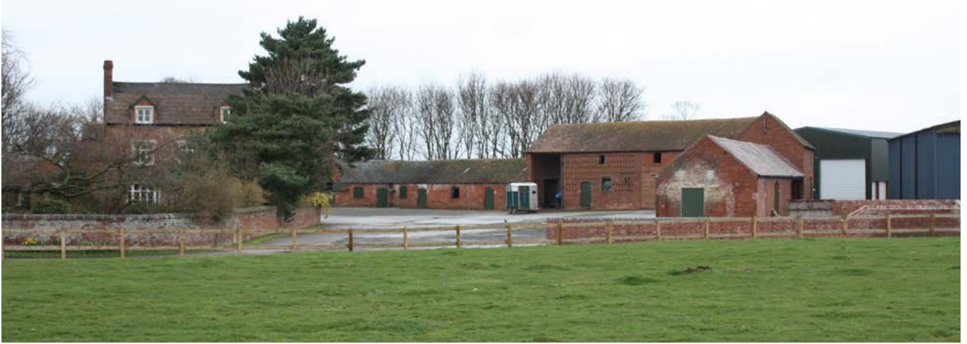
A regular U-plan range with a combination barn and extensive stabling and outward facing cart shed bays, which reflects the importance of arable farming in the southern sub-area. Photo © Bob Edwards
