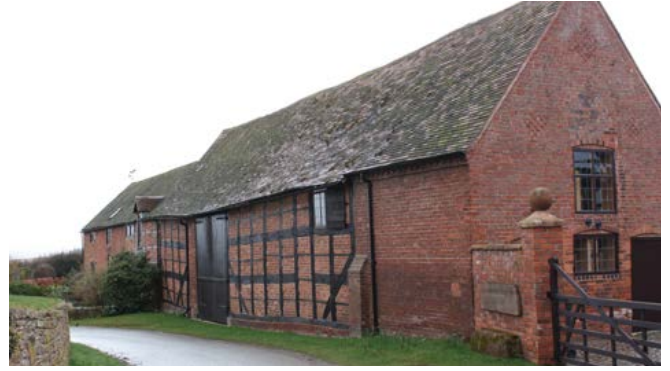
A timber-framed threshing barn near Shrewsbury. This is five bays in length, but many barns in this area and around the Severn are larger. It displays the square panel-framing, typical of the western English carpentry tradition. This barn was extended with brick stable and granary ranges in the 19th century. Photo © Bob Edwards
