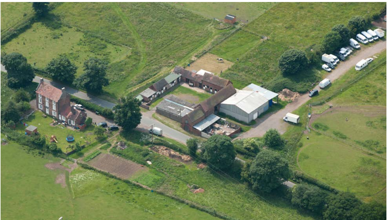
A regular courtyard 'U' plan constructed of brick and typical of the larger farmsteads to be found in the mixed farming areas to the south of the area (this one is in Staffordshire). The working buildings had originally stood adjacent to the late 18th-century, three-storey farmhouse, but were rebuilt on a new site on the opposite side of the road in the mid-19th century. The new arrangement appears to be a reflection of the social aspirations of the occupier, with the farmhouse sited with its back to its working buildings. Photo © Historic England 27701/003
